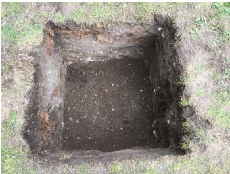
Protective soil added prior to pouring concrete
