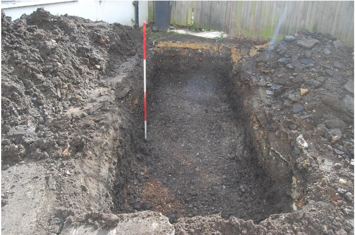
Plate 4. Trench 2, looking south from the north
