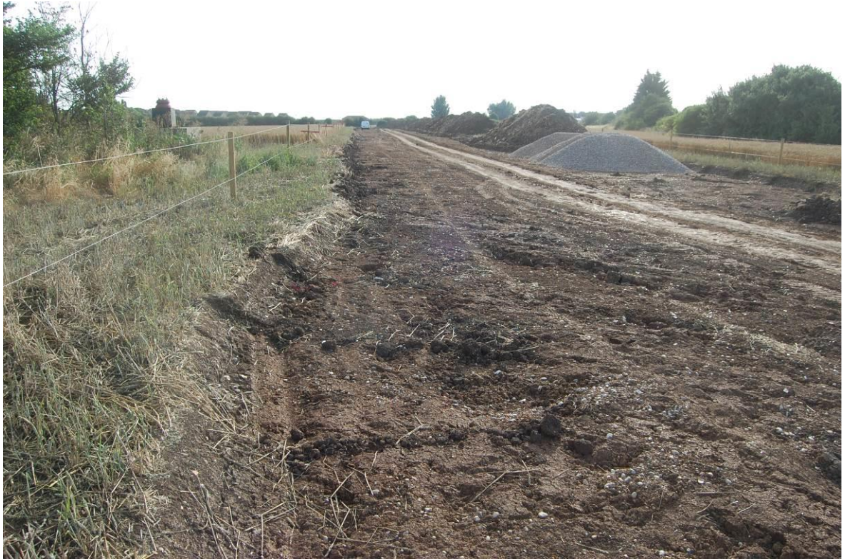
Plate 15. View of the north-east to south-west section of the Warden Bay scheme, from its south-western end, after machine reduction to the exposed upper surface of the London Clay. No scale.
