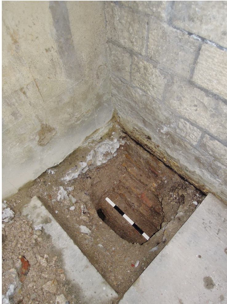
Fig. 11 Test Pit 5 in courtyard. Stepped brick footing to north-west wall 504, looking west. Scale, 50cm
