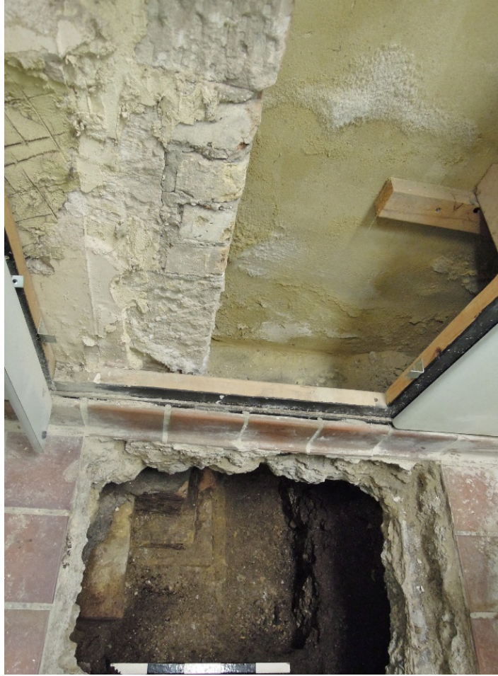
Fig. 9 Test Pit 1 in Gents toilet. Stepped brick footing exposed, looking south-east. Scale, 50cm
