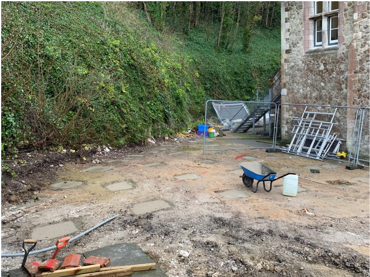
Fig. 5 Excavated pits on north-eastern side of the site filled with concrete
