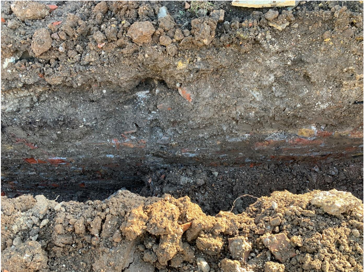
Fig. 11 Detail view of brick wall 438 exposed in face of SE Trench, looking south-east
