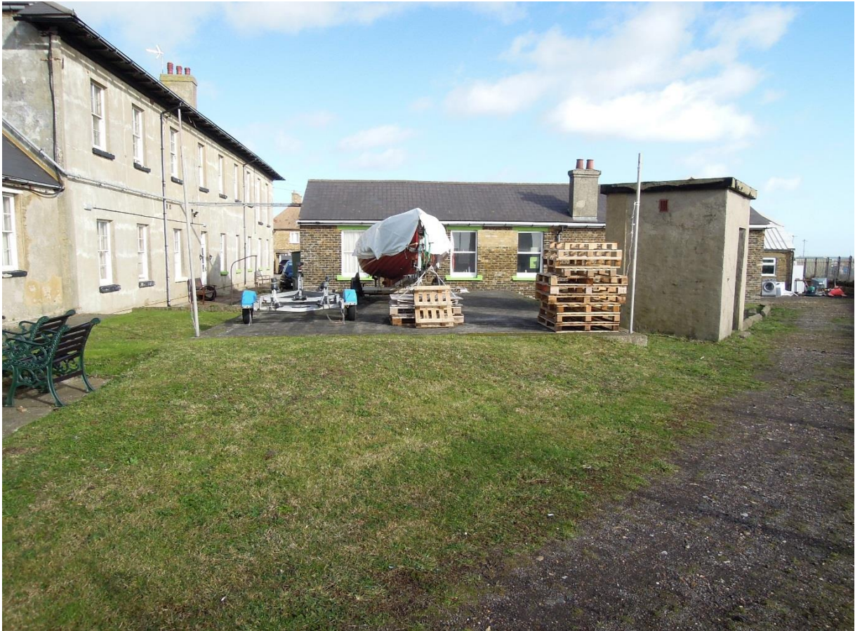
Fig. 7 General view of Building 9 (platform) looking north-east in 2019
