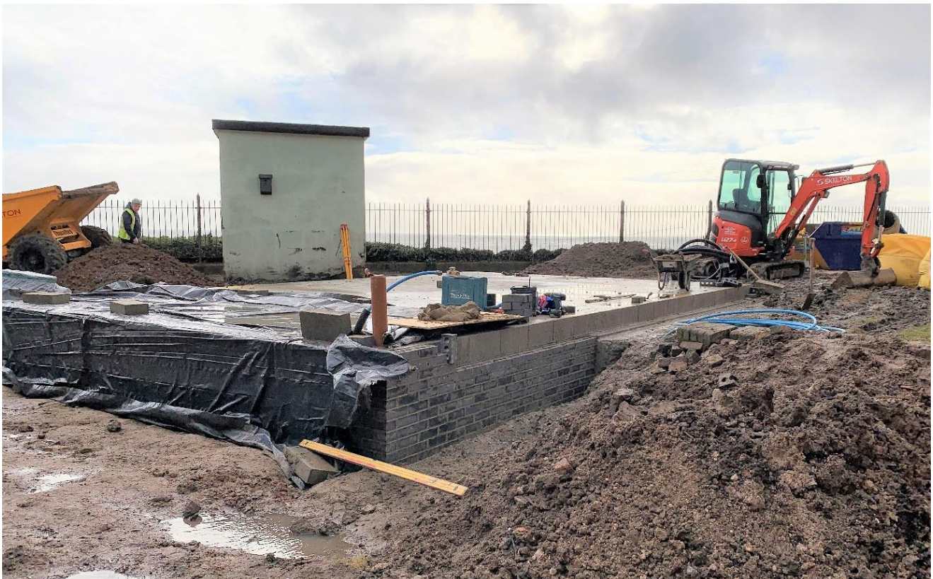
Fig. 18 The completed foundation for the new workshop, looking south
