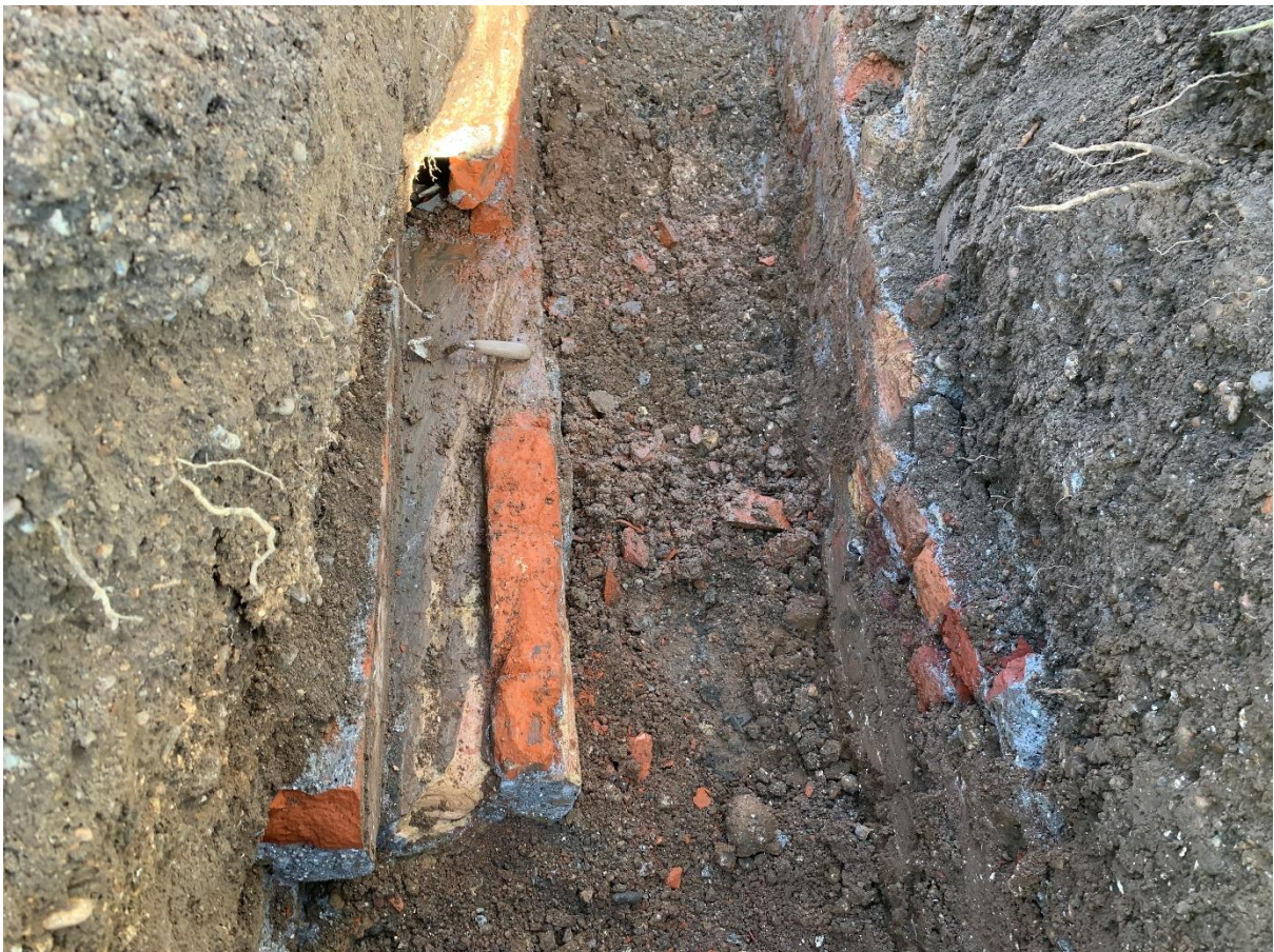
Fig. 14 Brick culvert 406 and Wall 438 exposed in SE Trench, looking north-east
