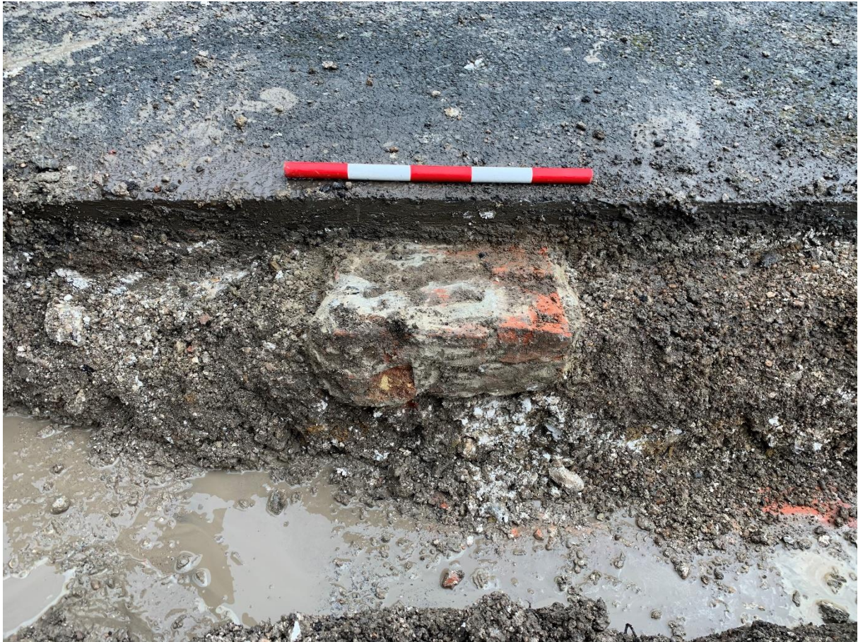
Fig. 14 Small brick pier, Context F. 22, located south of Spur Casemates, looking east. Scale, 50cm
