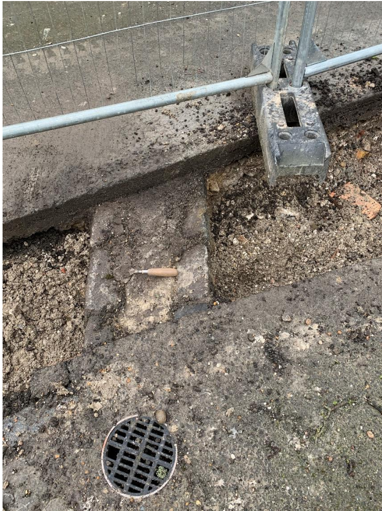
Fig. 12 Cobbled drainage gully, Context F. 23, exposed to the east of stable block, looking east
