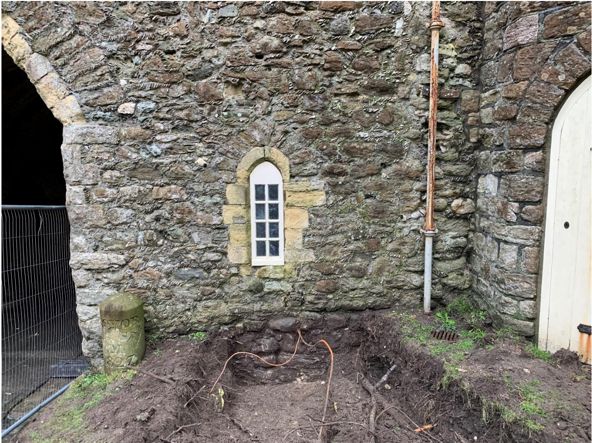
Fig. 6 General view of trenching on eastern side of Constable's Gate-tower, looking west
