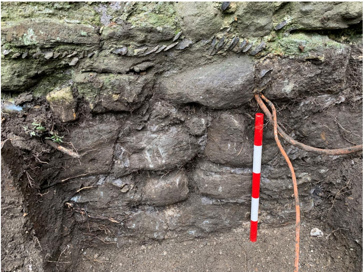
Fig. 7 Detail of construction of east wall of Constable's Gate-tower below ground. Scale, 50cm
