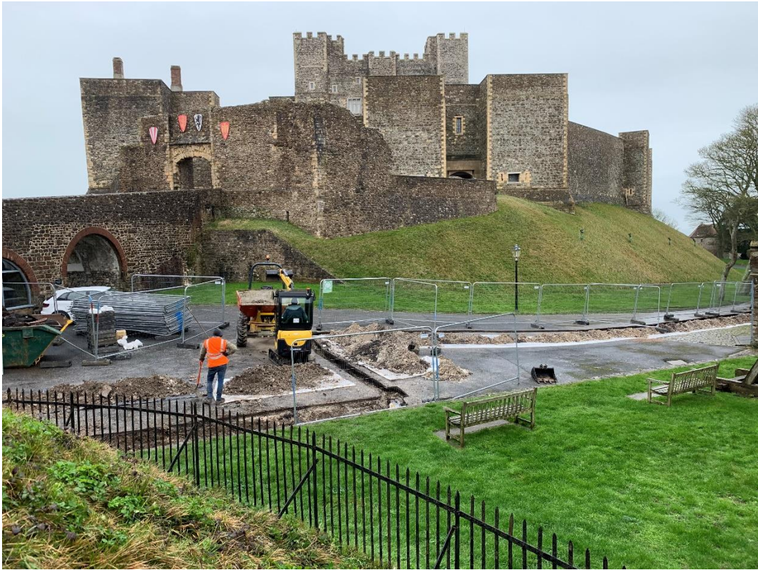
Fig. 4 Trenching work in the area of Test Pits 1 and 2, looking south-east
