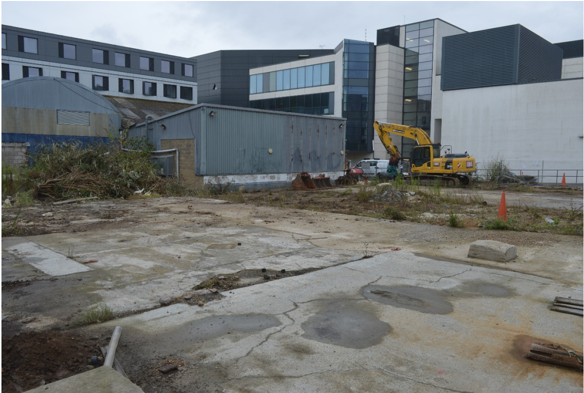
Image 2. General view of PDA prior to archaeological investigation works, looking northeast
