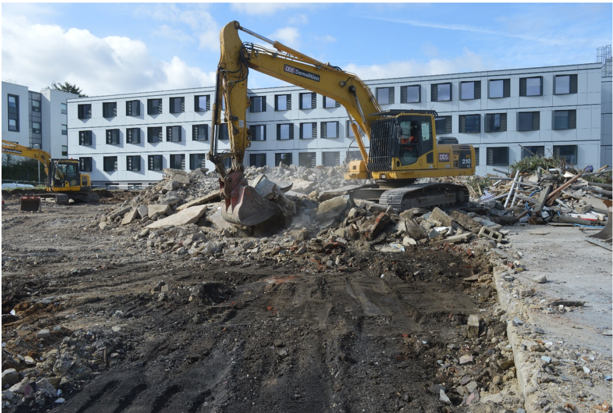
Image 3. Monitoring of demolition groundworks in progress, looking northeast
