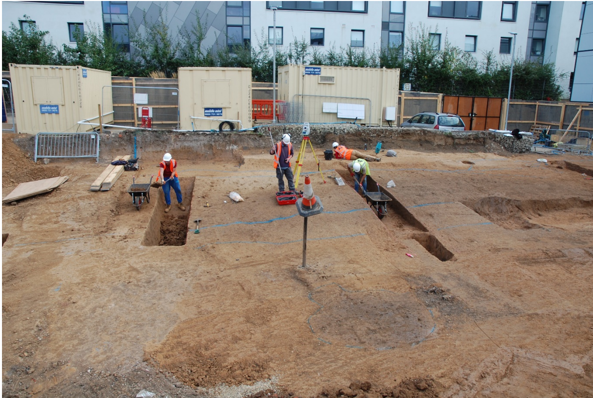
Image 14. G6 cemetery boundary ditch during hand excavation, looking southeast
