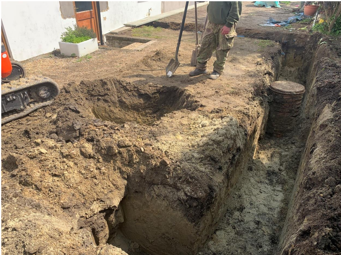
Fig. 12 General view of completed trenches, looking south
