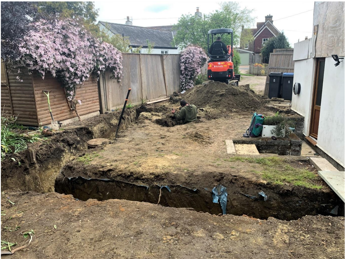
Fig. 10 General view of the site, looking north
