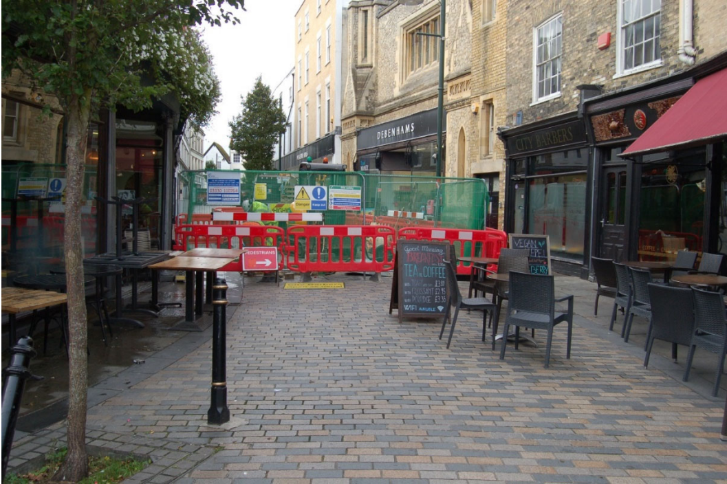
Photo 17. Site 9 Guildhall Street, trench location, looking south-west (no scale)
