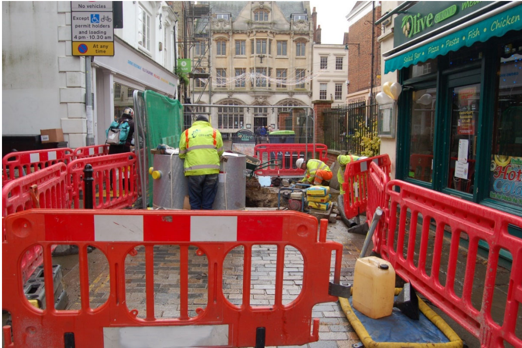
Photo 11. Site 6 Best Lane, trench location, looking south-west (no scale)
