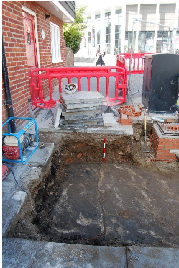
Photo 9. Site 5 The Friars, trench location, looking west (scale 0.5m)
