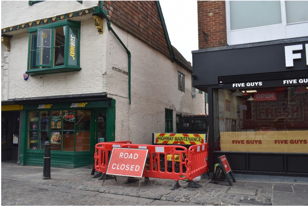
Photo 7. Site 4 St Peter's Grove, trench location, looking south-west (no scale)
