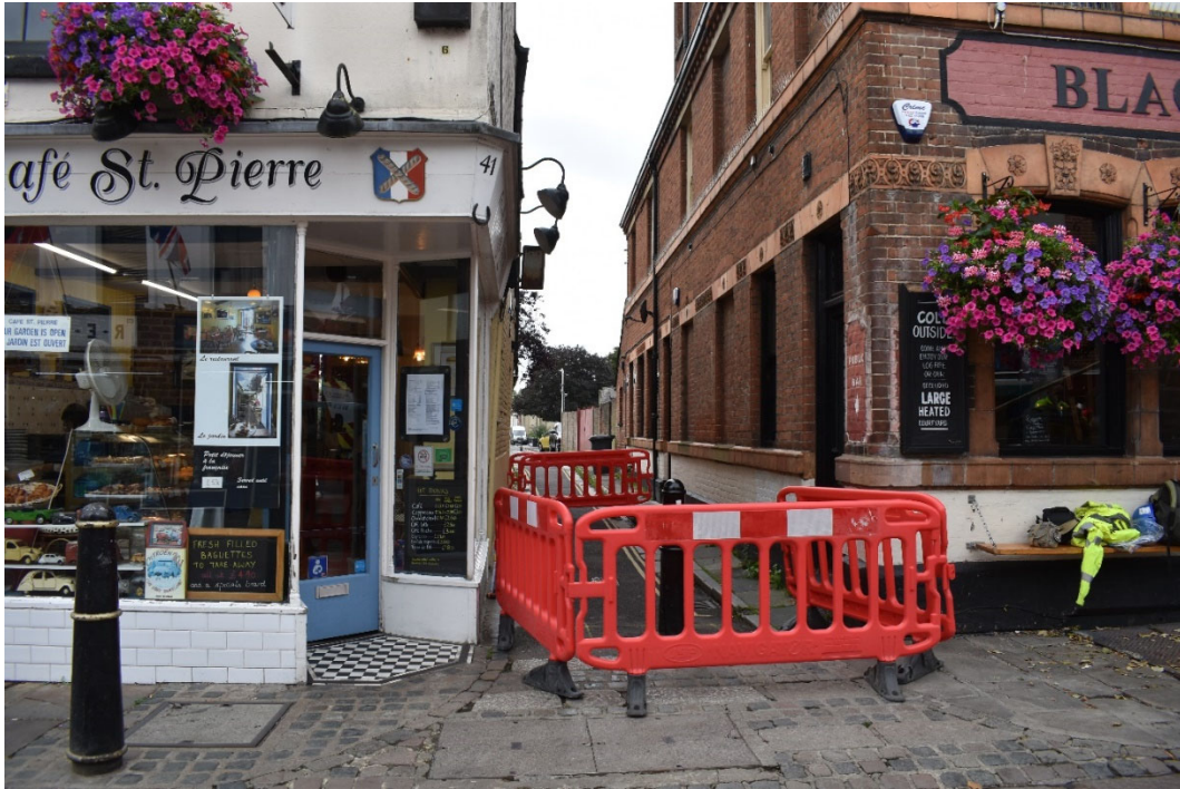
Photo 3. Site 2 Black Griffin Lane, trench location, looking south-west (no scale)
