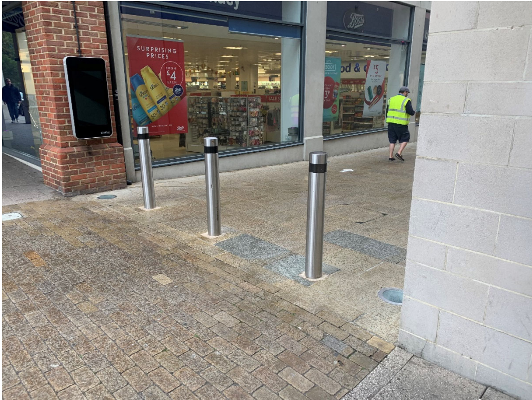
Photo 35. Site 16 Gravel Walk (footway), trench location post-installation, looking north-west (no scale)
