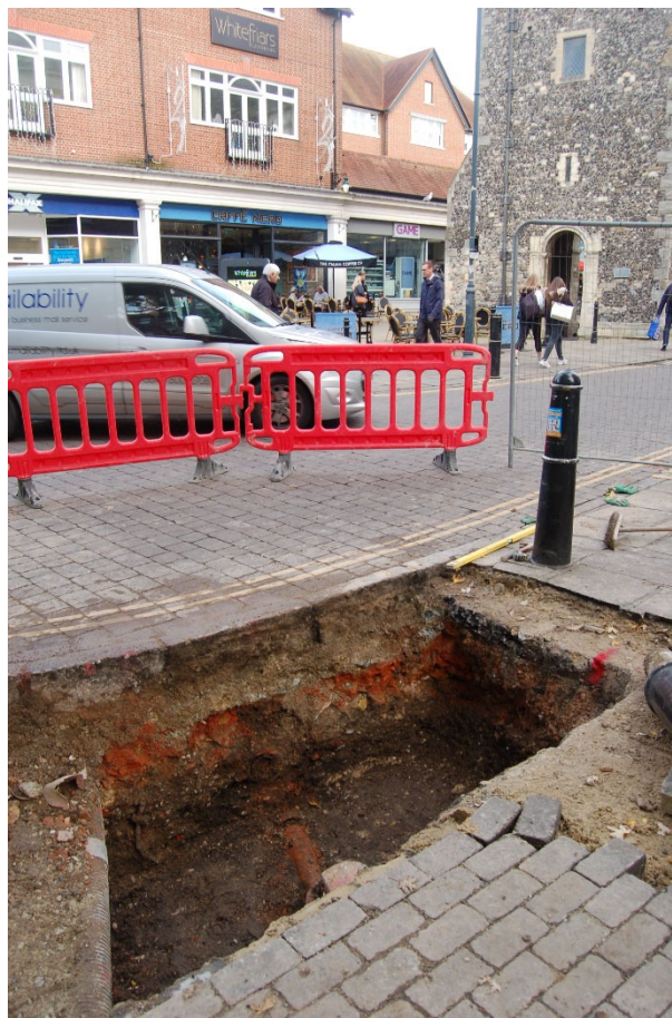
Photo 24. Site 12 St George's Street, trench A location, looking east (no scale)
