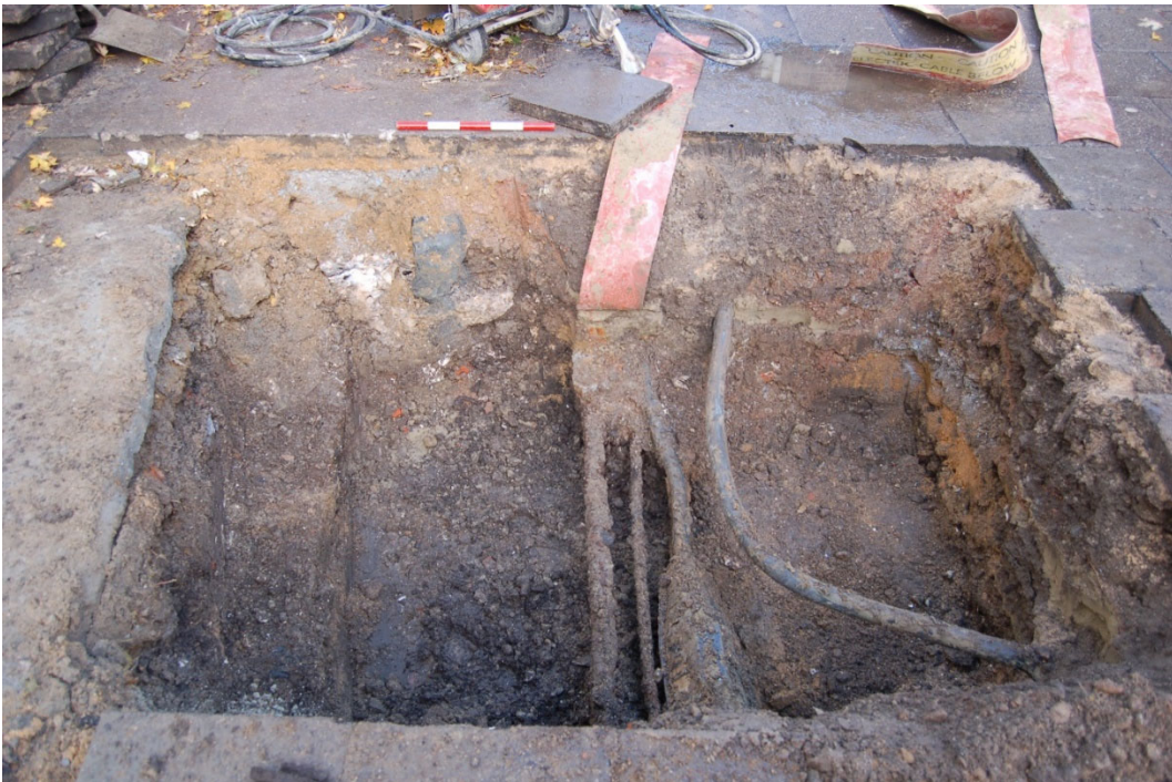
Photo 26. Site 12 St George's Street, trench B, looking north-west (scale 0.5m)
