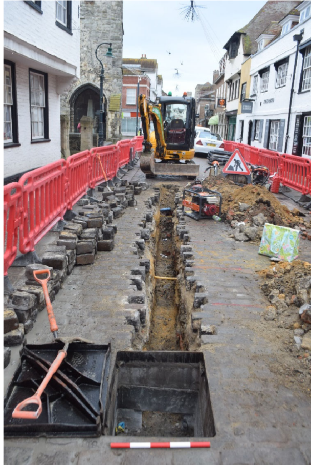
Photo 27. Site 13 Burgate, trench location, looking north-west (scale 0.5m)
