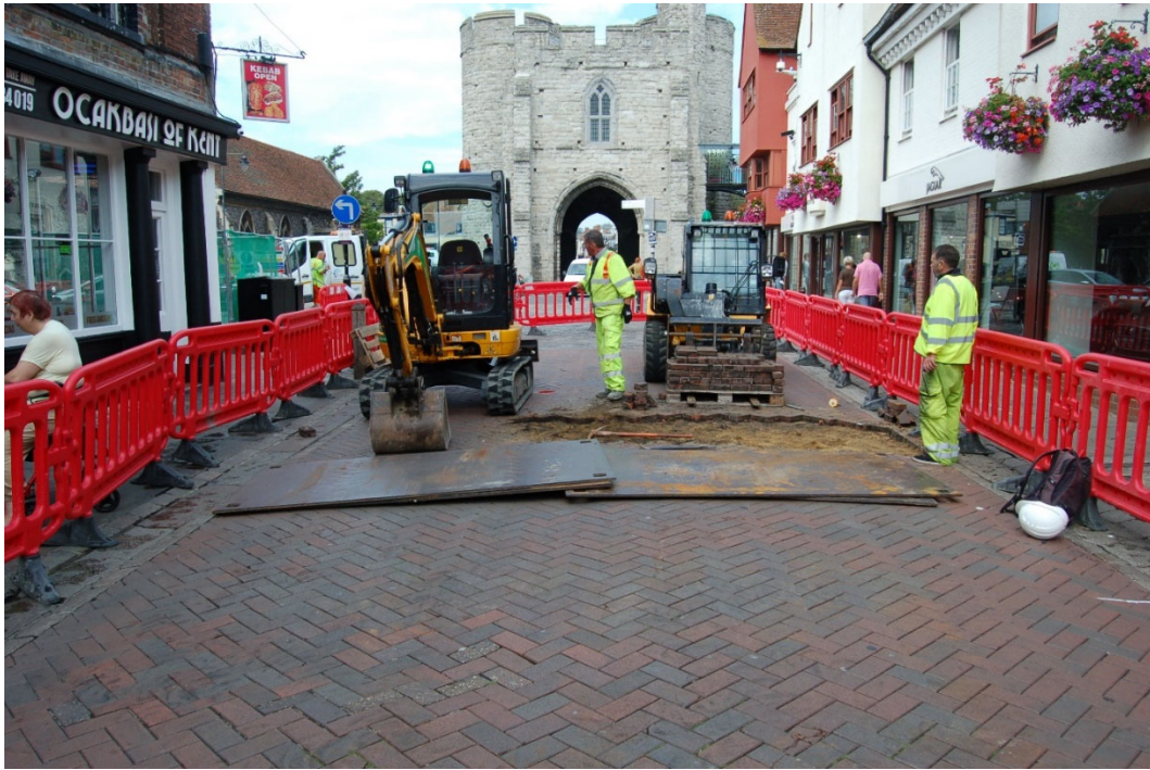
Photo 1. Site 1 St Peter's Street, trench location, looking north-west (no scale)
