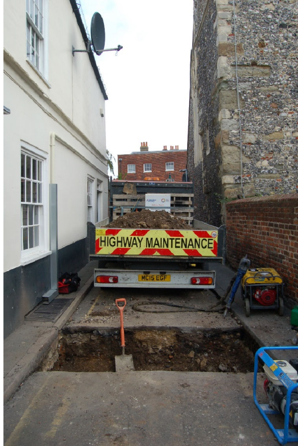
Photo 5. Site 3 St Peter's Lane, trench location, looking north-east (no scale)
