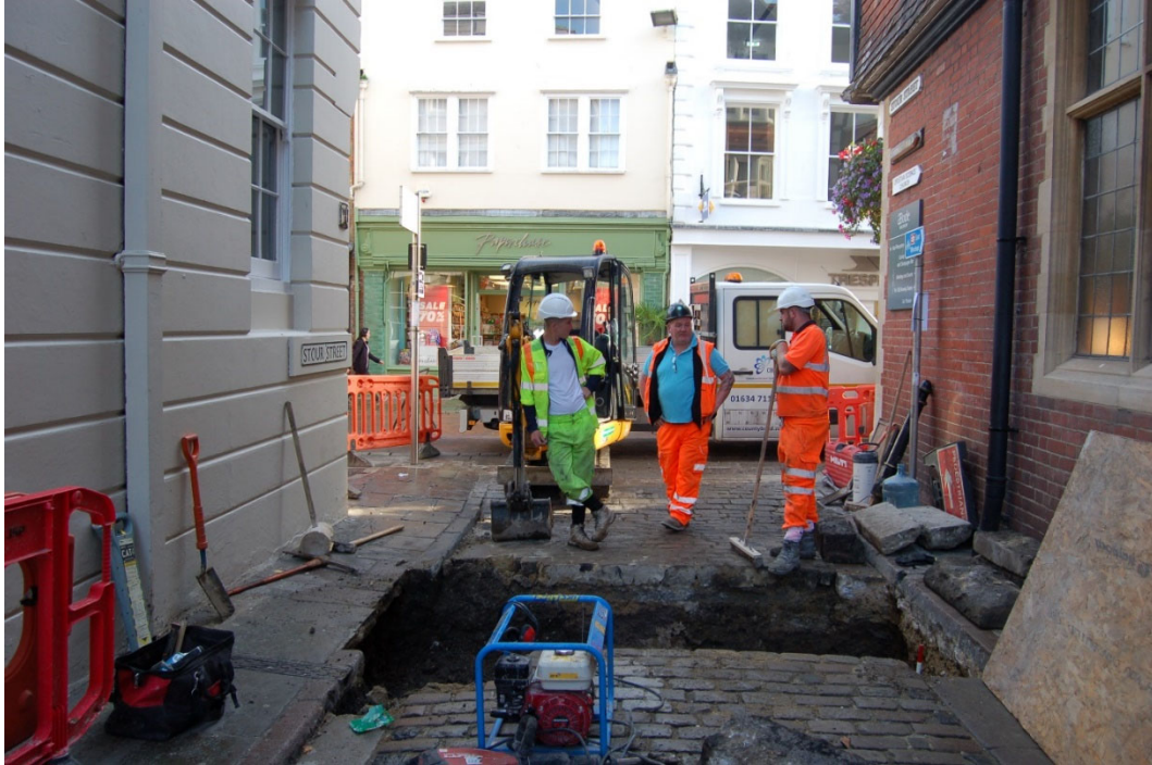
Photo 13. Site 7 Stour Street, trench location, looking north-east (no scale)
