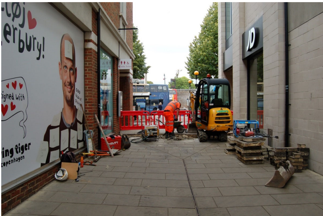
Photo 36. Site 17 Whitefriars Passage, trench location, looking south-east (no scale)
