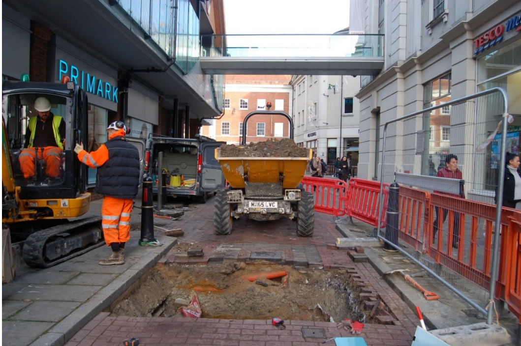
Photo 29. Site 14 Rose Lane, trench location, looking north-east (no scale)
