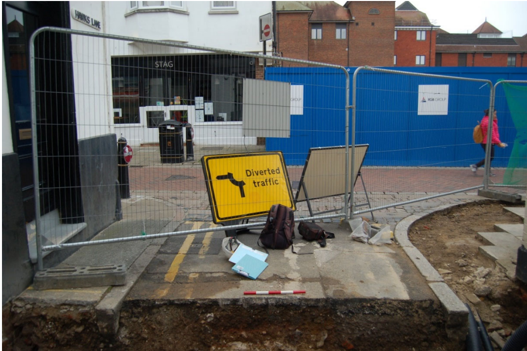
Photo 37. Site 18 Hawks Lane, trench location, looking south-east (no scale)
