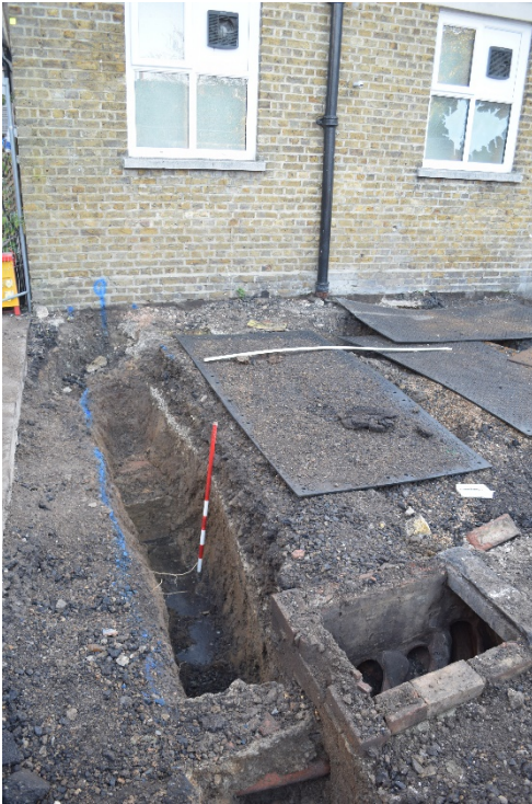
Plate 1. Extension footings, looking south-west scale 1m
