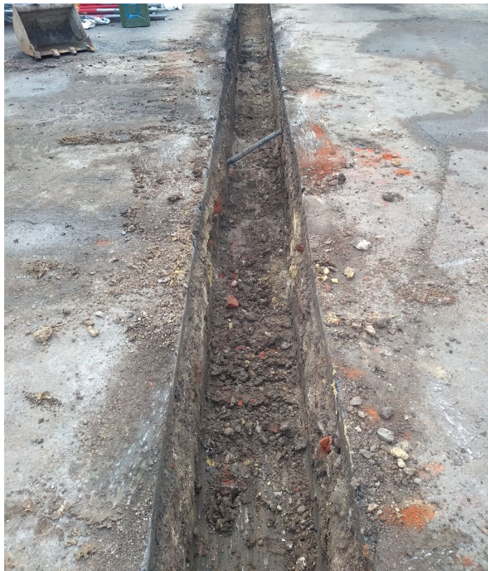
Photo 14. Longport Car Park, Area 3 duct trench, looking north (no scale)
