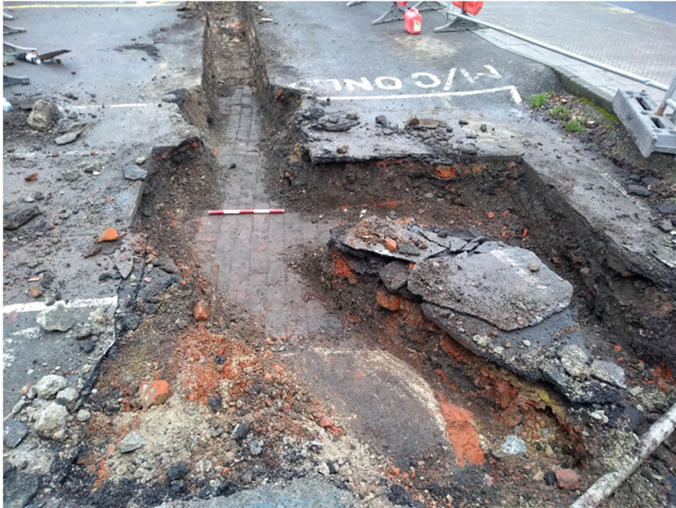
Photo 25. Watling Street Car Park, brick walls 5004 and 5020, brick floor 5005, concrete floor 5023, and utility trench 5022, looking north-west (scale 0.5m)
