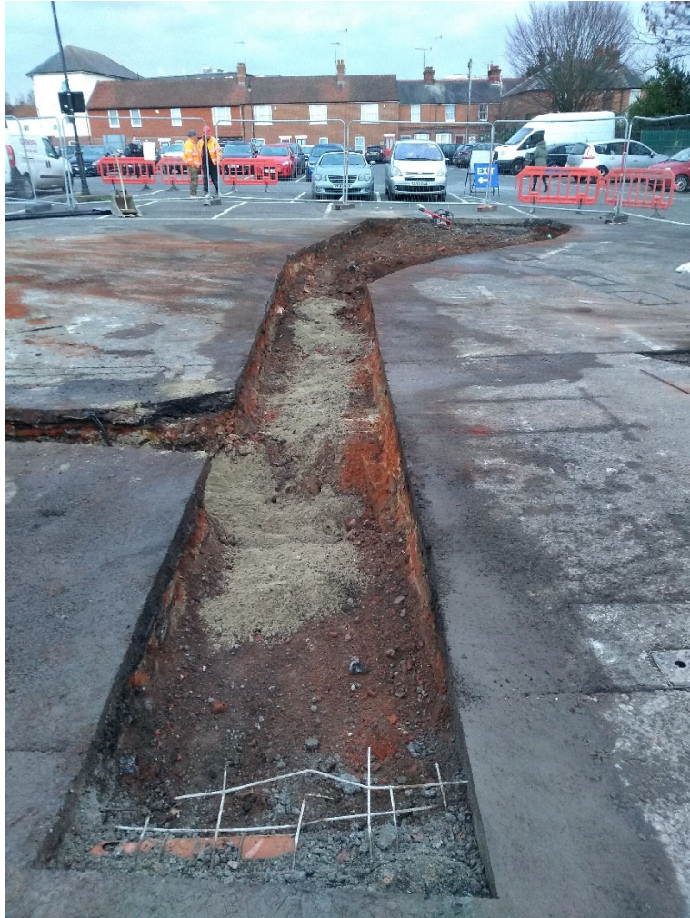
Photo 15. Longport Car Park, Area 4 barrier island, looking south (no scale)
