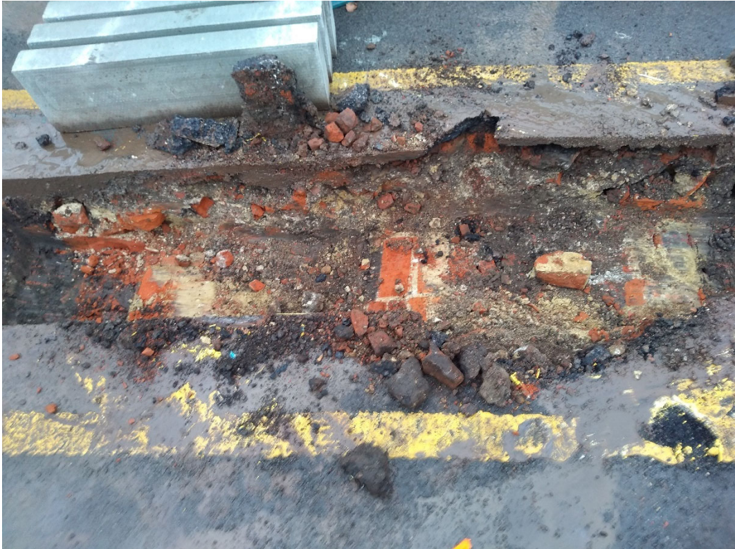
Photo 27. Watling Street Car Park, brick walls 5016, 5017, 5018 and 5019, looking south-west (no scale)
