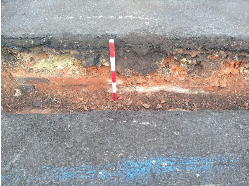
Photo 31. Queningate Car Park, brick wall 6010, looking south-east (scale 0.5m)
