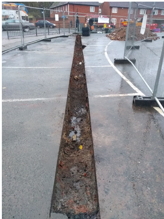
Photo 12. Longport Car Park, Area 1 duct trench, looking south-east (no scale)
