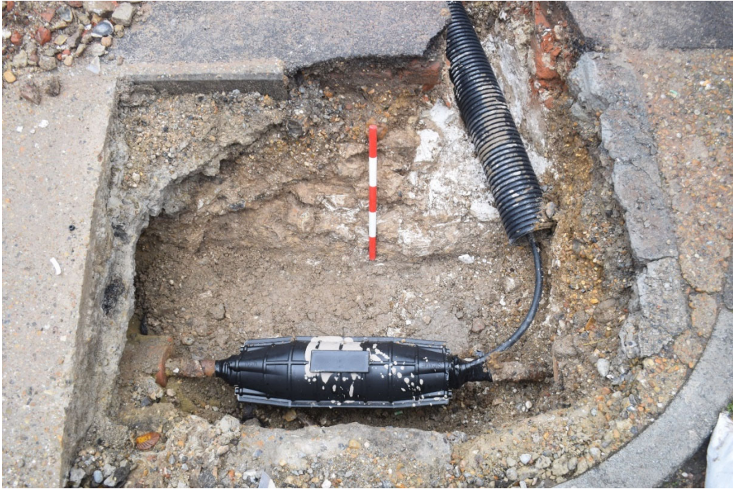
Photo 1. St Radigund's Car Park, masonry wall 1404, looking north (scale 0.5m)
