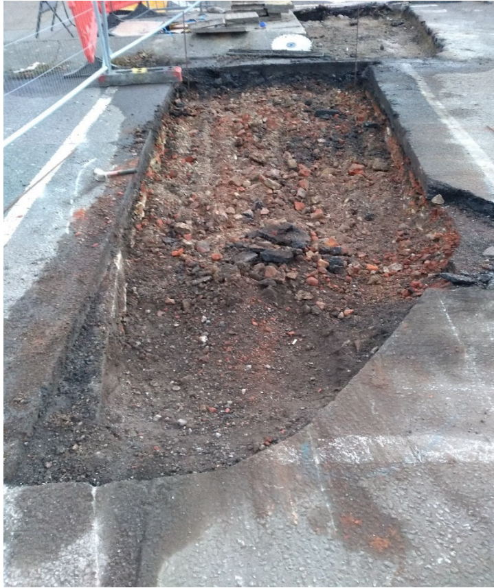
Photo 17. Longport Car Park, Area 4 brick wall 3019, looking north (no scale)
