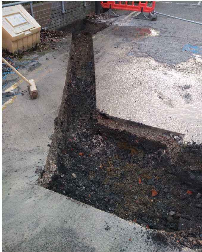
Photo 20. Castele Row Car Park, Area 1, duct trench, looking south-east (no scale)
