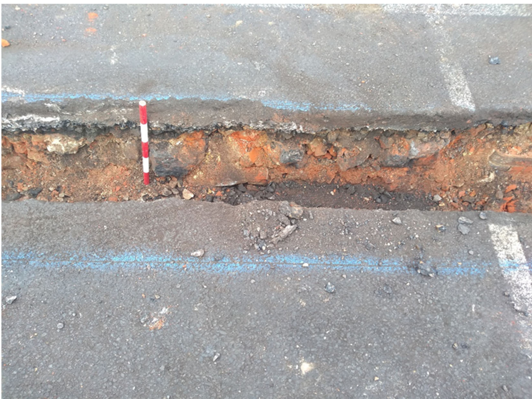
Photo 32. Queningate Car Park, duct trench, demolition deposit 6005, looking west (scale 0.5m).
