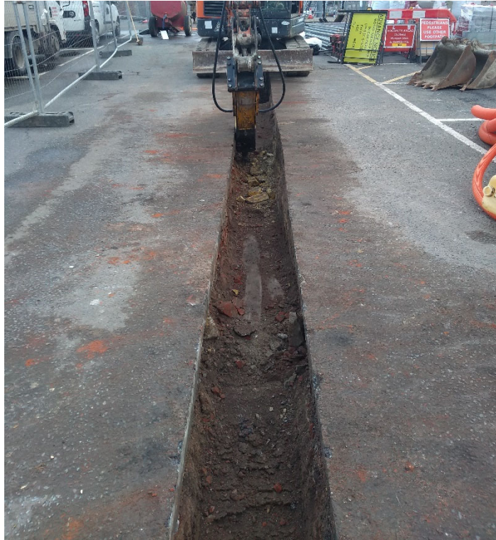
Photo 13. Longport Car Park, Area 2 duct trench, looking north-west (no scale)
