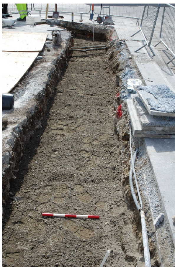
Photo 2. Marlowe Theatre Area 1 bollard installation trench, looking south (scale 0.5m)
