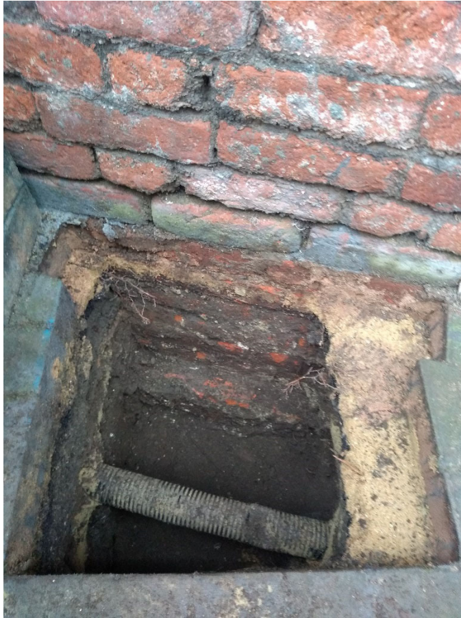
Photo 6. Marlowe Theatre Area 2 security gate installation trench P1, looking north-west (no scale)
