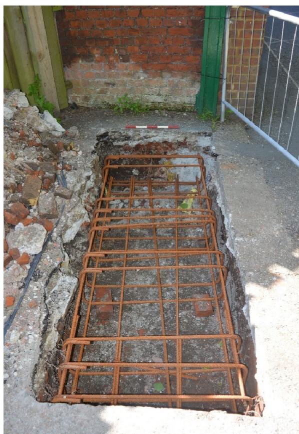
Photo 11. Marlowe Theatre Area 3 bollard installation trench, looking north-west (scale 0.5m)
