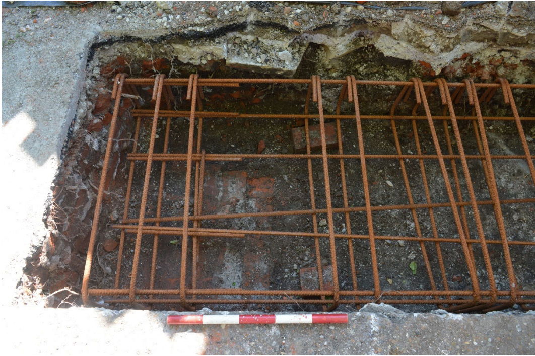
Photo 12. Marlowe Theatre Area 3 bollard installation trench, brick floor 3004, looking south-west (scale 0.5m)
