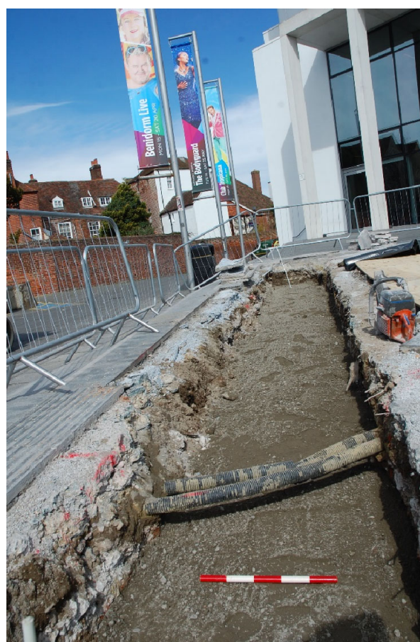
Photo 3. Marlowe Theatre Area 1 bollard installation trench, looking north (scale 0.5m)
