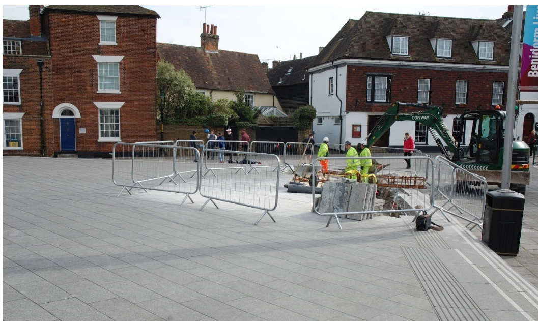
Photo 1. Marlowe Theatre Area 1, bollard installation trench location, looking south (no scale)
