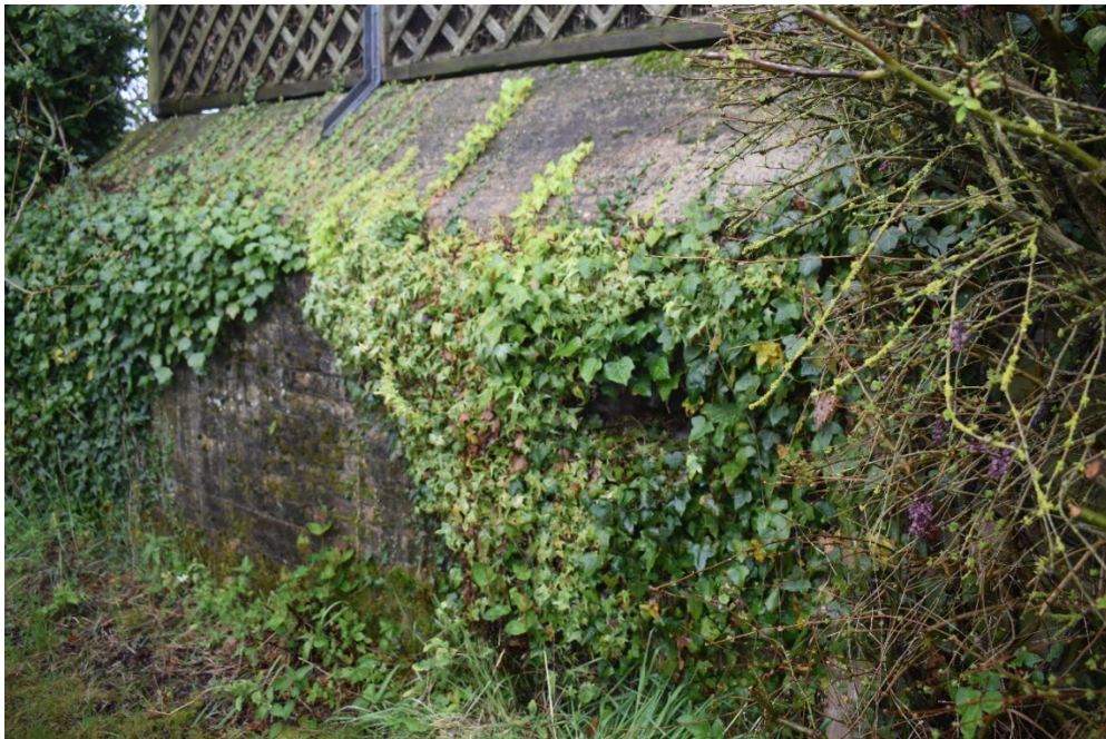
Plate 12. View of Second World War shelter, incorporated into the property of Abbots Court Lodge, located at the north-western boundary of Area 1
