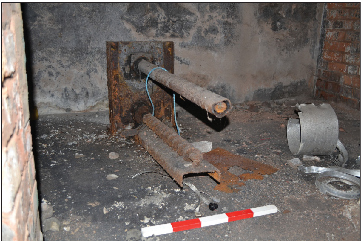
Plate 14: Photo no. 161 Original coal feeder to boiler, Infirmary boiler house, looking north-east
