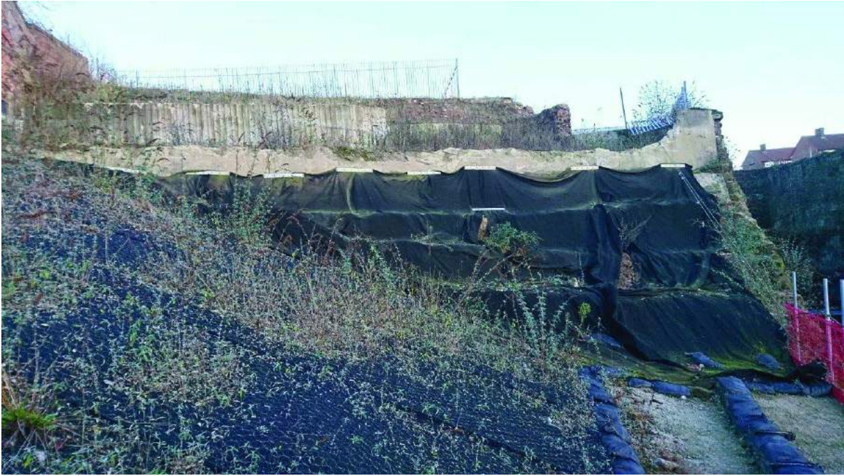
Plate1: Concrete structure obscuring the eastern extent of the 'Triple Decker Tunnel'
