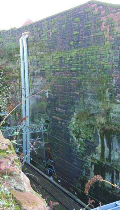
Plate 2: The stopped-up continuation of the 'Triple Decker Tunnel'
