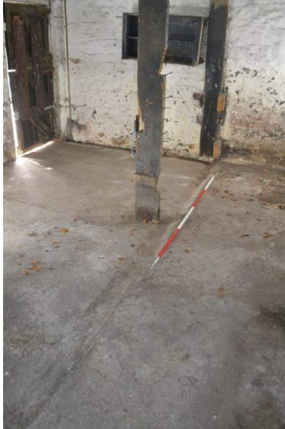
Plate 48: Stable ground floor, detail of channel cut into concrete floor.
