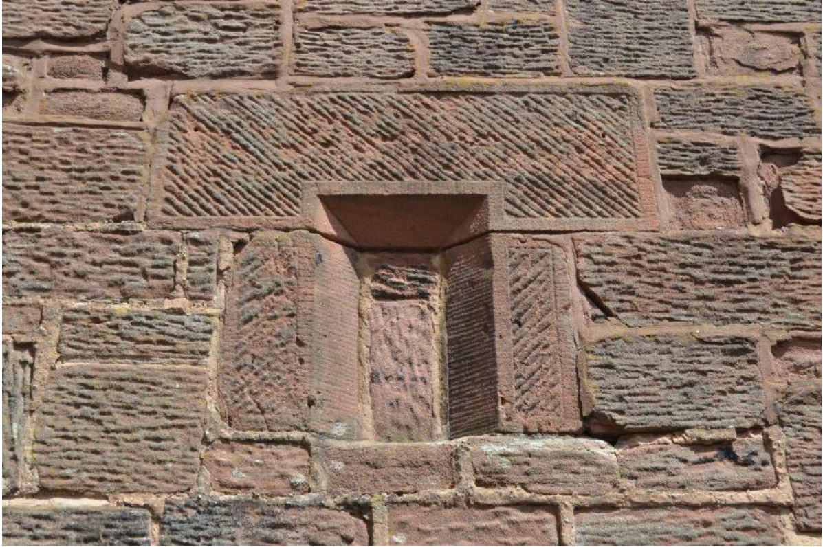
Plate 15: Detail of curtailed and blocked arrow-slit vent.
