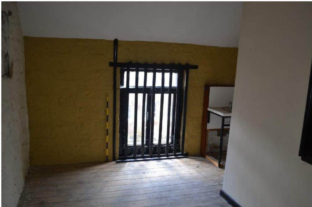
Plate 81: First floor, Workshop, view towards the window opening in the south-facing elevation with casement frame and security bars. Scale = 1m
