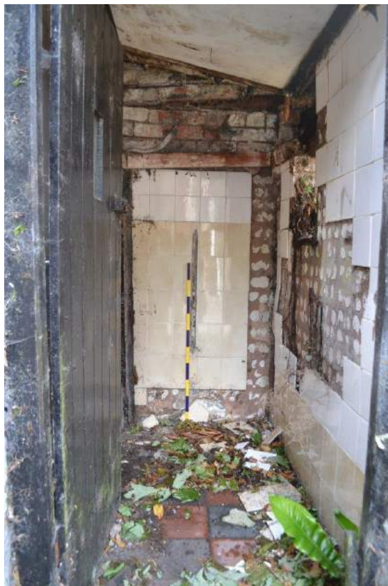
Plate 111: Interior of the WC. Scale = 1m
