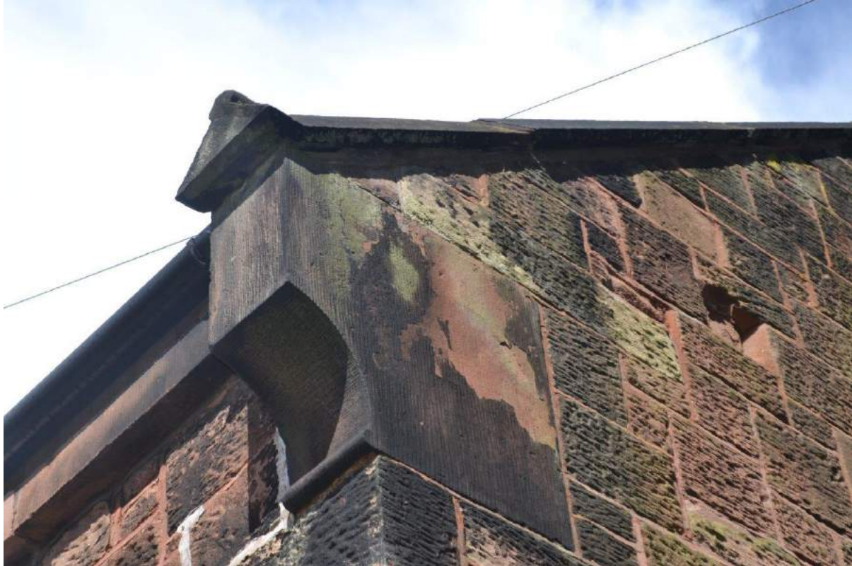
Plate 63: Detail of the finely dressed projecting corbelled gable skew with cavetto moulding and roll margin. Also roll-topped, pyramidal coping terminal and fascia
