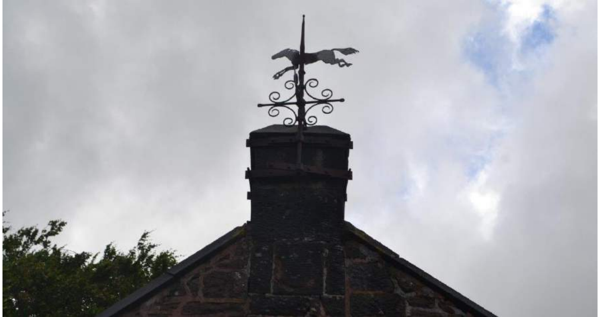
Plate 65: Detail of decorative, equine themed weathervane affixed to chimney by iron straps.
