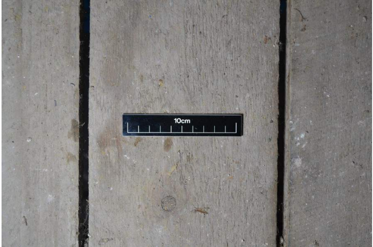
Plate 32: Floorboards on the northern balcony, probably deal-boards. Floorboard is 175mm wide (7 inches). Scale = 10cm.
