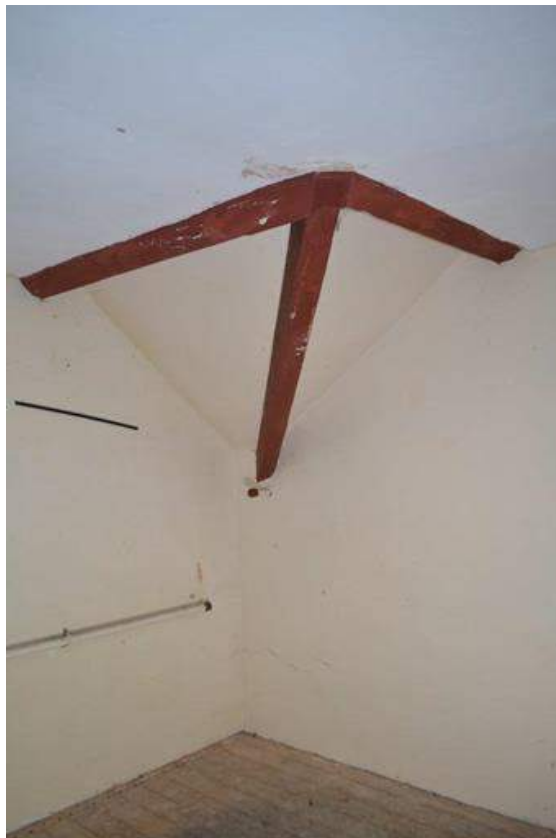
Plate 53: Stable first floor, detail of valley rafter and jack rafters
