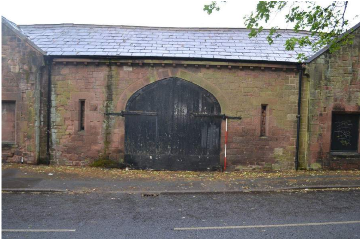
Plate 7: Sightline to the east from Quarry Street to the east-facing, random-coursed elevation of the barn showing the cart-entrance door, the multi-centred arch and broached ashlar facings, also the two arrow slit vents with broached ashlar facings.
