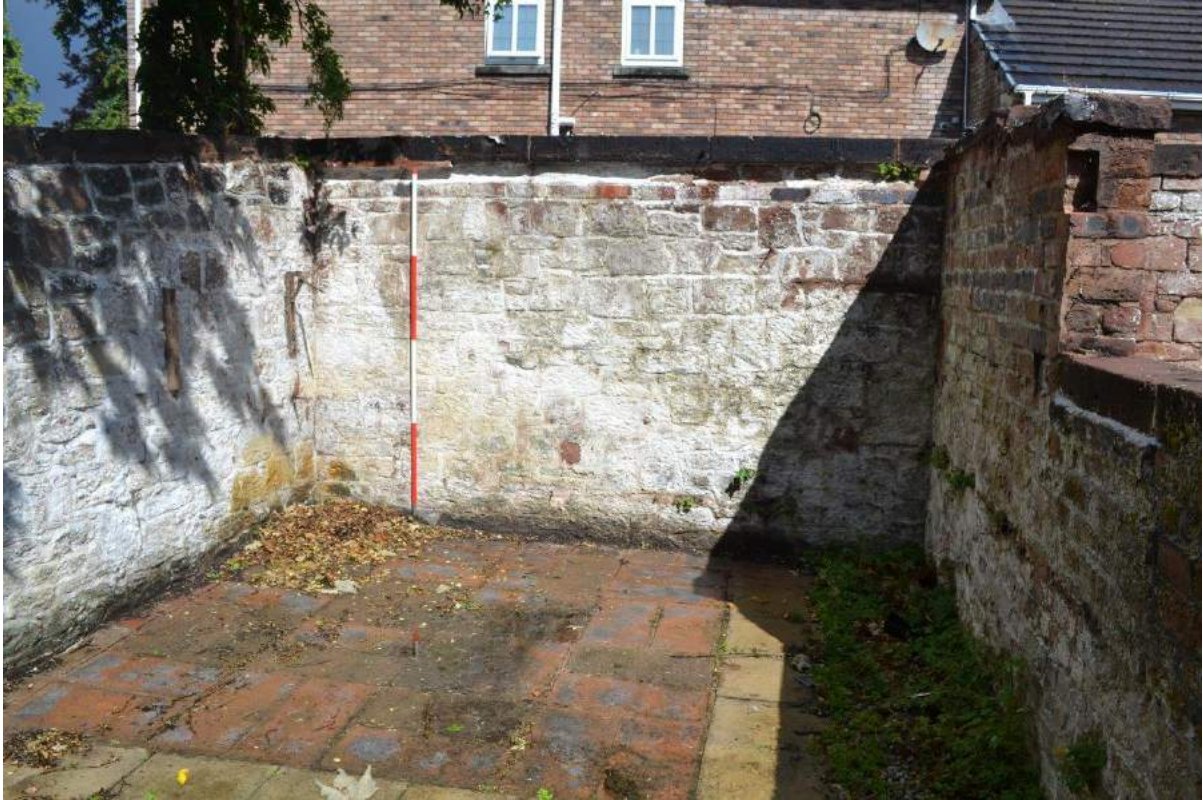
Plate 101: Sightline into the western bay of the pigsty showing the interior of the first and second loose boxes, white-washed side of the north-facing elevation and the wall dividing the second stall from the third.
