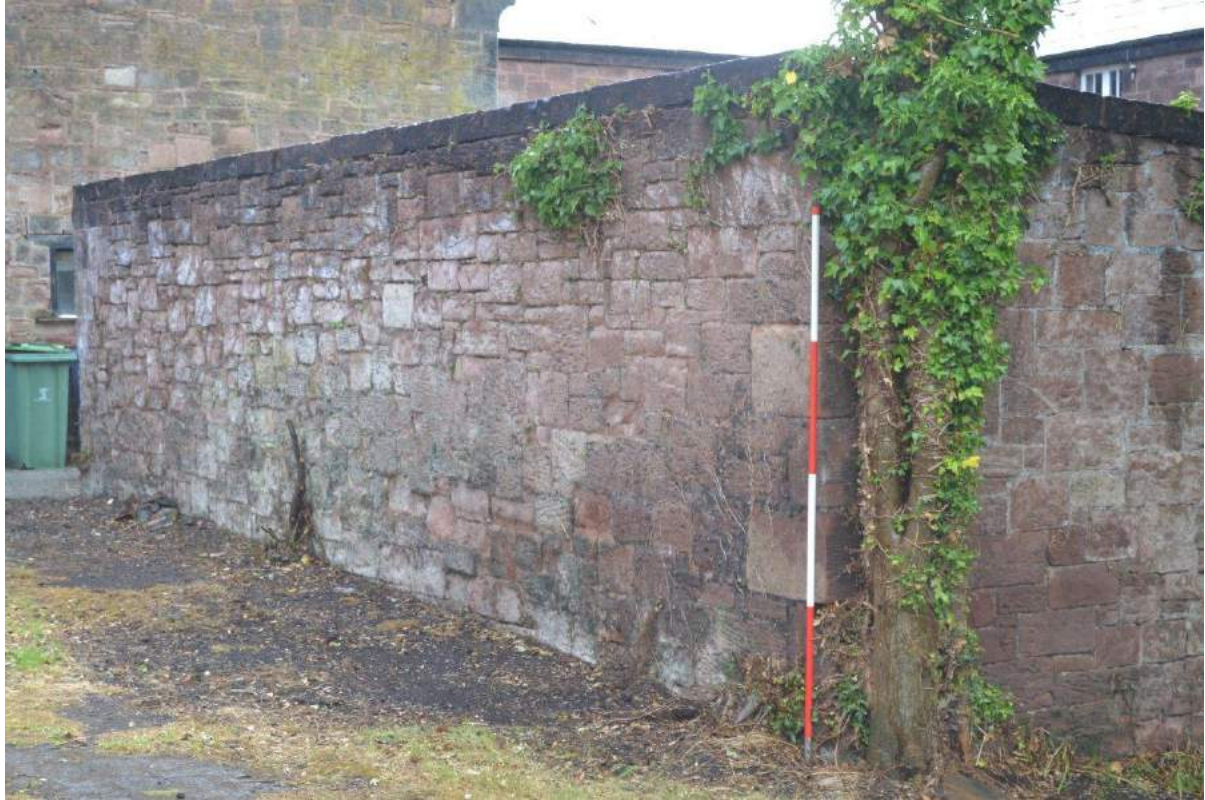
Plate 93: Sightline looking south-east towards the north-facing elevation of the pigsty
