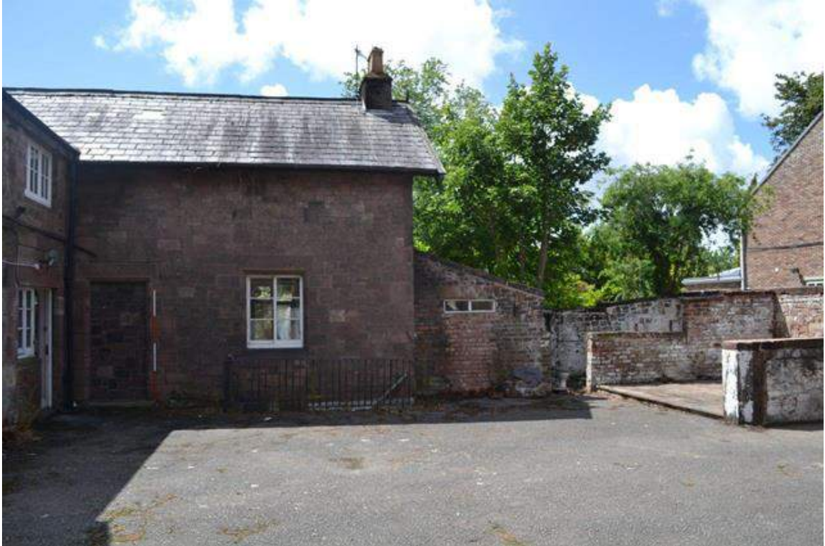
Plate 104: Sightline to the east from the farmyard showing the brick-built west-facing elevation single storey store, with twin-light window and mono-pitch roof, butted onto the north-facing gable end of the western wing of the farmhouse
