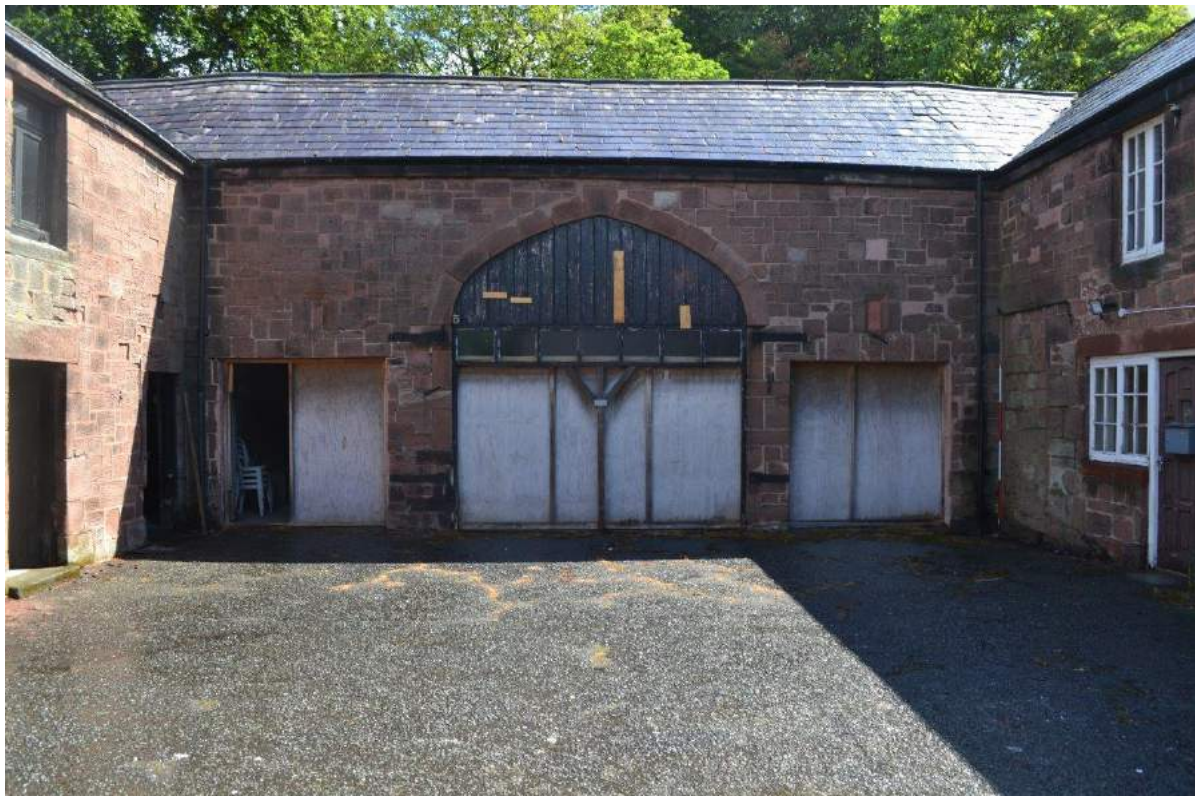
Plate 10: Sightline to the east from the farmyard showing the west-facing, random-coursed elevation of the barn with the cart-entrance blocked up and two doorways inserted either side of it, curtailing the arrow slit vents.
