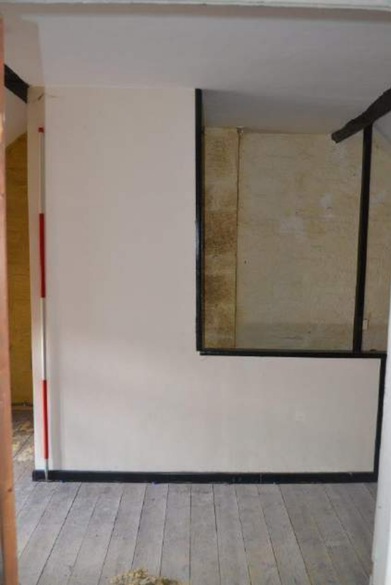
Plate 85: First floor, Workshop, partitions defining the staircase
