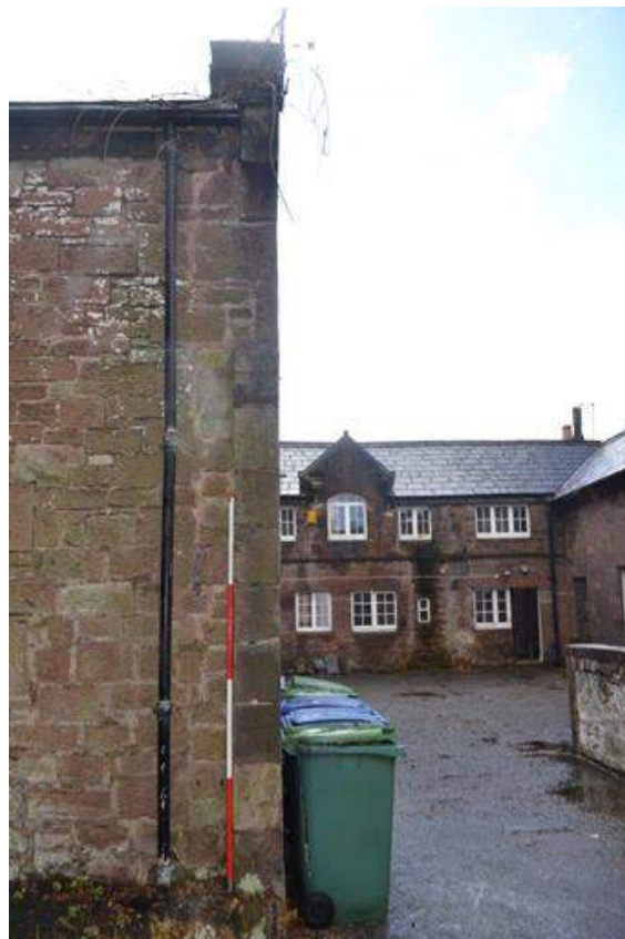
Plate 60: Sightline to the south showing the broached ashlar quoining (farmhouse in background).
