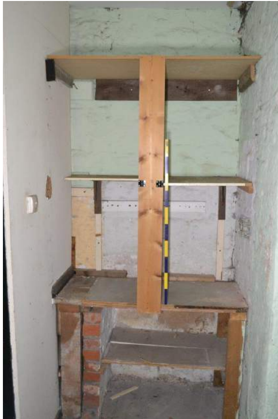
Plate 72: Ground floor, Workshop, view of the shelving. Scale = 1m
