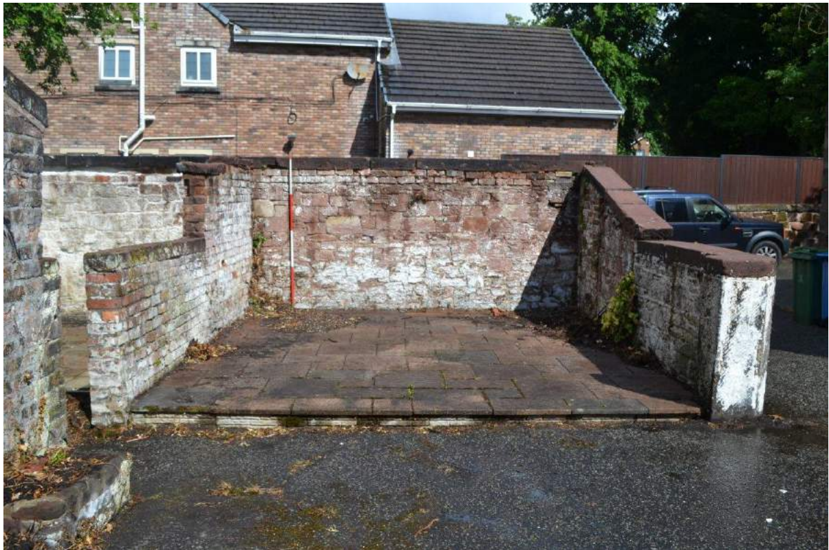
Plate 100: Sightline to the north, into the western bay of the pigsty from the farmyard. The wall forming the exercise yard, which probably contained the feed chutes, the wall to separate the loose box from the exercise yard and the third and fourth stalls are all no longer extant.
