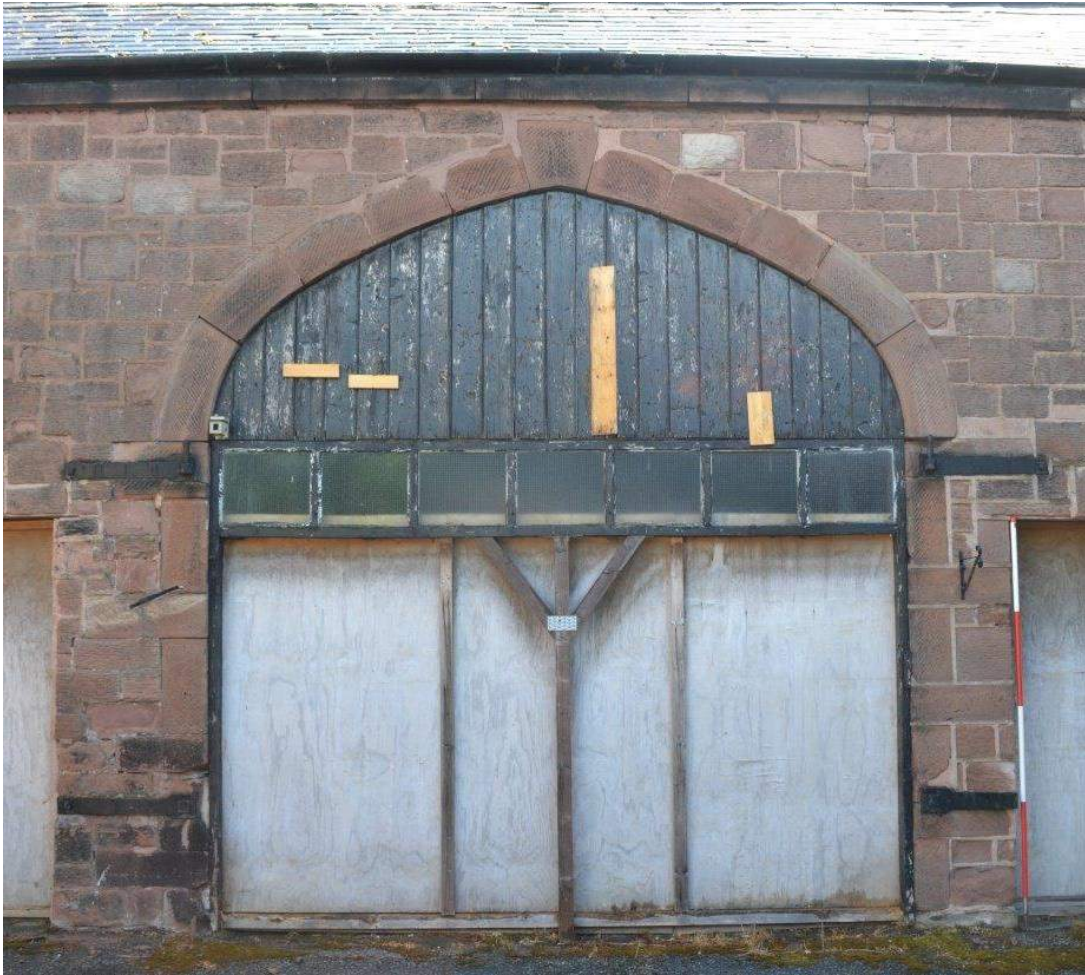
Plate 11: Detail of the blocked-up cart-entrance with multi-centred arch. Note secondary, lower set of carcass hinge leaves, and exposed pintles of the upper set of carcass leaves.
