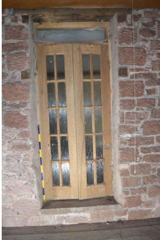
Plate 26: The opening containing a porte-fenêtre above a stone sill and under a timber lintel (scale = 1m)
