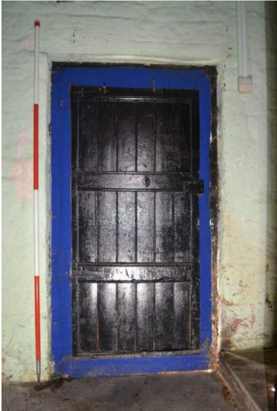
Plate 71: Ground floor, Workshop, view of the internal side of the ledged and framed timber door onto the farmyard
