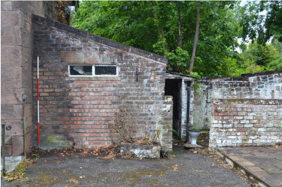
Plate 109: Sightline to the west showing detail of the east-facing brick-built elevation of the Store, with twin-light window, over-sized stone lintel and concrete sill in what appears to be a blocked doorway. Note stone verge coping.
