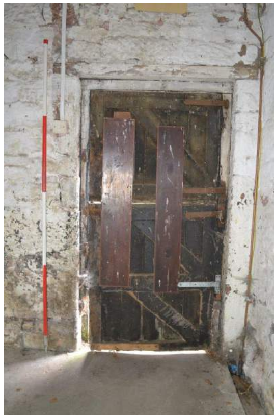
Plate 49: Stable ground floor, detail of the timber stable door, panelled, braced, framed and ledged
