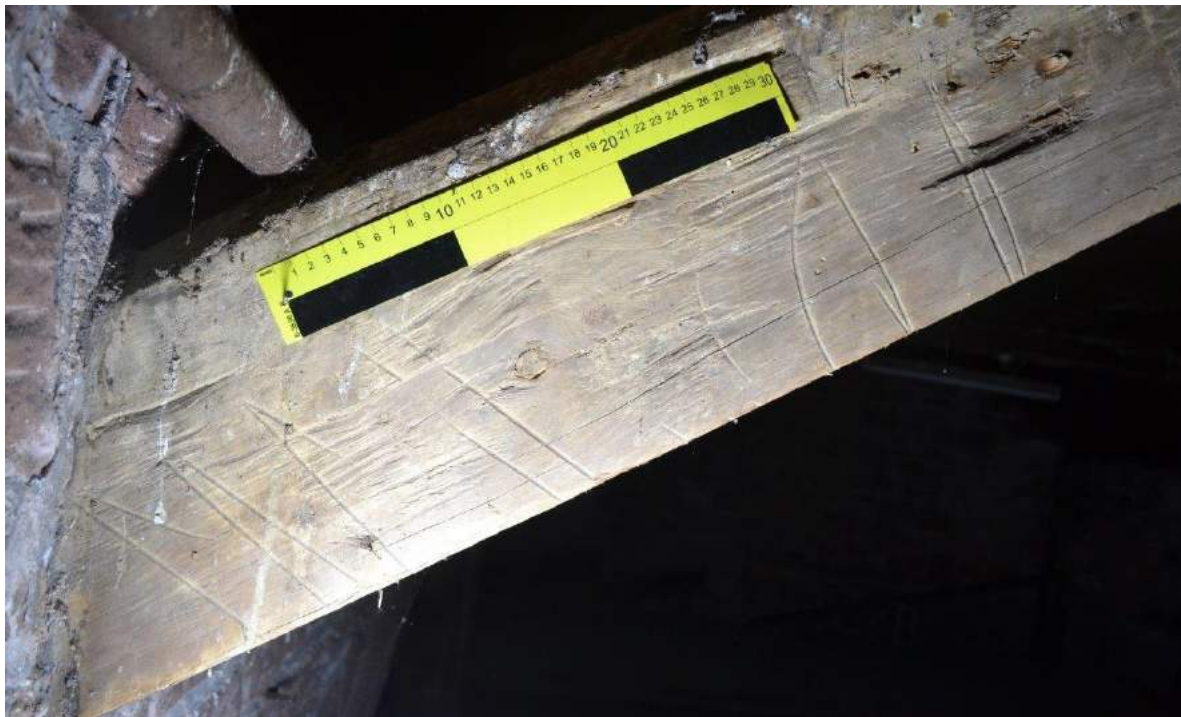
Plate 31: Carpenter's marks (apotropaic marks – potential Marian symbol or demon trap? 5 ) on the principal rafter. Scale = 30cm.
