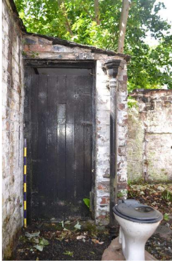
Plate 110: Looking west to the doorway entrance to the WC, with mono-pitch roof, plain close verge and cast-iron rainwater goods (hopper and down-pipe). The construction of the WC, in a passage between the pigsty and the Store effectively rendered the first two stalls of the pigsty unusable. Scale = 1m
