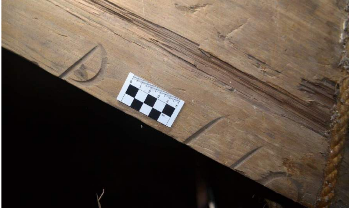
Plate 30: Possible carpenter's marks made with a race knife on the principal rafter. Such marks are usually Roman numerals, but corresponding geometric shapes are not unheard of. Scale = 5cm.
