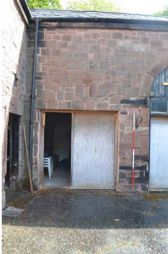
Plate 13: Detail of the inserted doorway to the left of the cart-entrance
