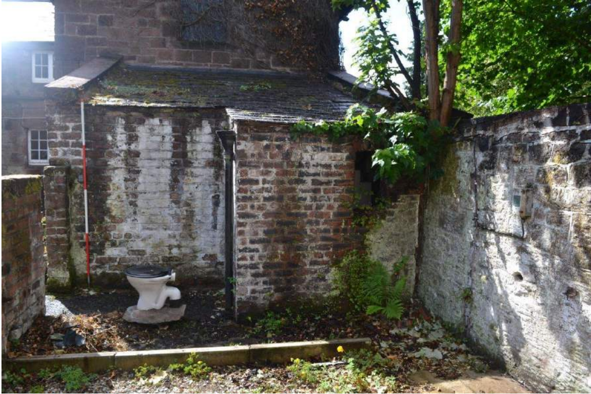
Plate 106: Sightline to the south from the western bay of the pigsty towards the brick-built, north-facing elevations of the WC and the Store showing the mono-pitch roofs.
