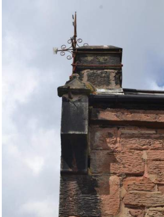
Plate 67: Sightline to the north to the south-facing elevation of the workshop showing detail of the finely dressed projecting corbelled gable skew with roll-topped, pyramidal coping terminal and fascia.
