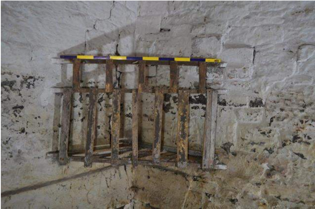
Plate 43: Stable ground floor, hay rack in corner formed by east-facing gable elevation and north-facing flank wall. Scale = 1m
