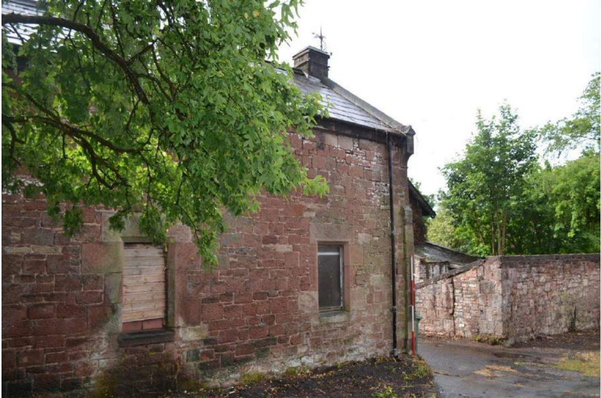
Plate 57: Sightline to the south-west showing an oblique view of the north-facing elevation of the workshop, highlighting ground floor window, weathervane, capped chimney-in-gable-wall, dressed fascia, coping-at-gable and projecting corbelled gable skew
