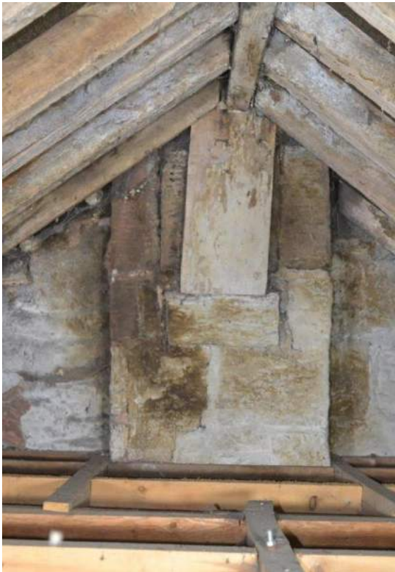
Plate 87: Roof space, Workshop, detail of chimney breast in west-facing gable elevation
