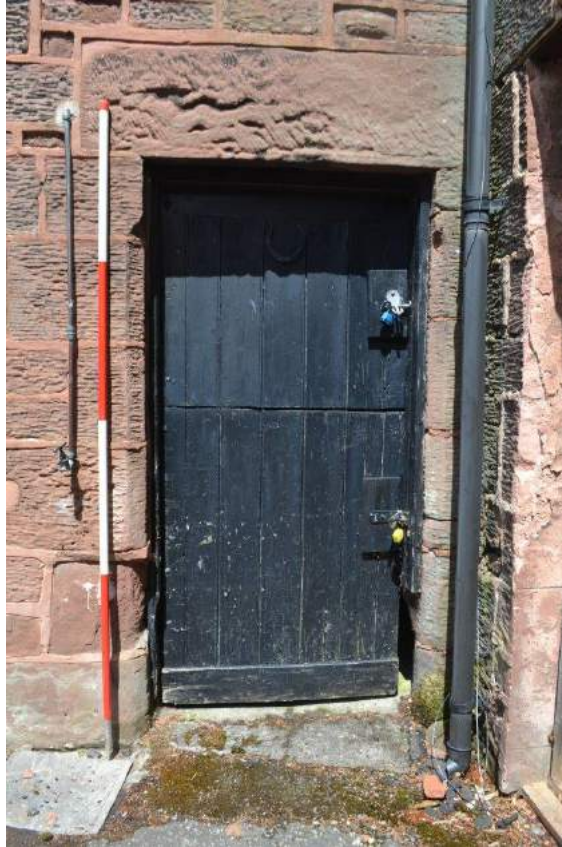
Plate 37: Detail of stable door from farmyard, with massive stone lintel and chamfered dressings. Stable floor is flush with farmyard surface
