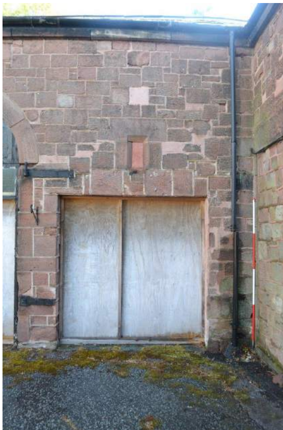
Plate 14: Detail of the inserted doorway to the right of the cart-entrance
