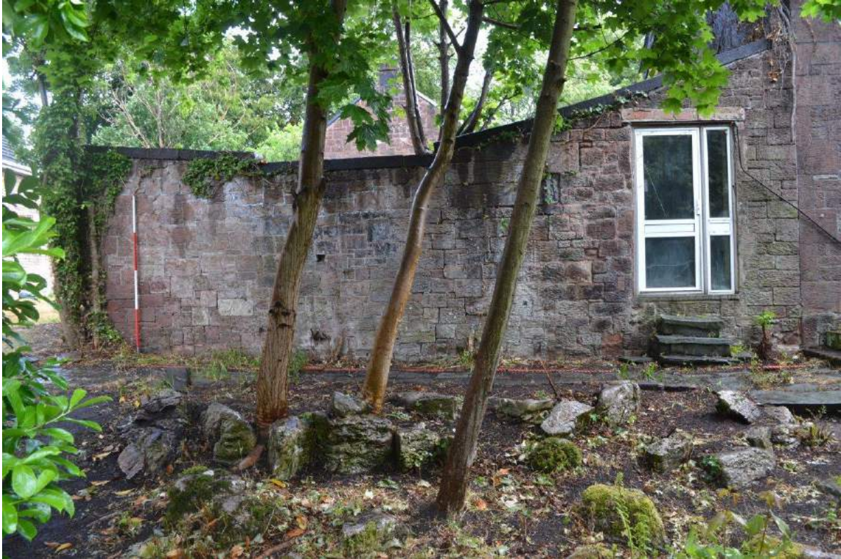
Plate 108: Sightline to the west showing the stone-built west-facing elevations of the WC and the Store. Shows, doorway in the Store providing access the garden with uPVC door and margin fenestration and butt-joint with the north-facing gable elevation of the western wing of the Farmhouse.
