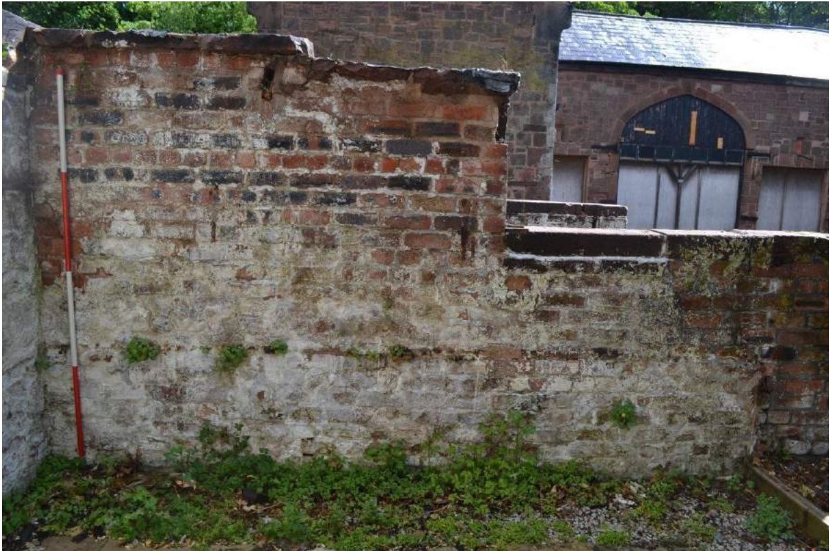
Plate 102: Inside face of the brick-built eastern wall to the second stall.
