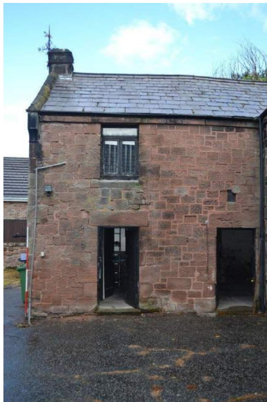
Plate 36: Sightline to the north towards south-facing elevation of the door (to right-hand side) to the stable (and the workshop) from the farmyard.
