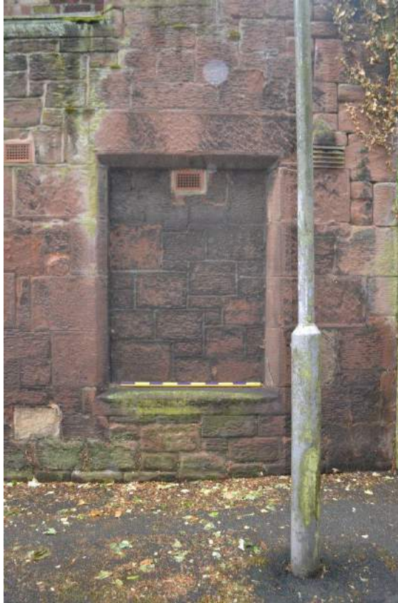
Plate 35: Detail of blind right-hand ground floor window with chamfered broached ashlar dressings
