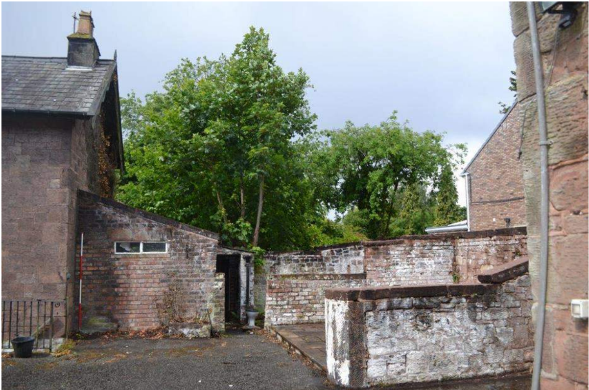
Plate 105: Sightline to the east from the farmyard showing the brick-built west-facing elevation single storey store, with twin-light window and mono-pitch roof, butted onto the north-facing gable end of the western wing of the farmhouse and the WC.
