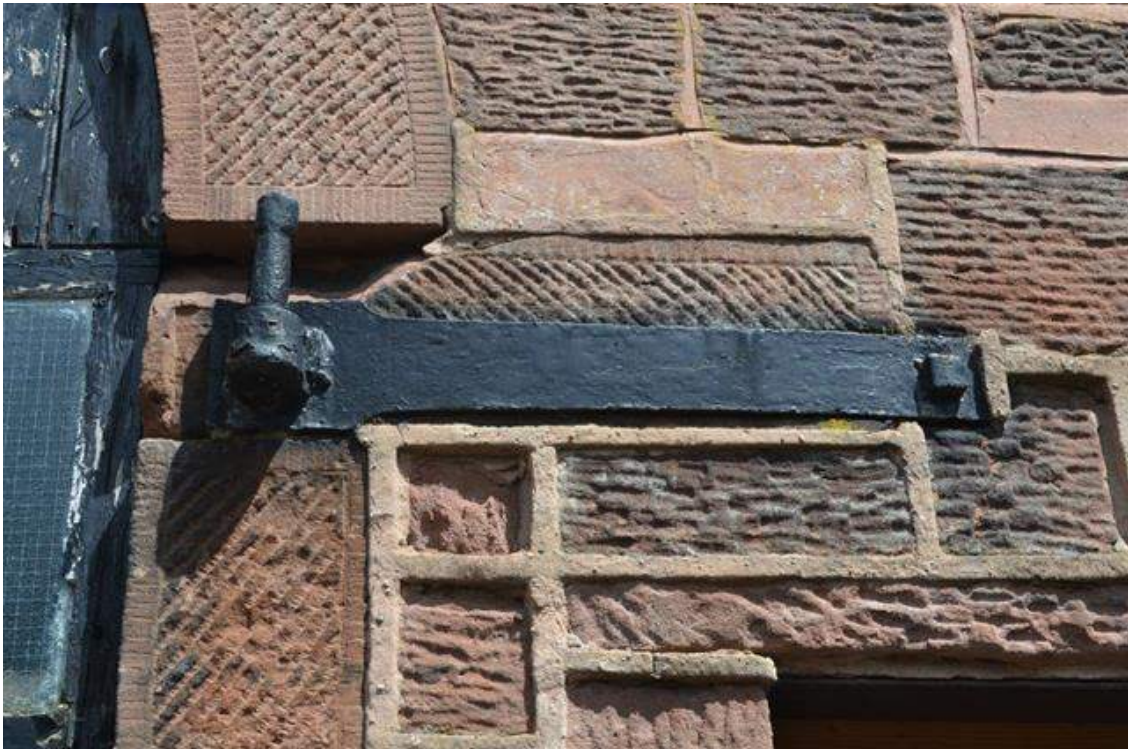
Plate 12: Detail of wrought-iron carcass hinge leaf and exposed pintle
