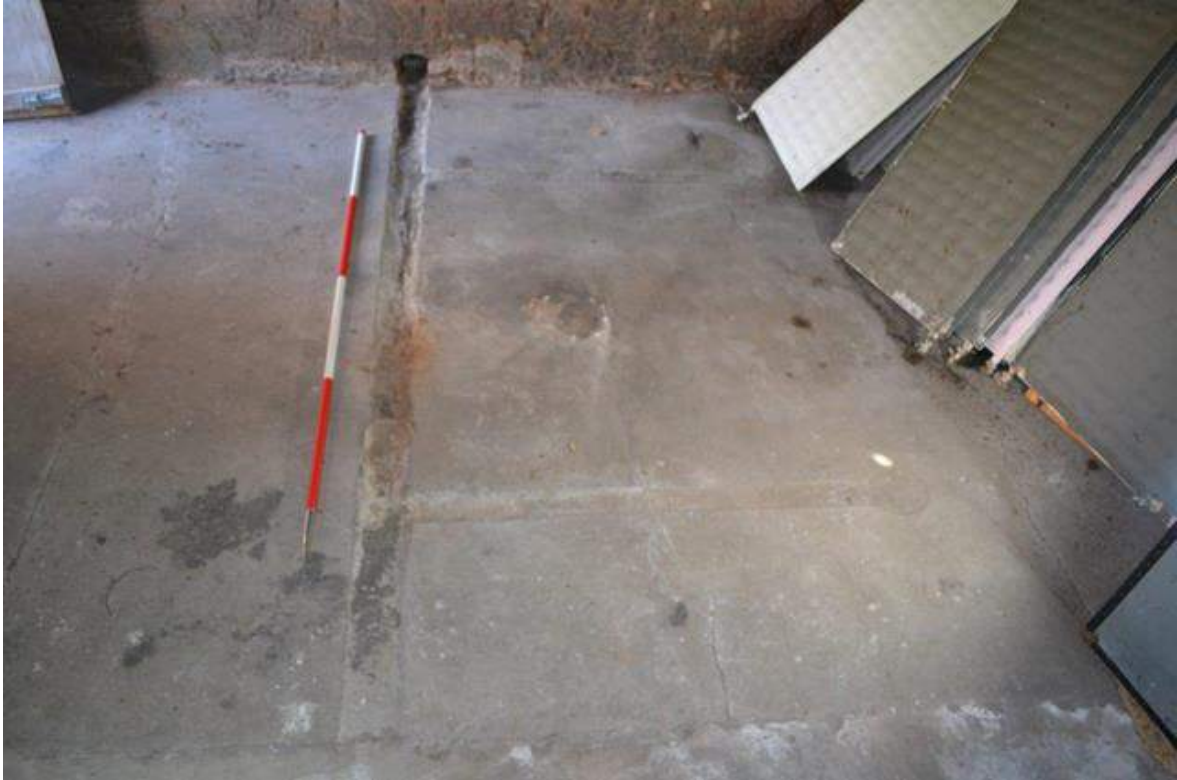
Plate 20: Concrete floor of the barn, with shallow channels leading to an aperture in the northern wall.
