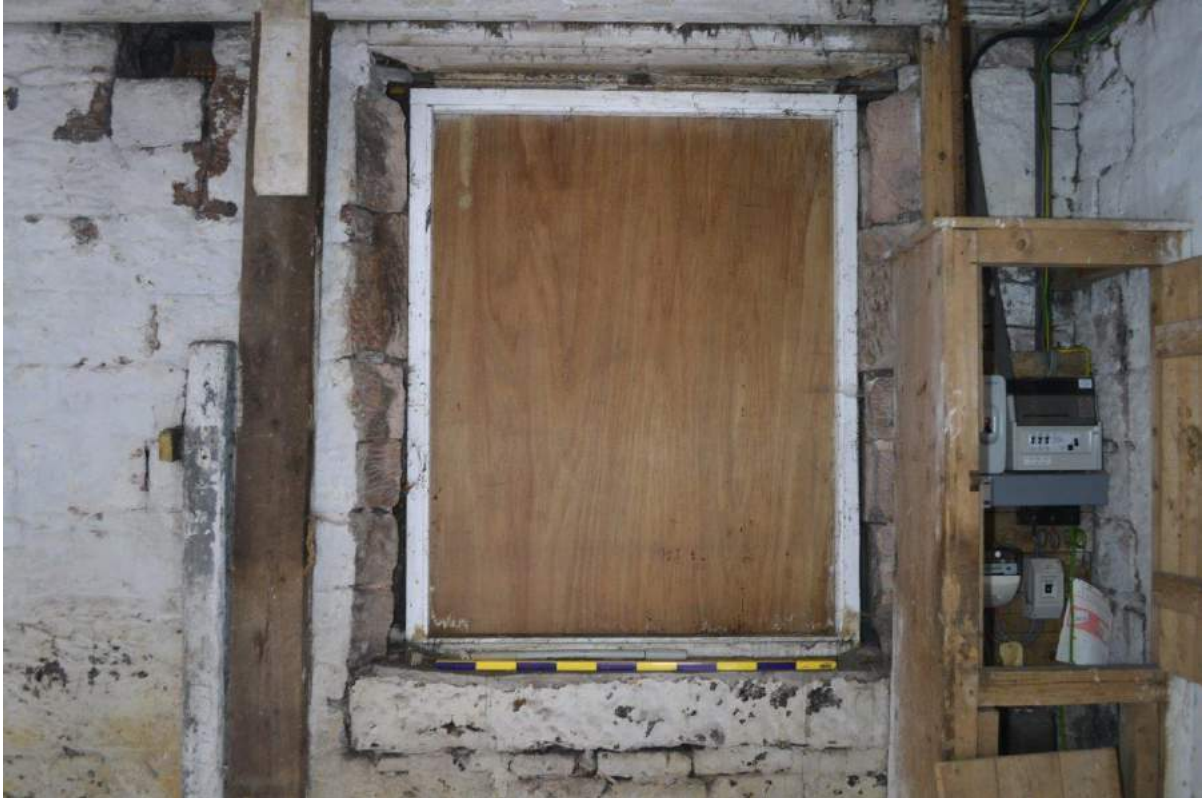
Plate 44: Stable ground floor, detail of boarded window opening in east-facing gable elevation. Stone sill, lintel obscured by joists. Scale = 1m.
