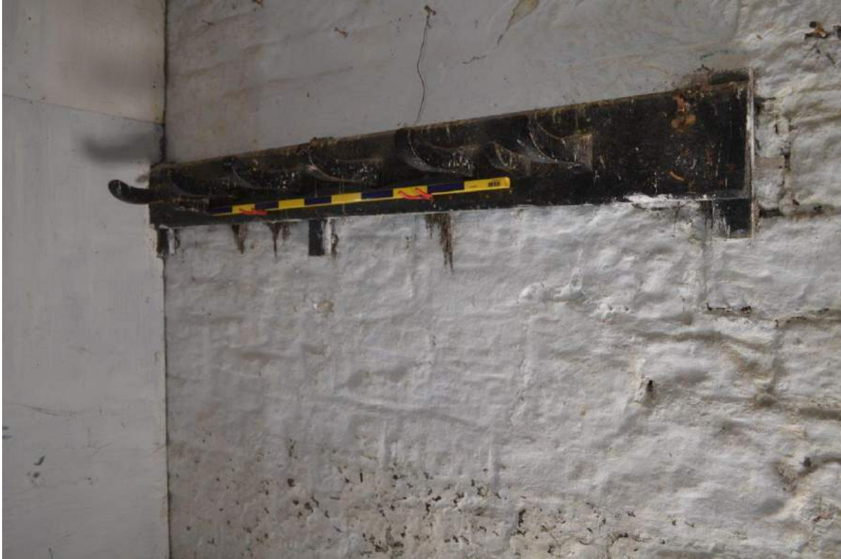
Plate 50: Stable, ground floor, detail of timber tack rack with seven hooks.
