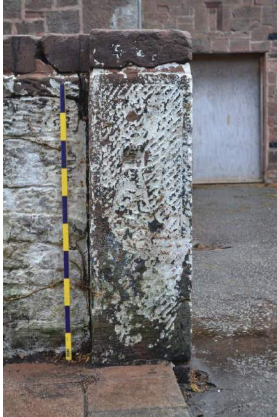
Plate 99: Sightline to the west, showing the broached stone pillar at the southern terminal of the east-facing elevation of the pigsty. Scale = 1m.
