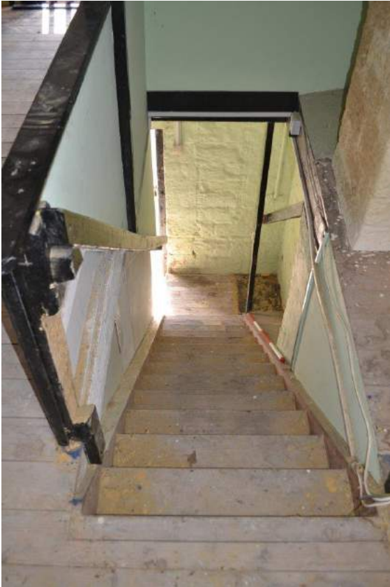
Plate 79: First floor, Workshop, sightline down the staircase. Chimney breast to right
