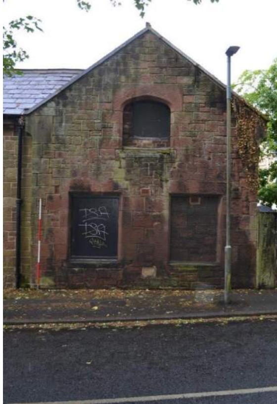
Plate 33: Sightline to the east-facing gable elevation of the stable, with two ground floor rectangular window openings and a single first floor window with carved lintel mimicking a multi-centred arch, possibly a four-centred Tudor arch. There are two projecting corbelled gable skews (not strictly kneelers as although they have horizontal beds their tops do not, wholly or in part, conform to the slope of the gable)
