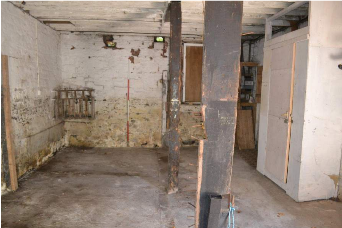
Plate 42: Sightline within the ground floor of the stable towards the east-facing gable elevation. Showing the concrete floor, the two posts defining the stalls, the corner hay rack, the boarded window opening and the joists supporting the first floor.
