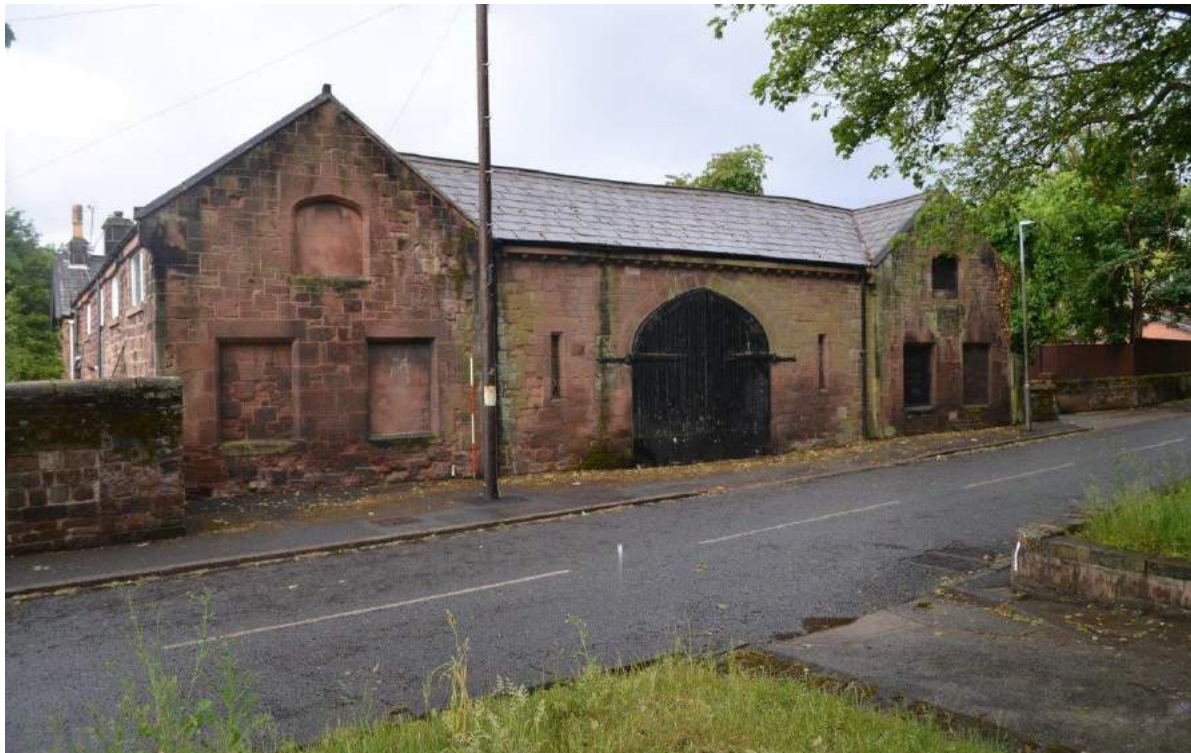
Plate 6: Sightline to the north-west showing the east-facing elevation of (from left to right) the boundary wall, the east-facing gable elevation of the farmhouse (with three blind windows), the barn with its cart-entrance doors and two arrow-slit vents and the east-facing gable elevation of the stable with its blind window and boarded-up windows.
