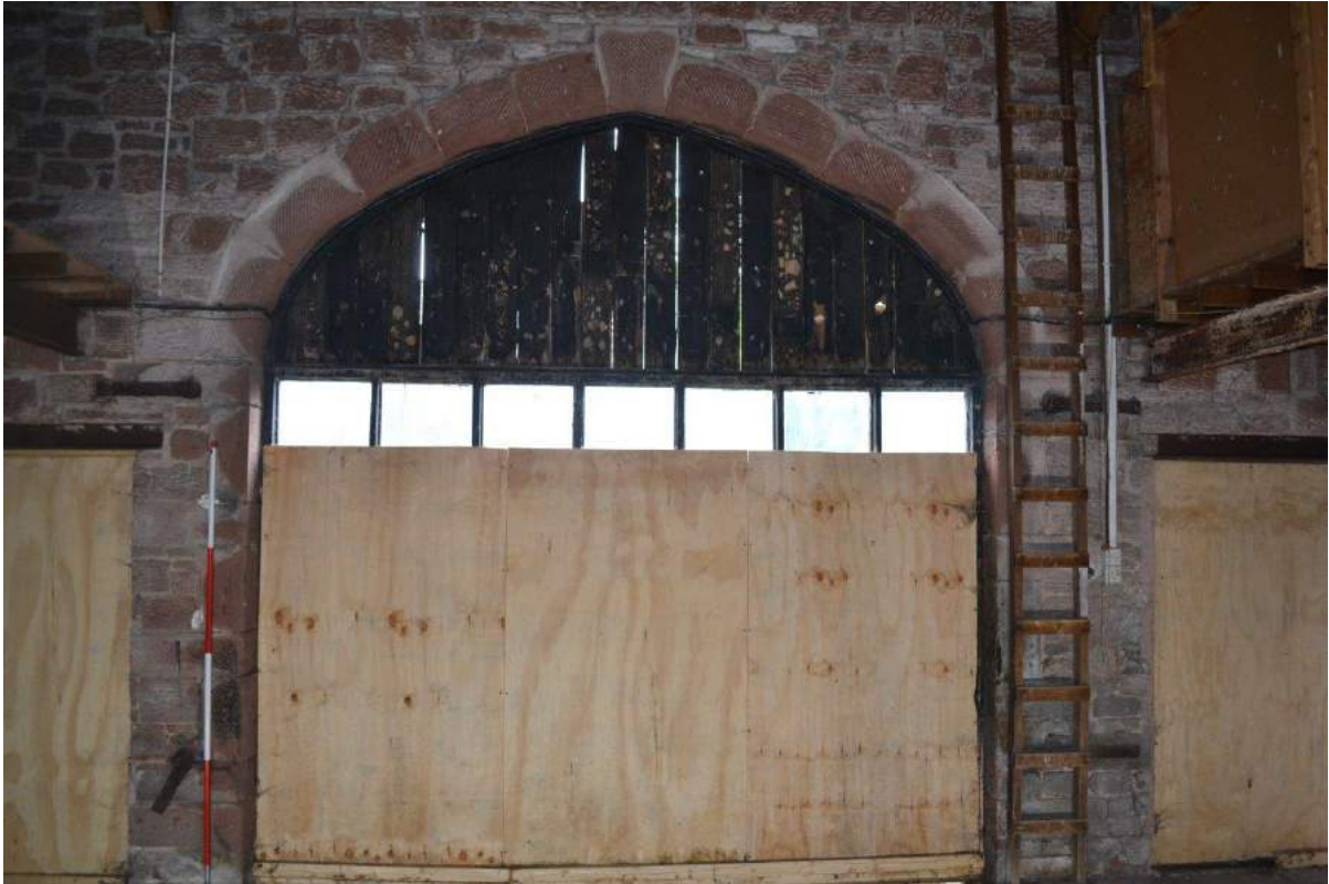
Plate 19: Inside details of the blocked cart-entrance doorway in the west-facing elevation.
