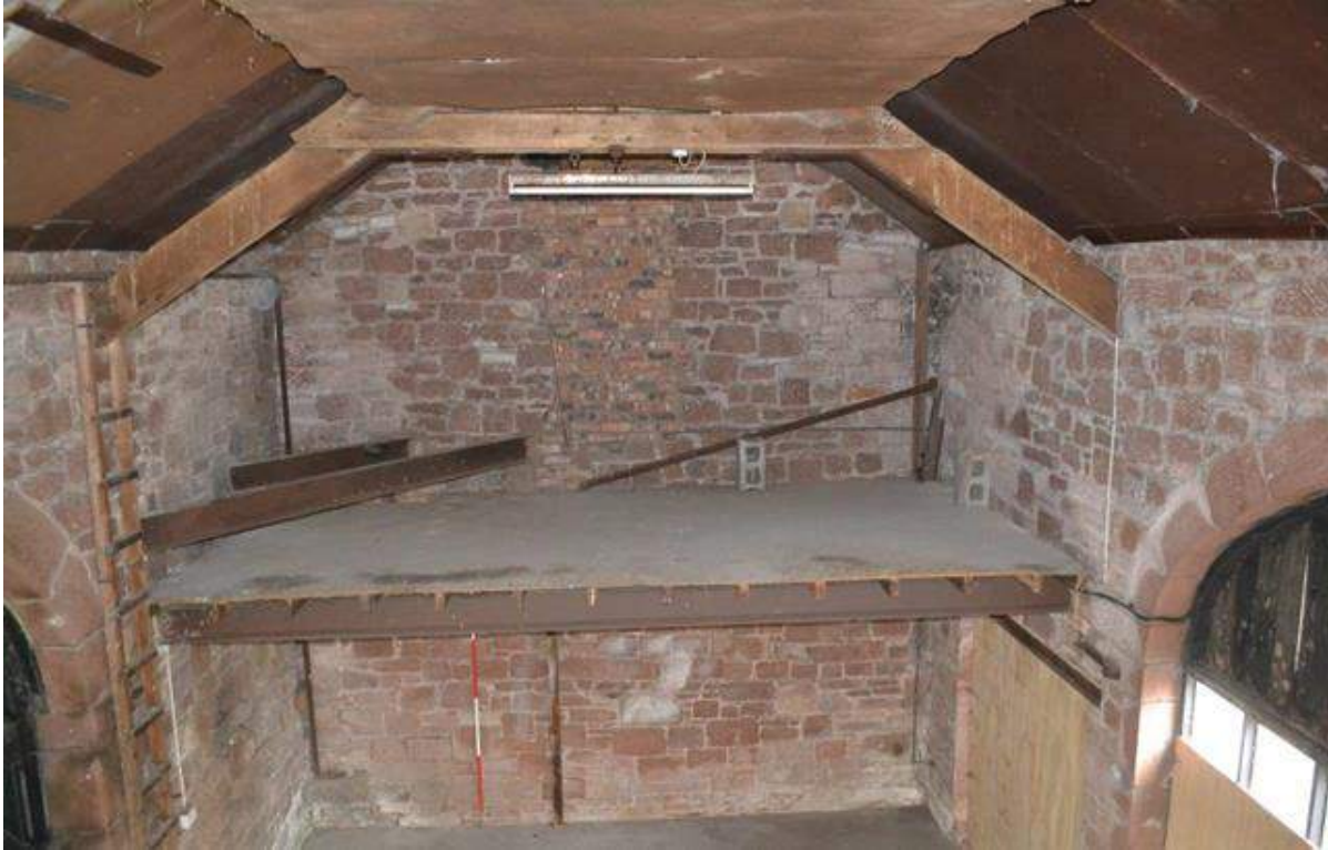
Plate 22: Sightline to the mezzanine floor at the southern end of the barn highlighting the board floor, joists and rolled steel joist. Also visible bricked-up door way into the first floor of the farmhouse, diagonal pair of rolled steel joists linking the gable wall to the east-facing flank wall and the raised tie-beam and principal rafter of the roof truss. Note absence of visible purlins.
