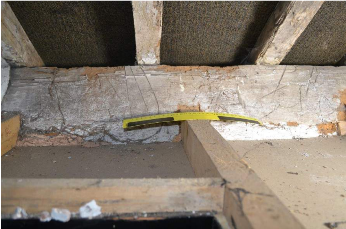
Plate 88: Roof space, Workshop, with incisions (unconvincing either as possible carpenter's marks or apotropaic marks – demon trap?) on canted purlin on which the common rafters rest. Scale = 30cm
