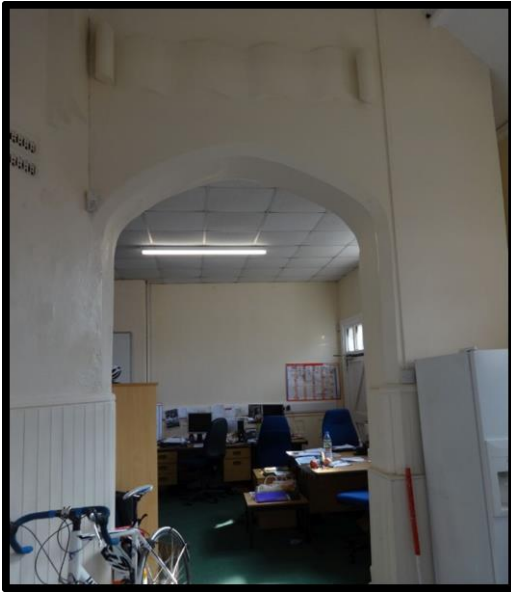
Fig. 21 The archway and scroll in the front gable of the early 1870s covered playground or schoolroom in the south-eastern range.
