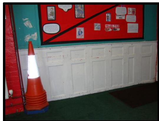
Fig. 18 Reused early 19th-century box pews from the old church reset in the school buildings.
