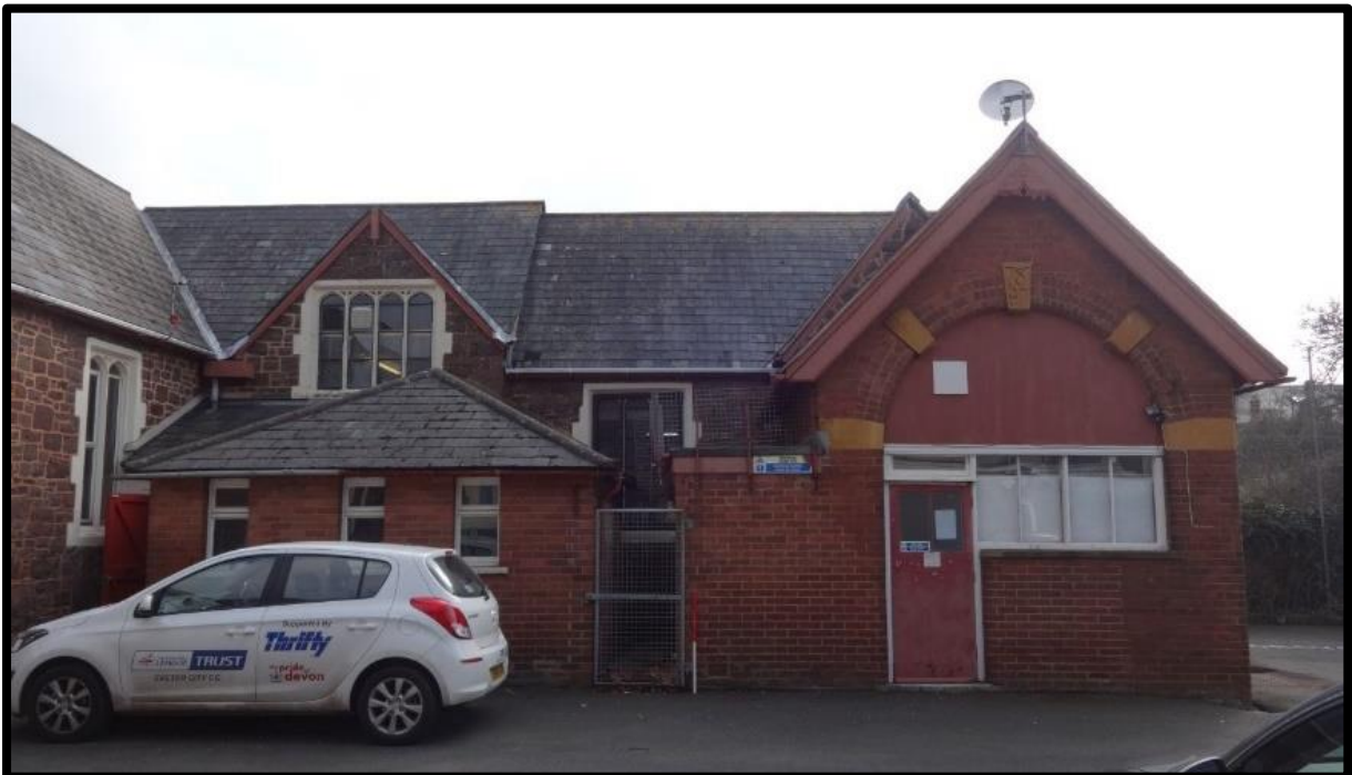
Fig. 20 View of the façade of the south-eastern range, showing the gabled chicket and high-level window of the former Master's House (left), the gabled extension of the early 1870s schoolroom (centre) and the new classroom of 1897 standing in front of this (Right). The brick cloakroom and lavatory blocks adjoining were added after 1902.
