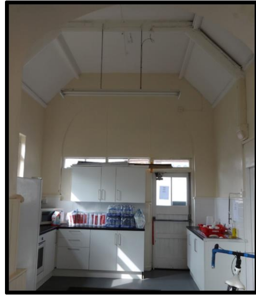
Fig. 22 View within the 1897 classroom added to the front beyond the arch, showing the carved corbels, high, boarded dado and ceiled roof.
