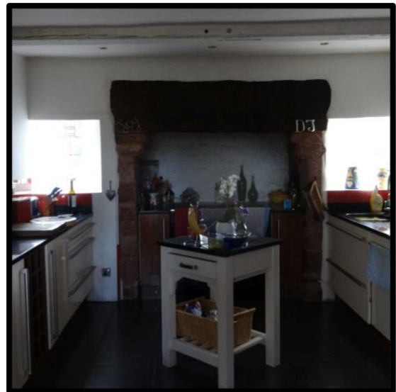
Fig. 14 The fireplace in the ground-floor kitchen, showing the truncated lintel, cut to accommodate two small side windows, and the rebuilt stone jambs beneath.
