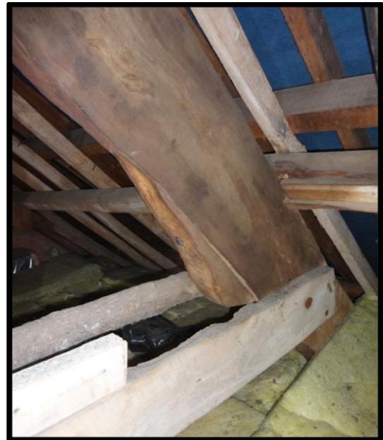
Fig. 20 Detail of the western foot of Truss III showing a similar timber cleat or wedge, now redundant, but perhaps part of an earlier partition.
