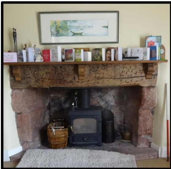
Fig. 13 The fireplace in the ground-floor drawing room, showing the curved stone brackets of local breccia supporting the timber lintel. This fireplace is possibly of 16th-century date.
