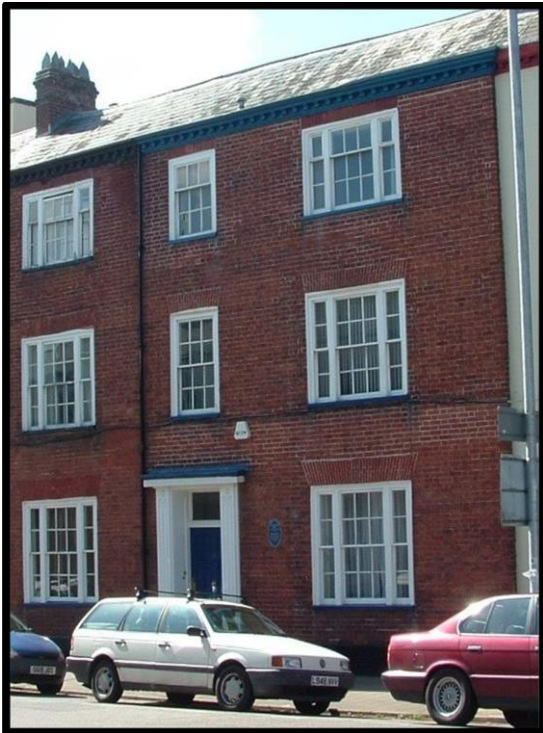
Fig. 8 View of Heathcote's House, Tiverton, showing tripartite sashes, with glazing bars, of late 18th- or early 19th-century date, probably similar to those originally at Harrington Farm.
