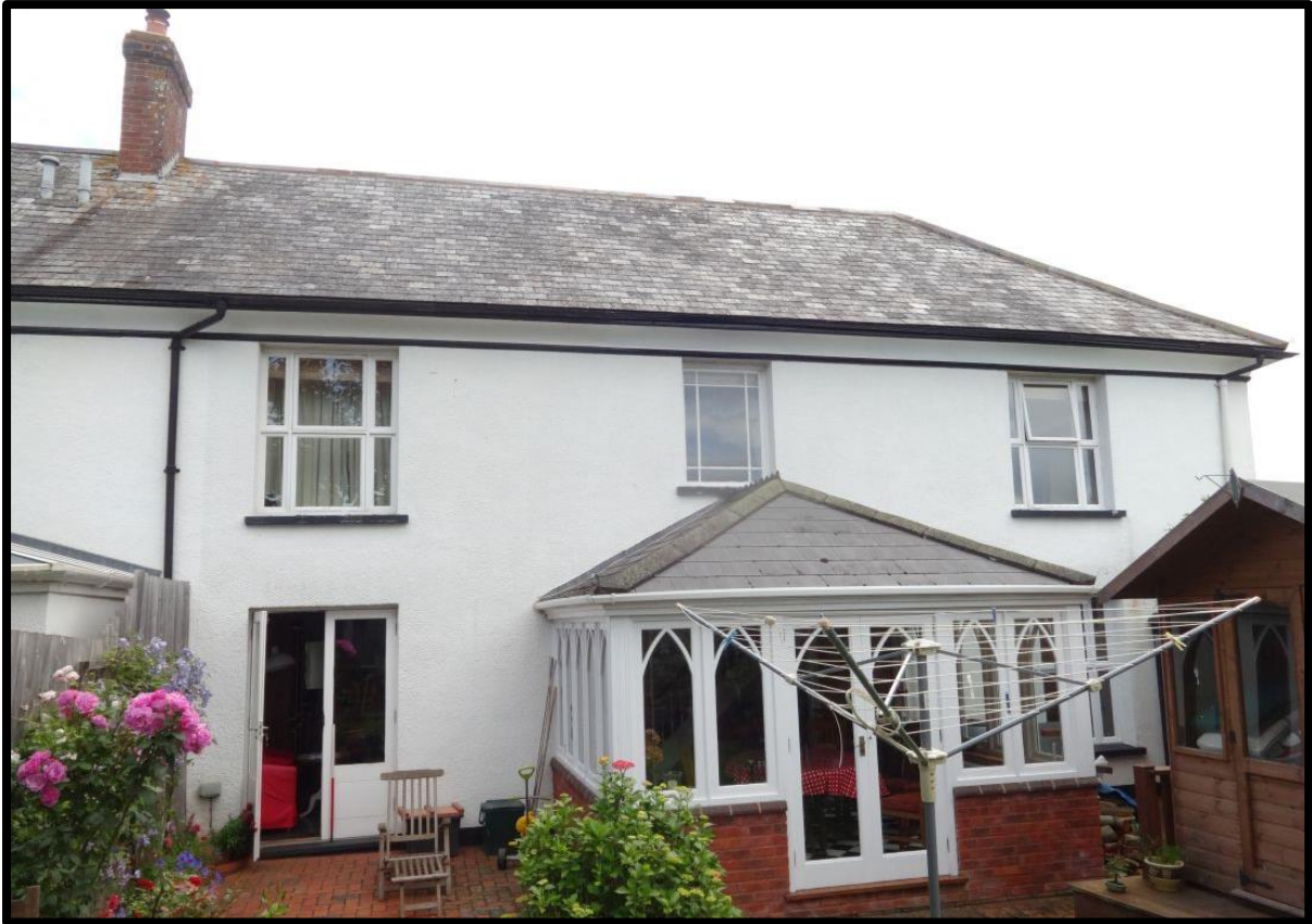
Fig. 4 West elevation of the farmhouse showing the modern replacement windows and the covered cornice of late 17th- early 18th -century type running below the roof at eaves level.
