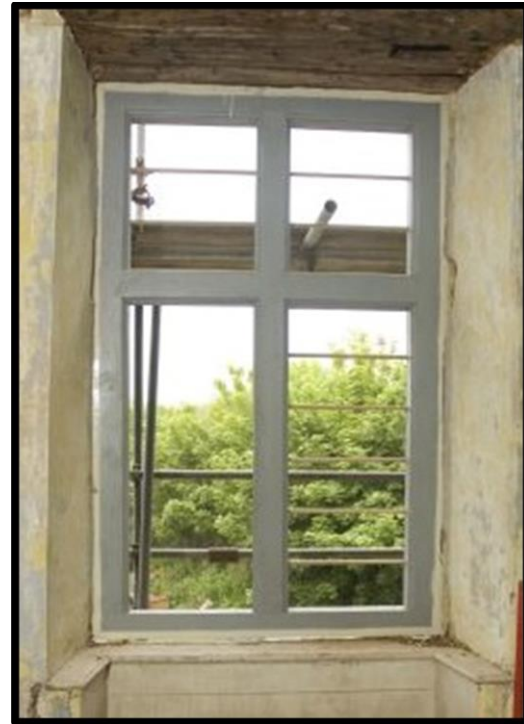
Fig. 9 A window from Yarde Farm, Malborough, dating from 1718 showing a mullion-and-cross frame (metal casements missing). The early windows at Harrington Farm may have been of this type.
