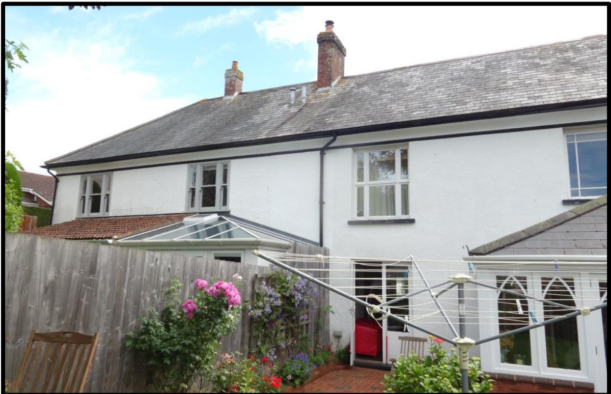
Fig. 5 West elevation of the northern part of the farmhouse, now a separate property, showing tripartite sash windows and the coved cornice continuing across the whole façade.
