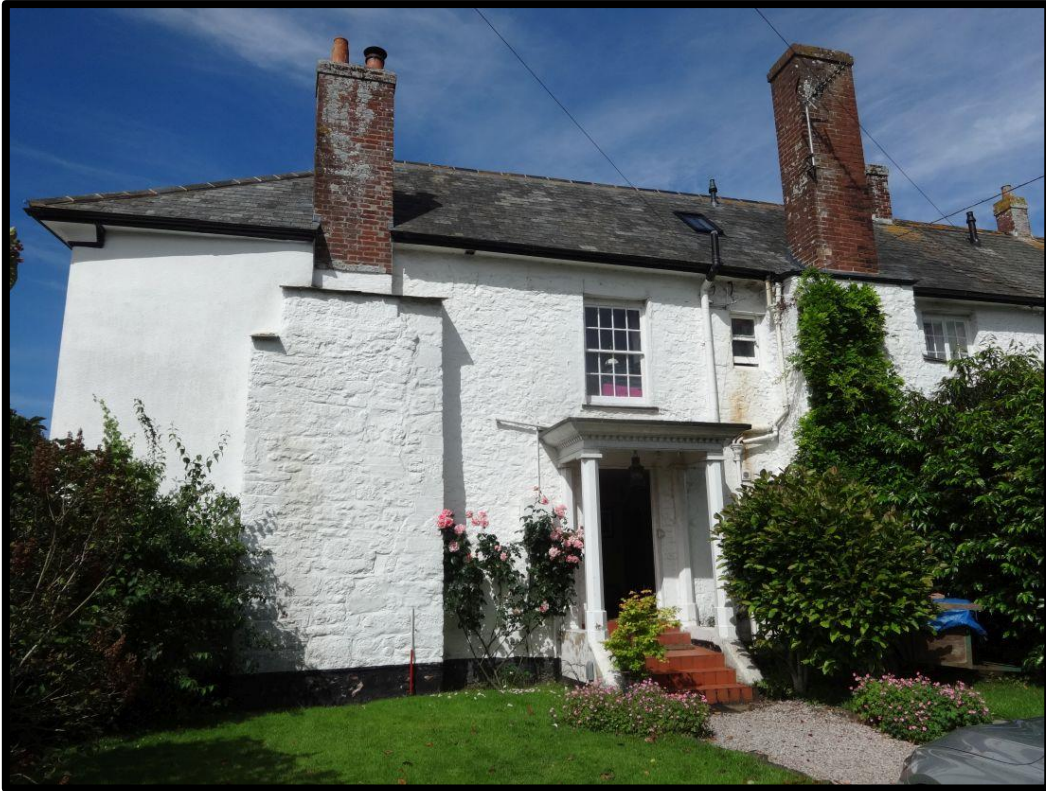
Fig. 10 East elevation of the farmhouse, showing the enormous chimney stacks and the portico.
