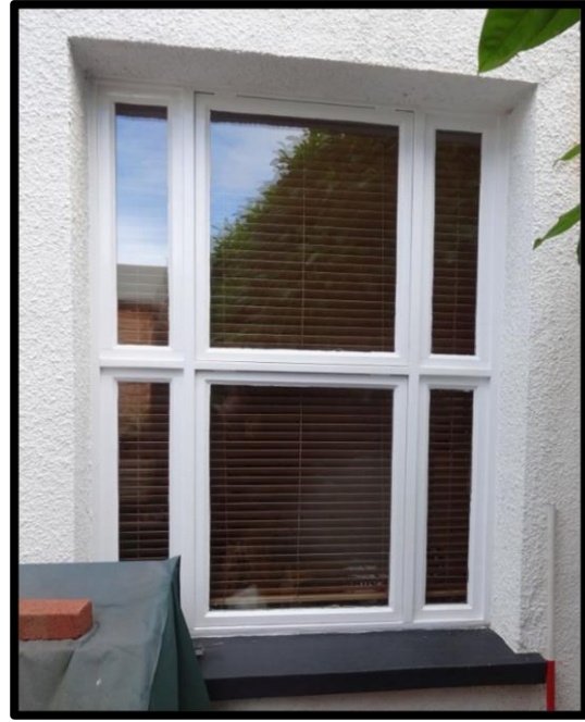
Fig. 7 Detail of one of the modern tripartite top-hung casements, probably inserted in place of earlier sashes in c.1987.
