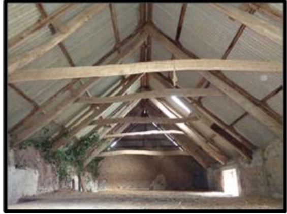
Fig. 53 The roof and loft over the stables.
