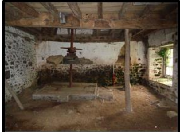
Fig. 47 The interior of the poundhouse, showing the cider press and the construction of the loft floor.
