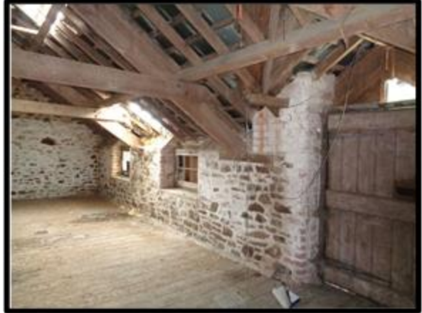
Fig. 45 The interior of the granary, looking north-east.
