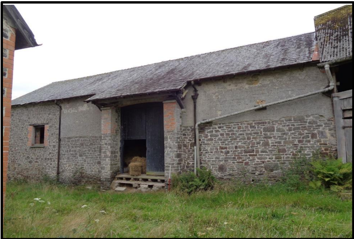
Fig. 23 The north elevation of the threshing barn, showing the secondary extension to its east end (left) and the 19th-century pent roof over the main doors.
