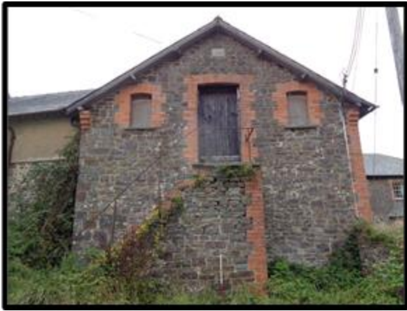
Fig. 42 The gable end of the granary showing the loft access.
