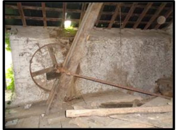
Fig. 49 The remains of a belt drive and transmission shaft above the doorway in the north wall of the poundhouse loft.
