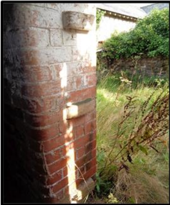
Fig. 56 The unusual projections at the piggery door jambs.
