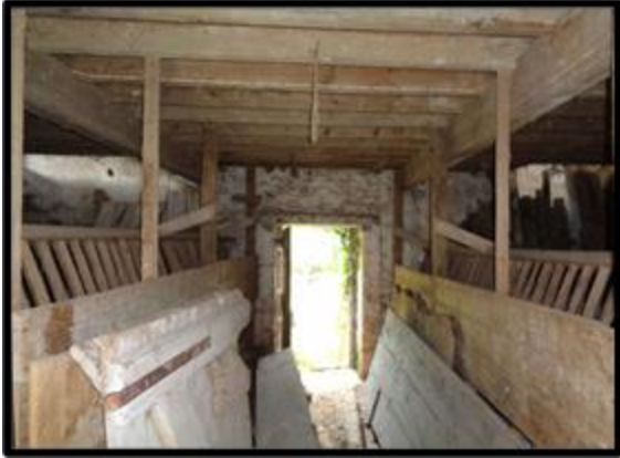
Fig. 52 The interior of the stable showing the head walk forming a cross passage through the building.
