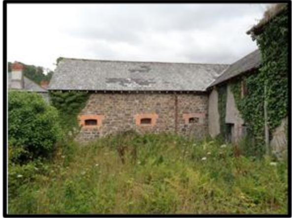
Fig. 43 The rear elevation of the granary showing possible stable ventilator windows.
