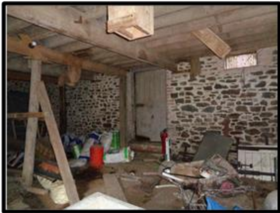
Fig. 44 The interior of the possible stable showing chutes from the granary floor above and the door to the poundhouse .
