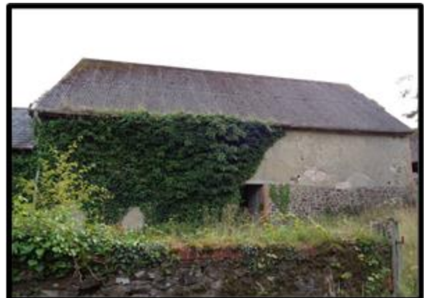
Fig. 51 The north elevation of the stables.
