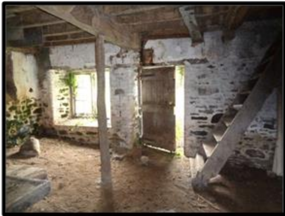
Fig. 48 The interior of the poundhouse looking towards the northern stair.
