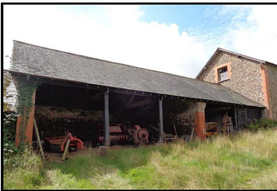
Fig. 18 The north elevation of linhay I.
