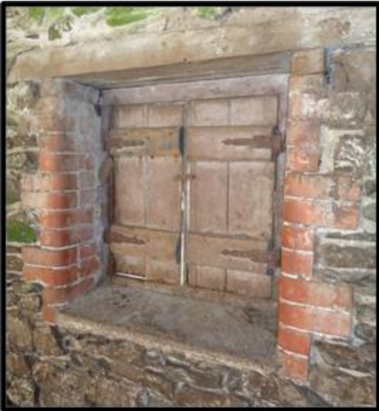
Fig. 27 One of the Shuttered windows of the horse-engine house.
