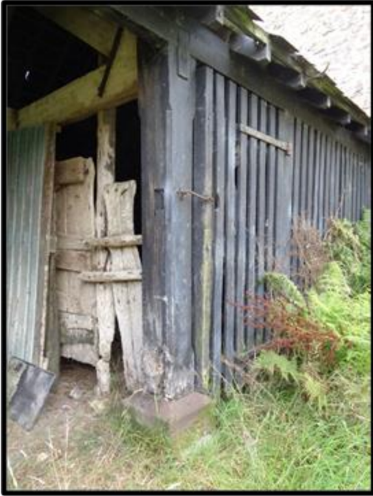
Fig. 21 Detail of the post and base supporting the western bays.
