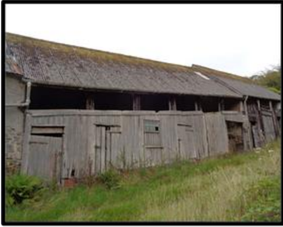
Fig. 29 The north front of Linhay II showing the late 19th-century enclosure of the lower part of the façade.
