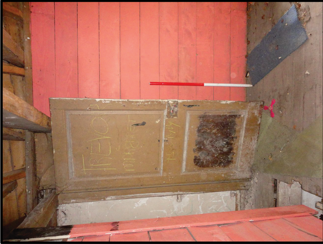
Fig. 23 Interior of the stables at first-floor level, showing a reused 18th-century door with two raised-fielded panels hung in the dividing partition.
