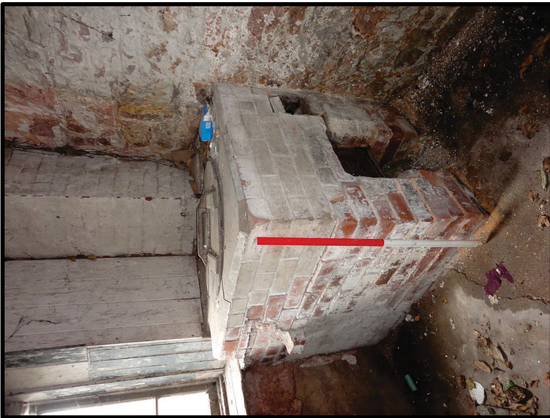
Fig. 23 Detail of the washing copper in the south-eastern corner of the stables showing the stokehole, flue and the timber lid.
