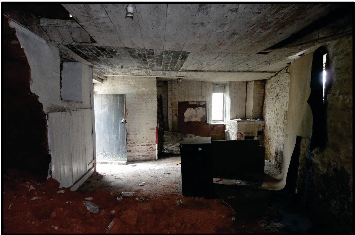
Fig. 21 Interior of the stables, looking east, showing the collapsed cob walling and the position of the washing copper in the south-eastern corner.
