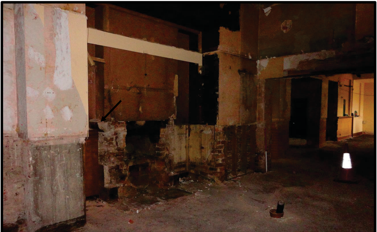
Fig. 17 View of the ground-floor rooms looking from the presumed site of the dining room to the site of the conservatory and the 1930s wing to the north, showing the remains of a chimney breast featuring a very large 'architectural' fireplace with a ovolo-moulded stone mantel shelf (arrowed), probably added as a feature in 1938-9.
