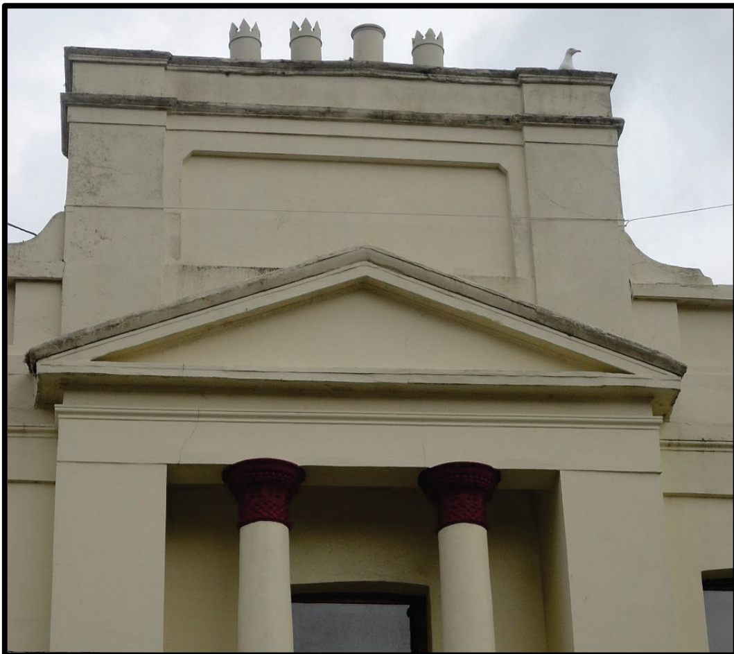
Fig 12 Detail of the pedimented aedicule and attic masking the chimneys on the south front of the house and showing the unusual 'basket-work' character of the capitals of the columns.
