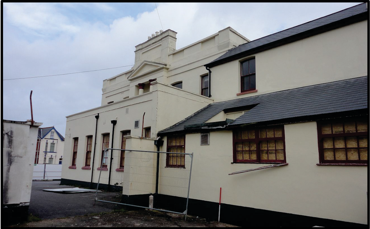
Fig. 13 The south elevation seen from the stable yard, showing the nucleus of the original house rising above the later 1930s porch extension added against its entrance façade (centre) and the lean to structure which might represent parts of the original central service range (right).
