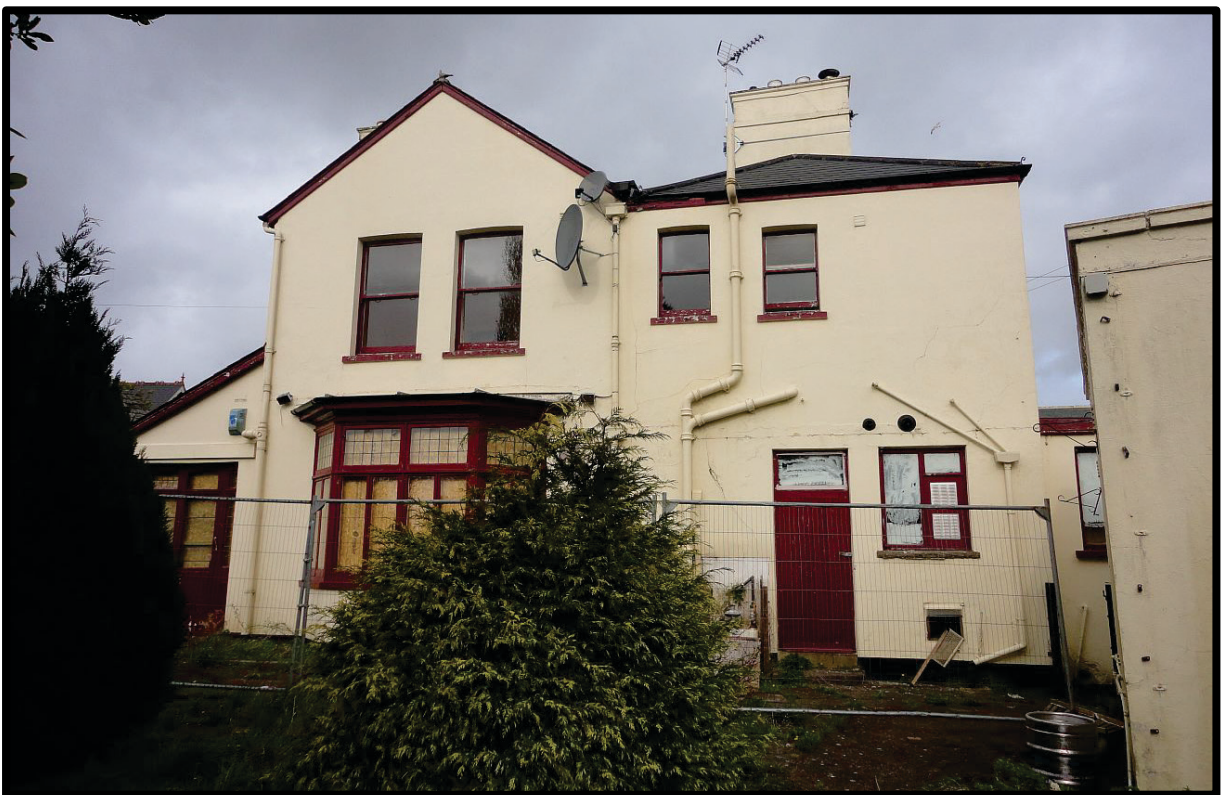
Fig. 14 The eastern elevation, showing the lean-to structure representing the remains of a further service range (left), the gabled elevation of the late 19th- or early 20th-century extension (centre) and the end of the original service wing (right).
