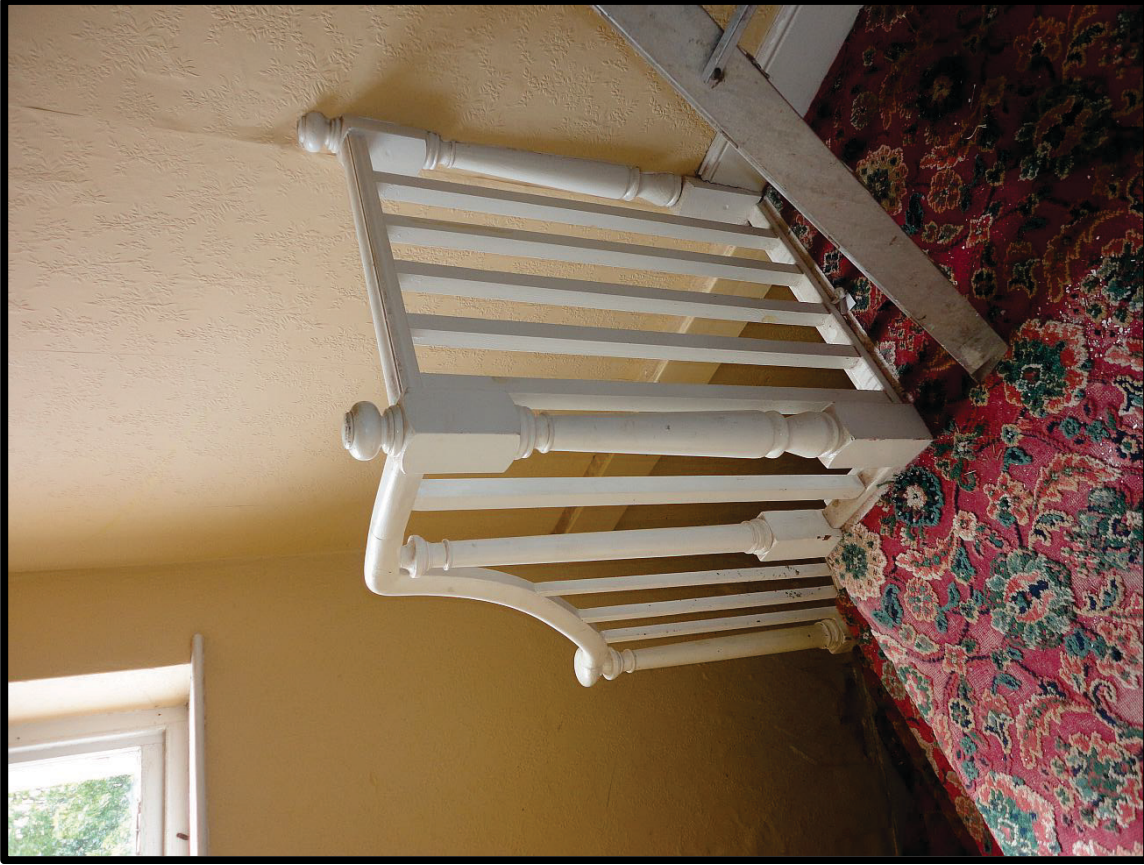
Fig. 19 Detail of the service stair, from first-floor level, showing the original balustrade with columnar newels curtailed by a late 19th-century section with ball finials.
