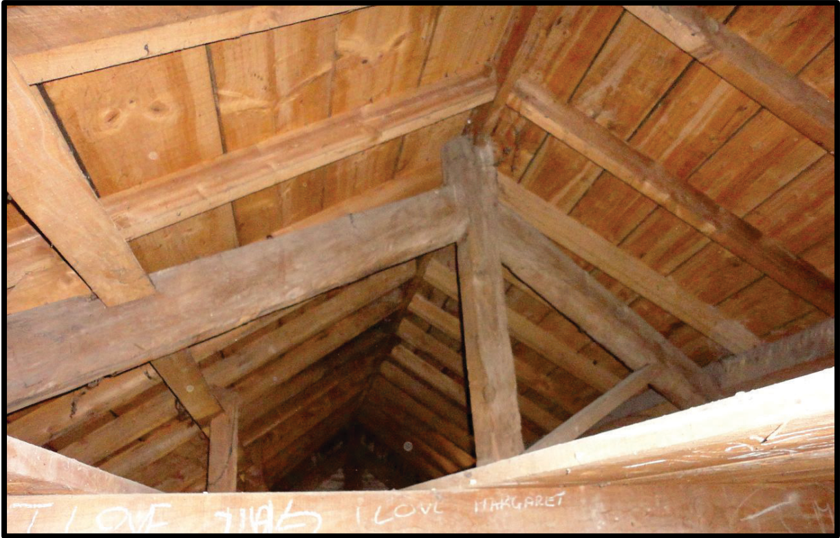
Fig. 24 The roof of the stable block, showing primary king-post trusses but later 19th- or 20th-century purlins, rafters and sarking boards.
