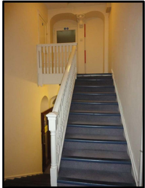
Fig. 24 View of the staircase showing the paired openings at the summit perhaps relating to an earlier stair turret.
