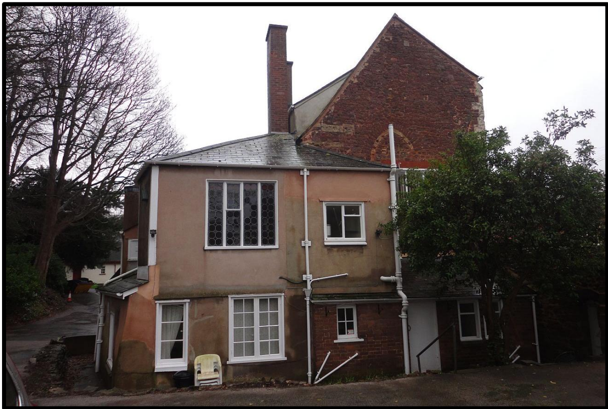
Fig.19 The north-western elevation of the projecting rear extensions, showing (extreme left) the angled wall possibly representing an early garden wall absorbed into a lean-to structure, the timber-framed structures at first-floor level above it and the later brick extension (right) underlying it against the original gable wall of the gatehouse.
