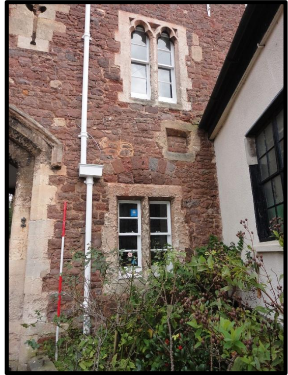
Fig. 12 Detail of the wall east of the gate, showing 19th-century windows and the remains of earlier features
