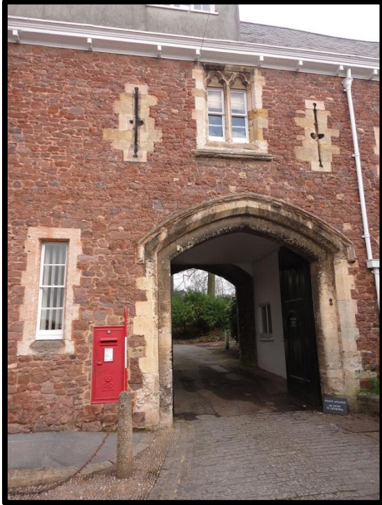
Fig. 11 Detail of the gateway, showing the arrow slits and varied geology of the window openings.
