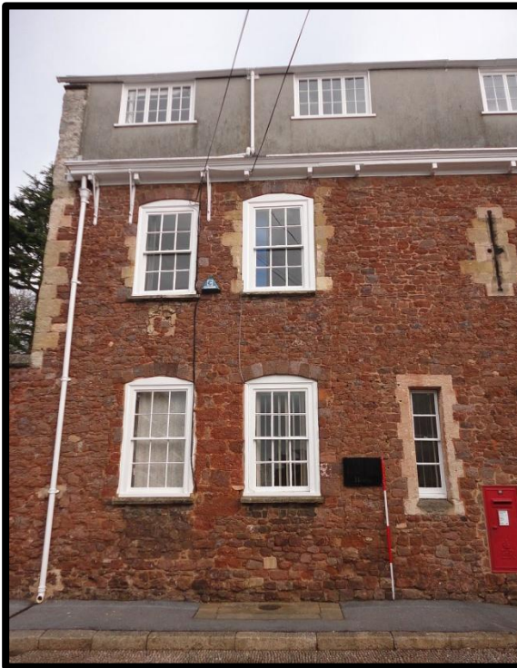
Fig. 13 Detail of the wall west of the gate showing the dressings around the first-floor window openings and the ground-floor windows cut into the walling.
