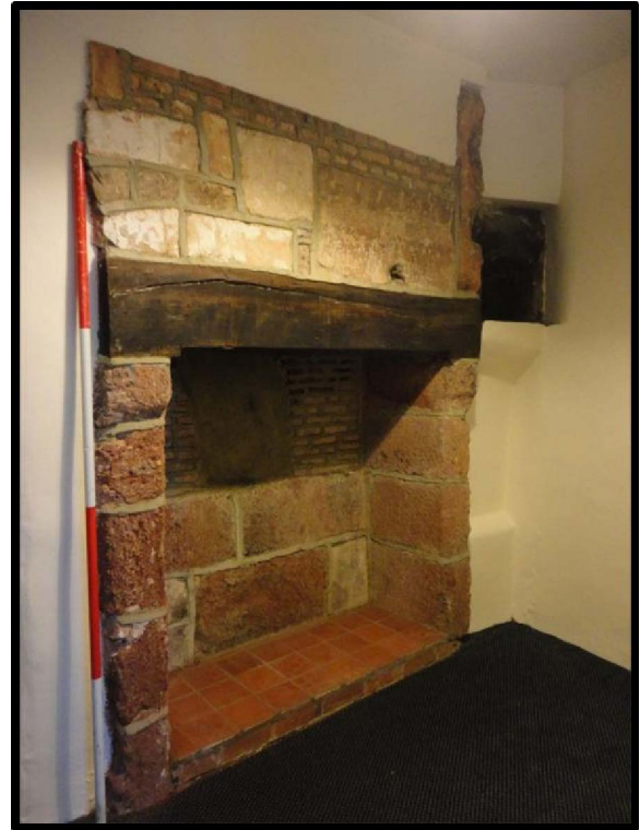
Fig. 29. Detail of the fireplace and oven in the eastern chamber, as rebuilt in the 17th-century by truncating a projecting hood.
