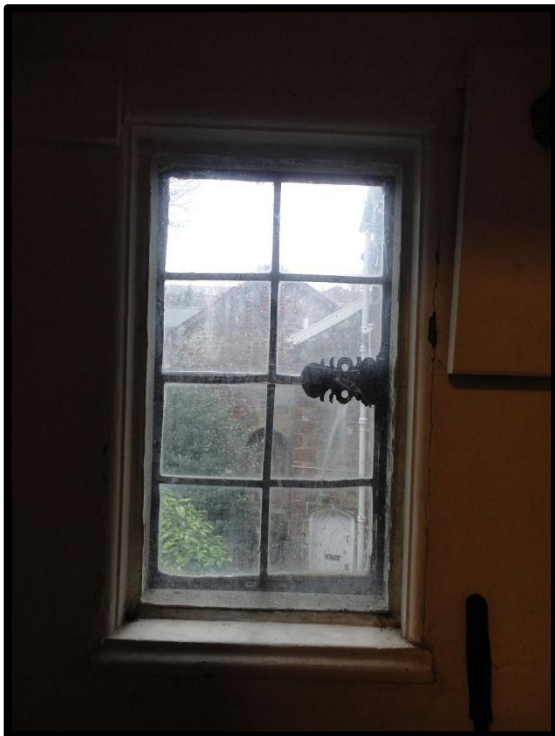
Fig.20 Detail of the 17th-century window casement in the stair wing added to the rear of the gatehouse, possibly associated with a 17th-century staircase.
