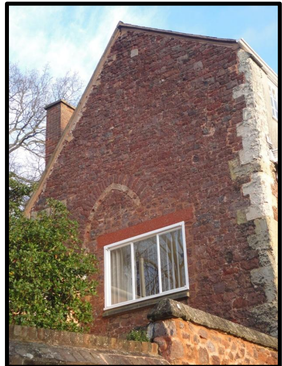
Fig. 14 Detail of the north-west wall of the gatehouse showing the remains of a very large arched window cut by a modern Crittall window.
