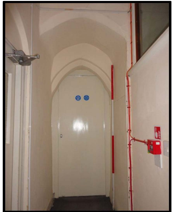
Fig. 26 Detail of the archway between the western chamber and the room over the gate passage showing a two-centred medieval archway rebated for a door opening into the chamber.
