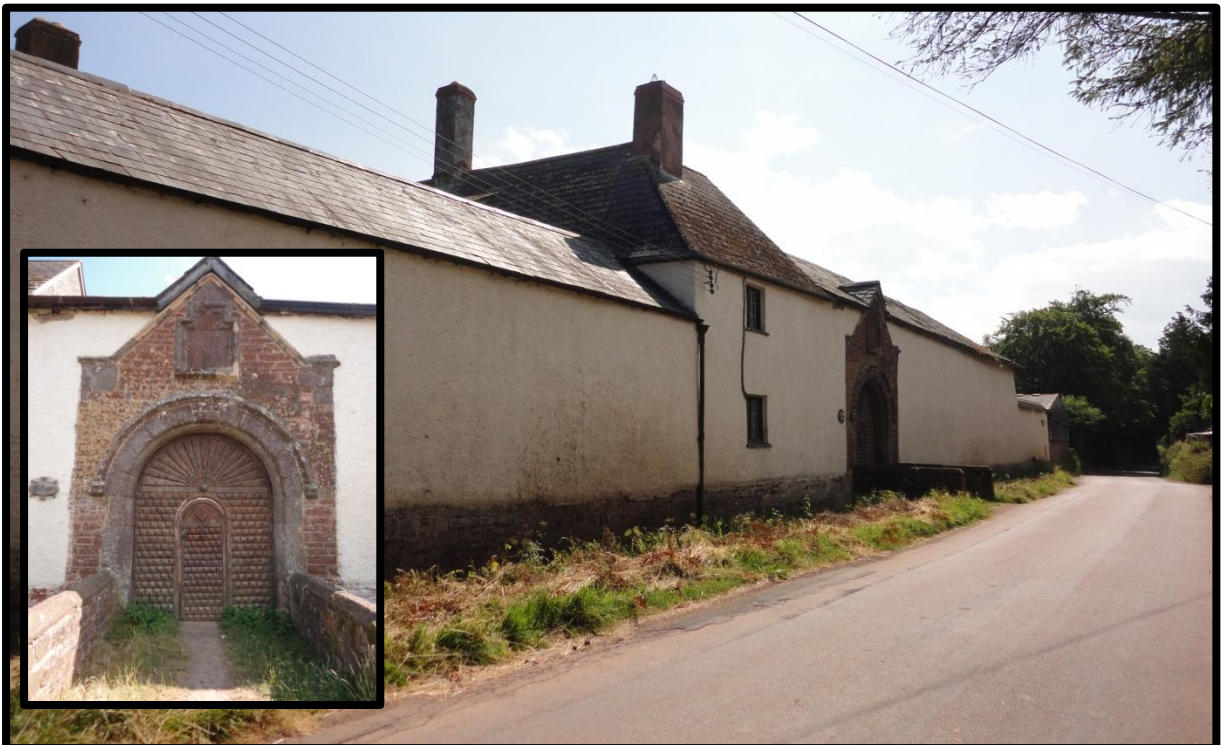
Fig. 3 General view of Widhayes, Uplowman, showing the gatehouse range of a Devon mansion of the late 16th or early 17th century (inset: a detail of the architectural frontispiece to the gateway). This may give an impression of the possible appearance of the mansion at Old Matford in its original state.
