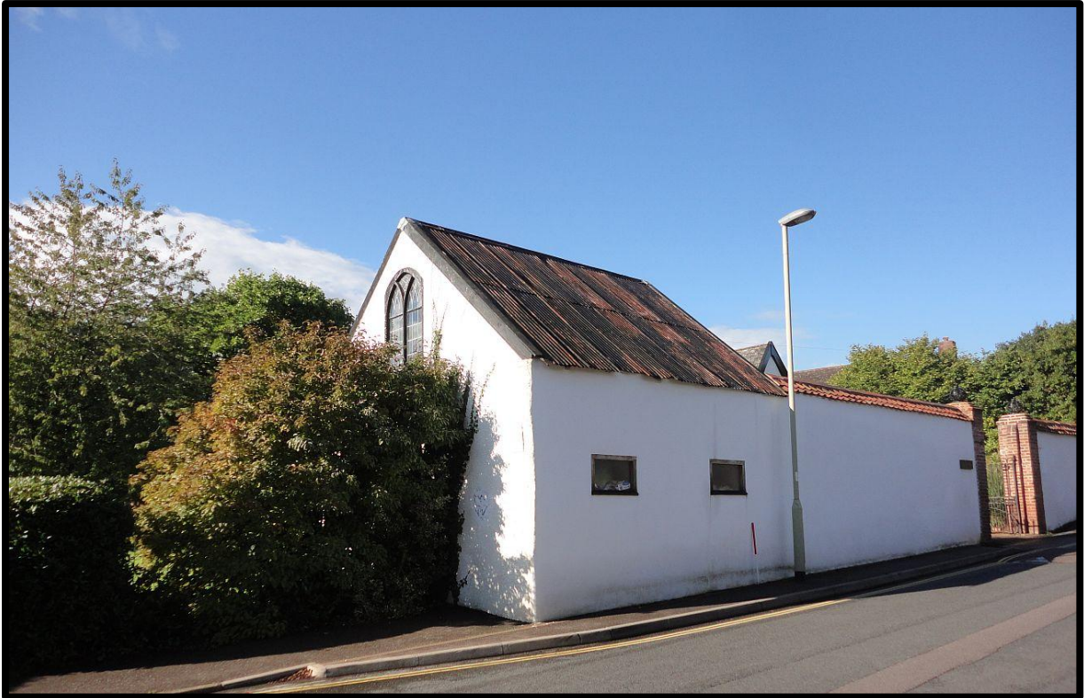
Fig. 2 General view of Old Matford from Wonford Road showing the outbuilding and the forecourt walls on the perimeter of the site.
