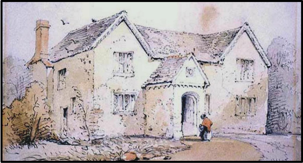
Fig. 1 The front elevation of Old Matford, from a 19th-century drawing by F.W.L. Stockdale, showing the modest scale of the surviving house.
