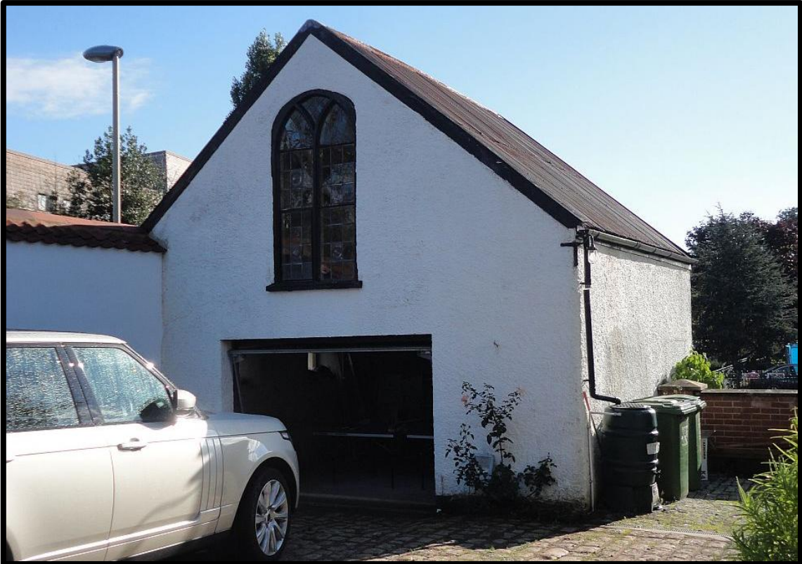
Fig. 8 General view of the garage building, looking east, showing its relationship with the site boundary wall to the north.
