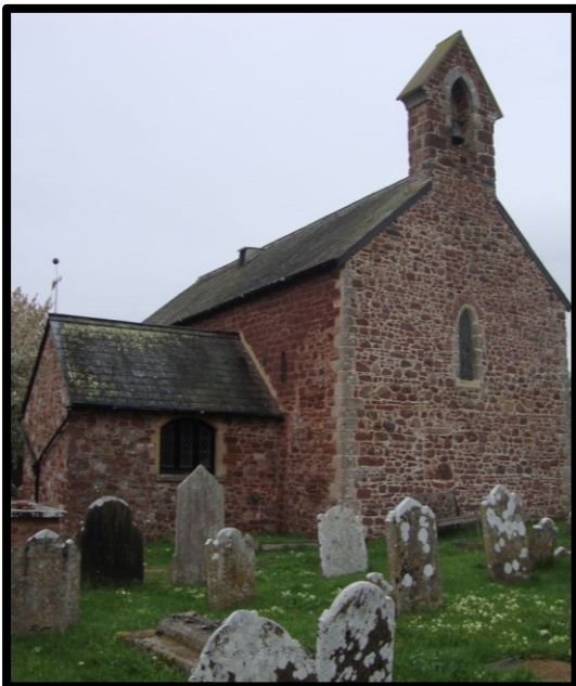
Fig. 6 The church from the north west, showing its simple un-aisled plan, as restored in the late 19th century, and the modern vestry attached to the north-western corner of the nave.
