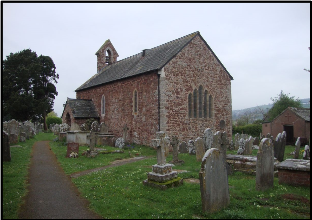
Fig. 2 General view of the church from the south east, looking north west, showing the simple rectangular form of the building, the densely-occupied churchyard, the fine group of 13th-century lancet windows at the east end and the 18th-century vestries at extreme right.
