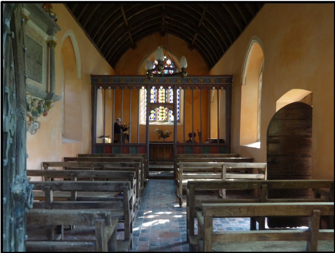
Fig. 27. The small, single-celled chapel at Ayshford, Burlescombe, Devon, showing features which are likely to have existed at St Nicholas, including a plain medieval rood screen, without a loft, and a wagon roof. The open benches shown are of 19th century date, but benches were in use in Devon from the 13th century.
