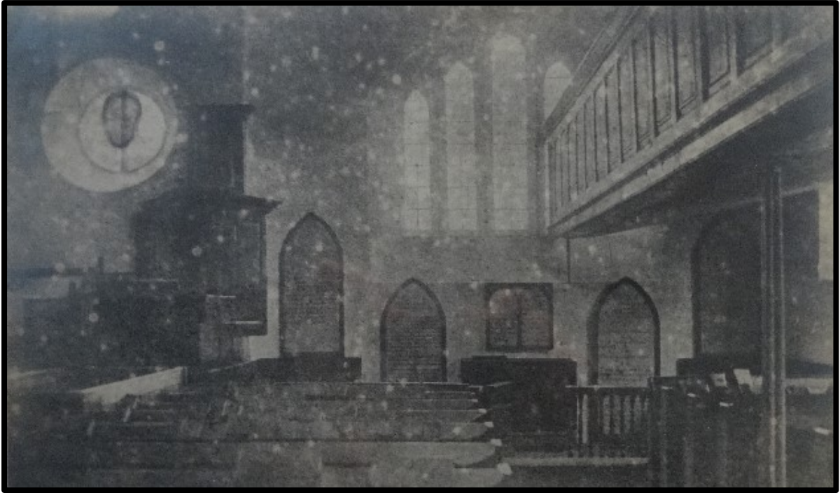
Fig. 11 Photograph of the interior in c. 1875 prior to restoration, showing the church as enlarged in 1790-1812 with the south gallery of 1822 still in place and both open benches and box pews (Photograph held by the PCC of St Peter with St Nicholas Shaldon).
