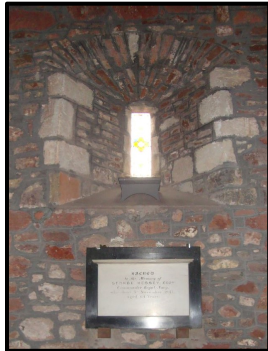
Fig. 20 The slit window seen from the interior showing the medieval jambs and vault to the embrasure.
