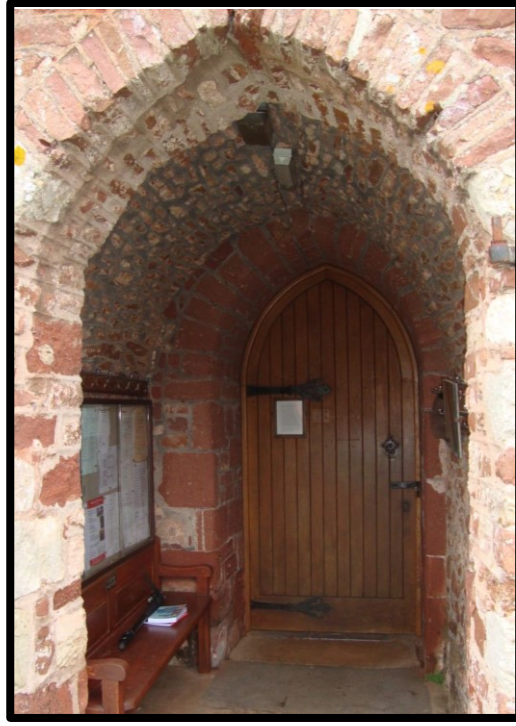
Fig. 5 The stone barrel vault of the porch, which with the graduated lancets of the east end may be the best surviving 13th-century fabric in the building.
