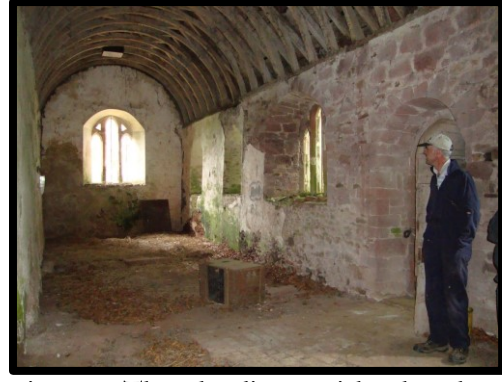
Fig. 26 The derelict parish church of Broadnymet in mid Devon, also a single-cell church of 13th-century date, but retaining its medieval wagon roof intact.
