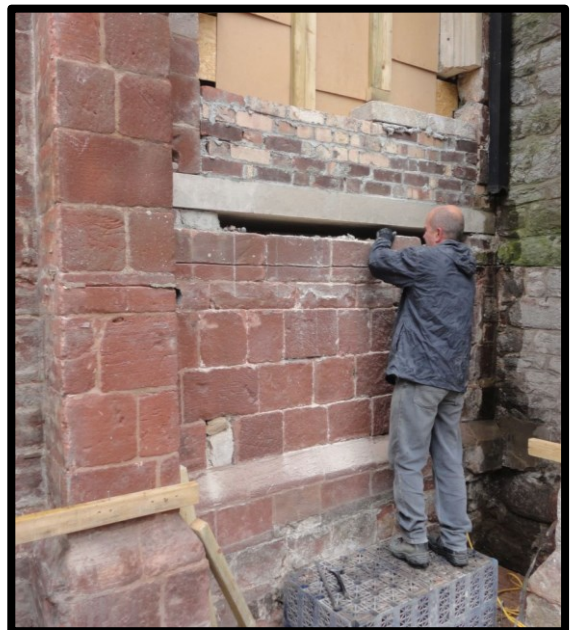
Fig. 10 View of the western elevation of the north aisle during the insertion of a concrete lintel for the new doorway and prior to the demolition of the medieval walling.
