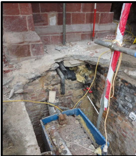
Fig. 9 View of the underground boiler house showing the brick lining of the room and the concrete capping which may have preserved the height of post-medieval ground levels.
