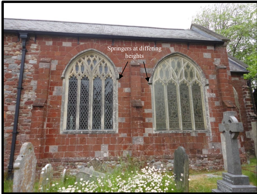
Fig. 5 Elevation of the east end of the south aisle showing evidence of discontinuity in otherwise apparently homogenous fabric.
