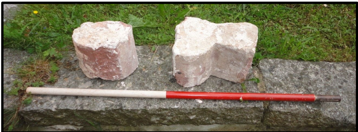
Fig. 14 Two shaped blocks recovered during the demolition of the west wall of the aisle, showing the characteristic 'keyhole' shape of the treads of a newel stair or vice.
