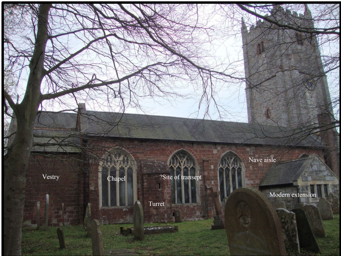
Fig. 6 Elevation of the north aisle showing apparently homogenous fabric with minor variations in the width of the windows. The easternmost bay represents a 19th-century vestry. The projecting turret for a rood stair might mark the eastern wall of a possible north transept.
