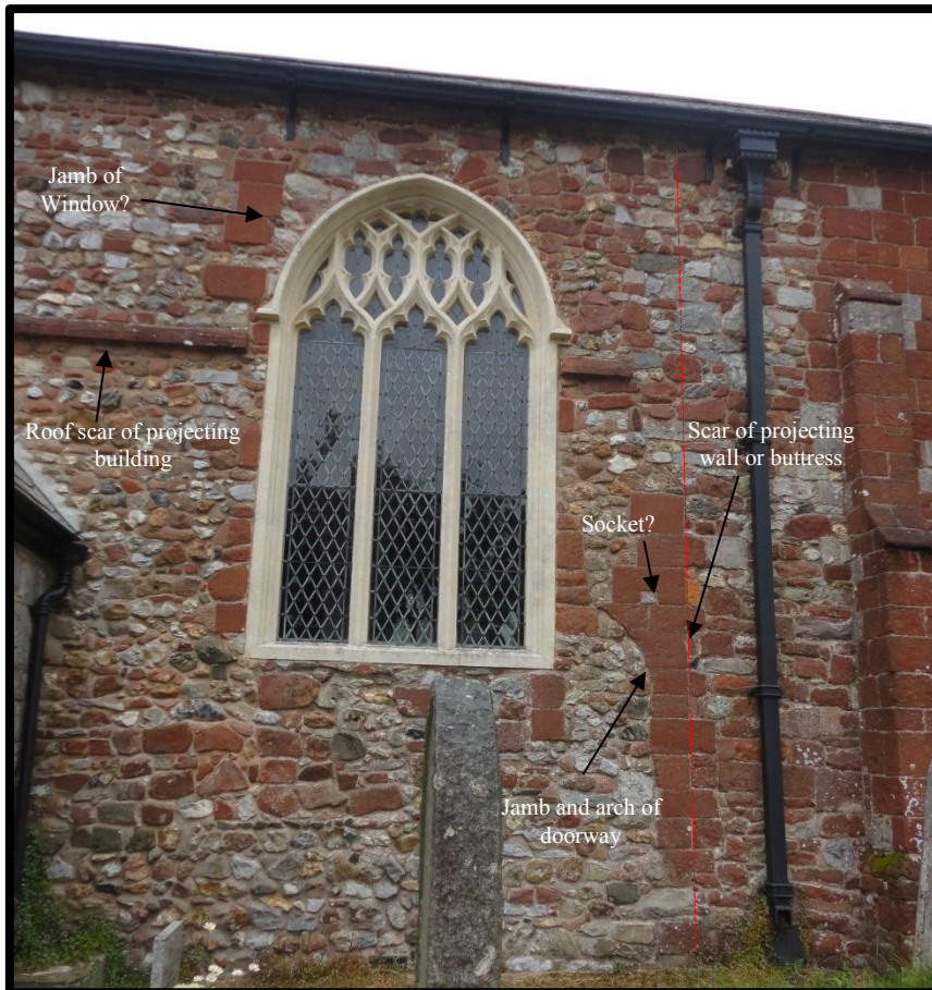
Fig. 4 Elevation of the west end of the south aisle showing features of possible early-medieval date cut by late medieval windows.
