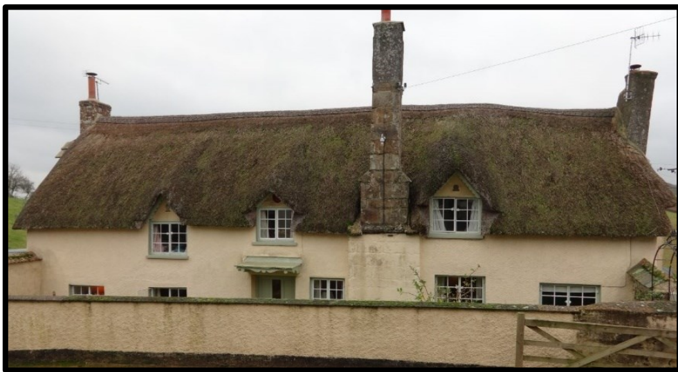
Fig. 3 General view of the farmhouse from the west, showing the façade with a lateral stack and floor levels descending to the north.
