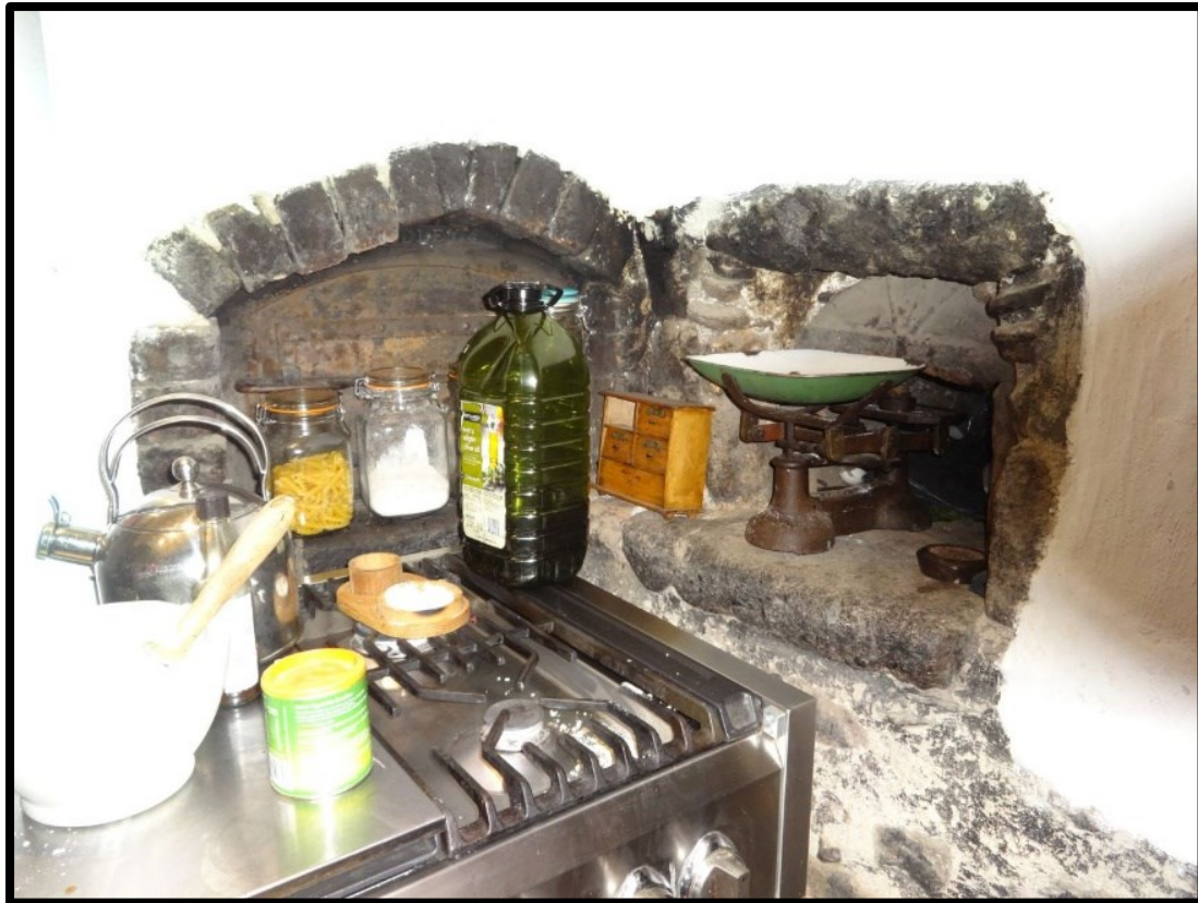
Fig. 8 View of the ovens in the south-eastern corner of the fireplace, showing a clay cloam oven built into a recess alongside a larger bread oven.
