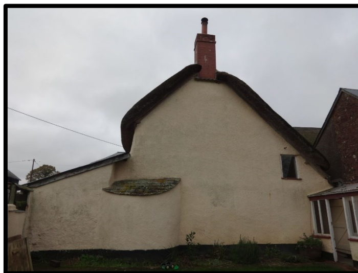
Fig. 4 General view of the farmhouse from the east, showing the projection for the oven. The whole elevation is effectively the chimney breast of the kitchen fireplace.
