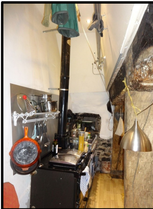
Fig. 6 View within the fireplace looking south, showing the very large space within the kitchen chimney which may have been employed as a smoking chamber.
