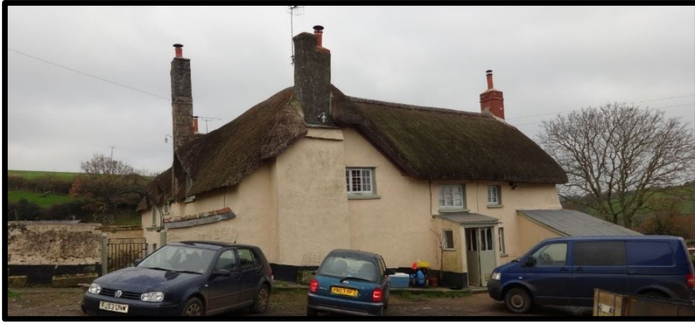
Fig. 2 General view of the farmhouse from the south, showing the 17th-century rear wing (right) attached to the rear of the main house.
