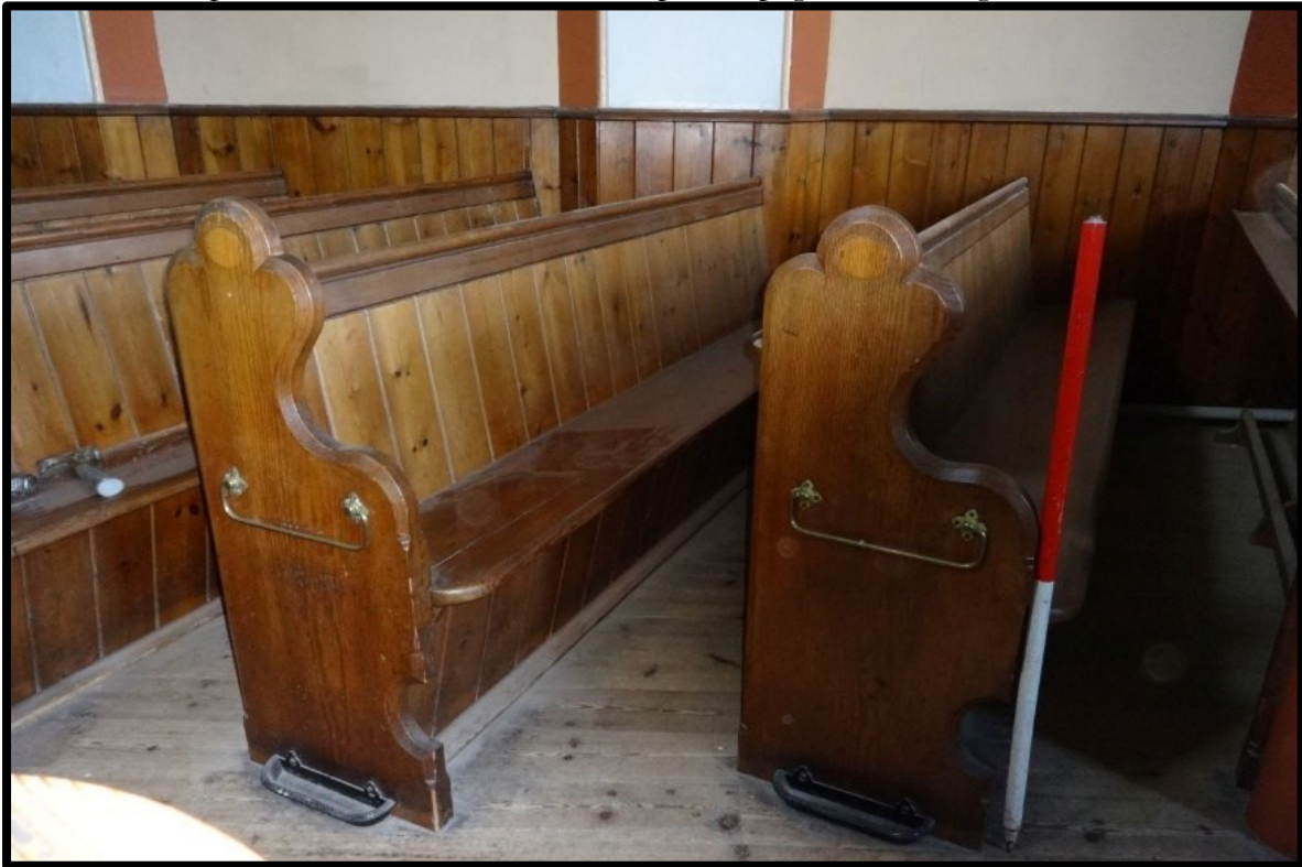
Fig. 16 Detail of the benches in the body of the chapel showing the shouldered ends, trefoil tops and the umbrella stands. Each bench incorporates a hat rest in the lower section.
