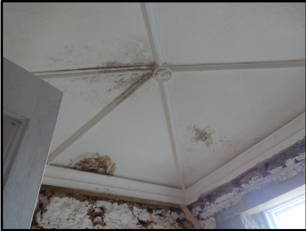
Fig. 25 Detail of the ceiling of the lower vestry showing simple Gothic motifs of ribs and a central boss.
