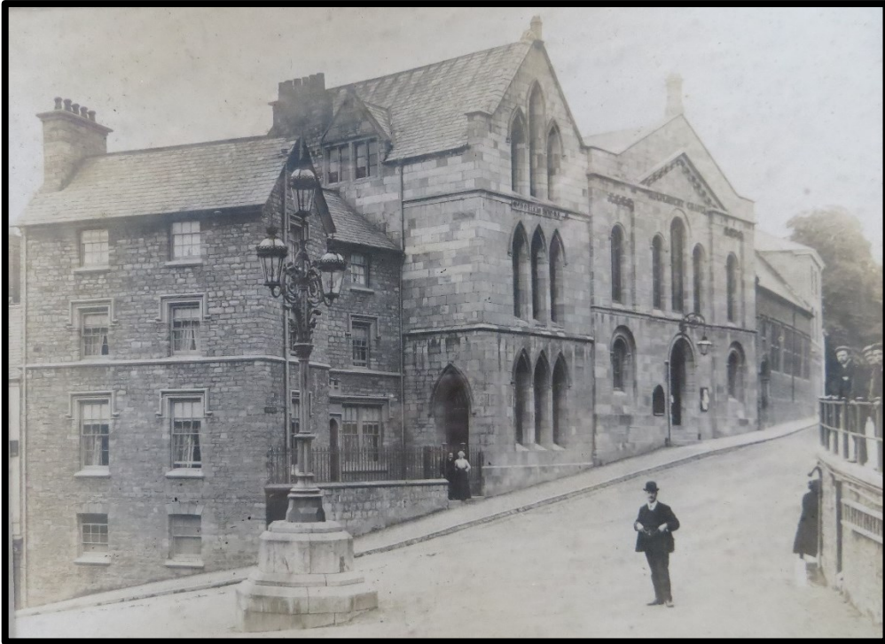
Fig. 9 Photograph of the buildings by E. McDonald, undated but probably c. 1900, Showing the buildings after the 19th-century alterations, including the 1860s addition of an upper storey to the Memorial Rooms (Sue Searle's collection).
