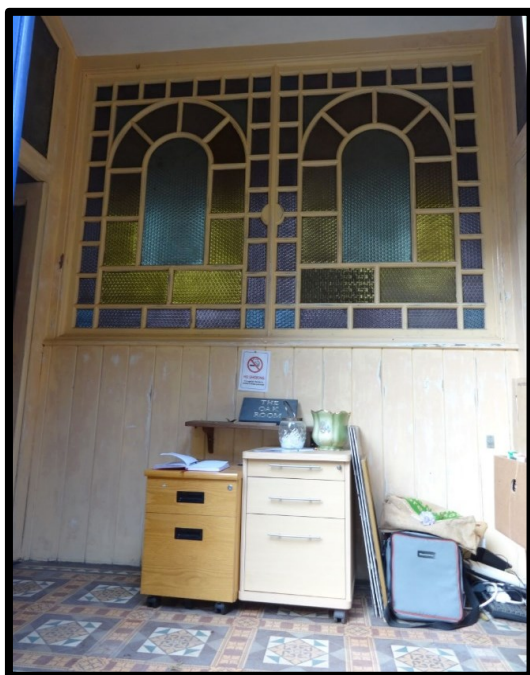
Fig. 12 View in the lobby showing the tinted rolled glass panels of 'diaper glass' and the tiled floors dating
