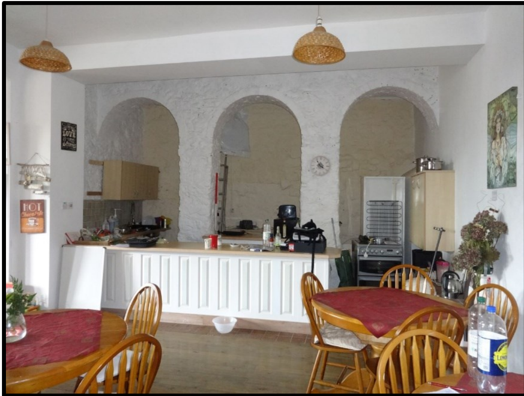
Fig. 27 View of the basement room looking north showing the arcade of three brick arches underlying the church. Similar arches exist within an inaccessible void on the south side.
