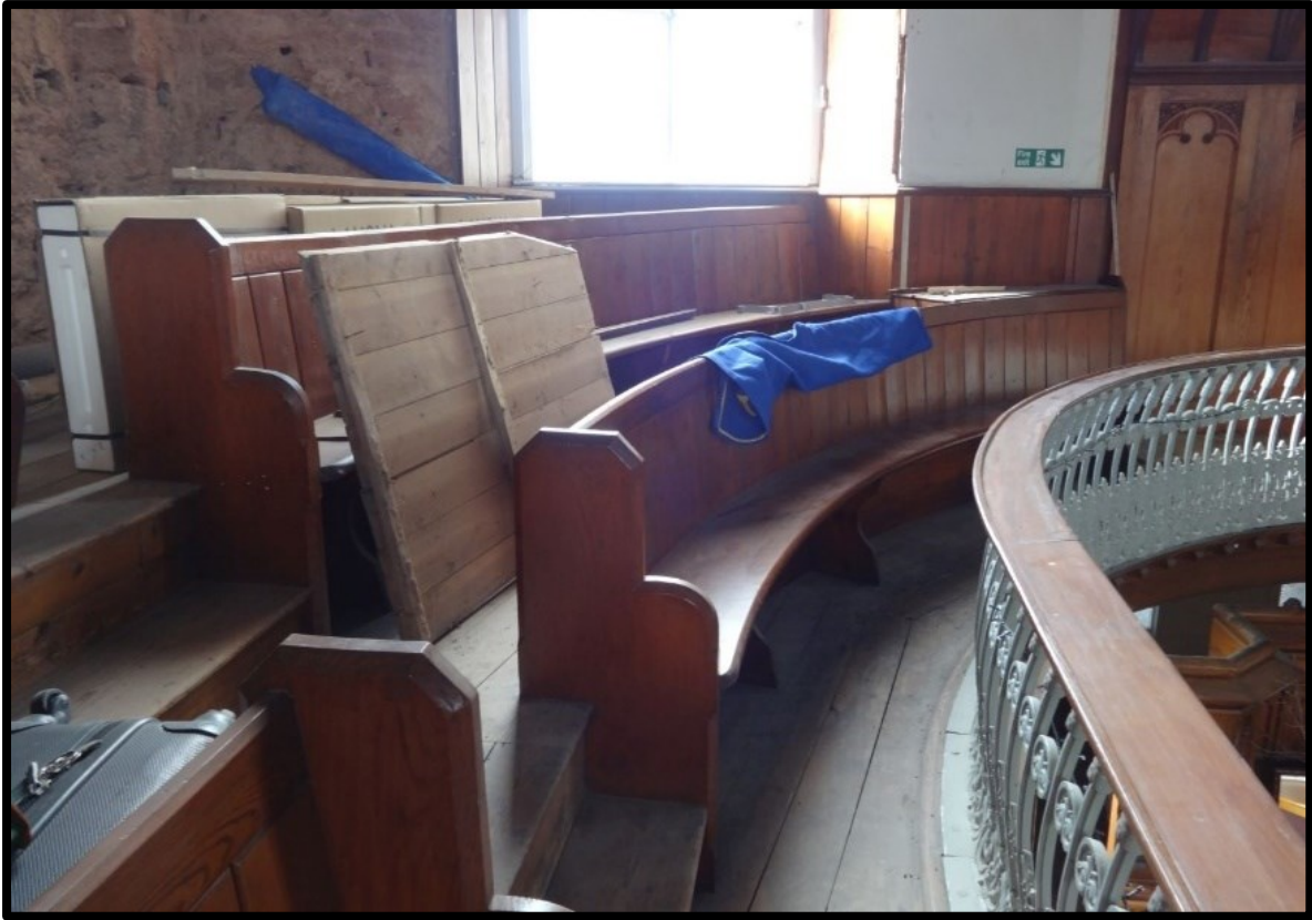
Fig. 17 Detail of the simpler form of benches in the curving part of the gallery. These have simpler profiles to the bench ends and may have been either free seats or choir seats, though they are not provided with suitable book rests for this purpose.
