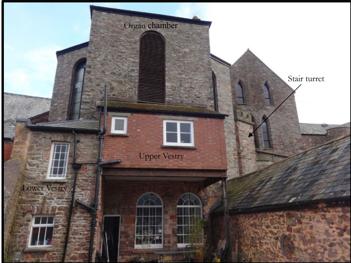
Fig. 11 Rear elevation of the chapel showing the two arched windows of the former Schoolroom, the small projection containing the Lower Vestry, the brick projection of the Upper Vestry and the polygonal apse with organ chamber above. Note the stair turret at the rear of the Memorial Rooms.
