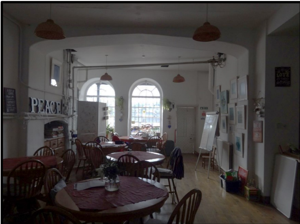
Fig. 26 View of the basement room looking west showing the shallow Gothic arch supporting the jambs of the apse and the windows and doorway to the yard.
