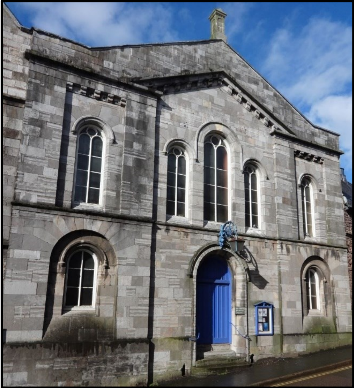
Fig. 10 The main elevation of the chapel from St Peter's Street. A discontinuity in the coursing of the plinth can be seen far right.
