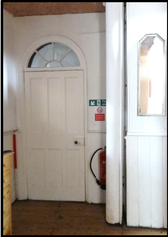
Fig. 23 The 1830s six panelled door with fanlight opening on the vestry stairs with the wind duct for the organ alongside.
