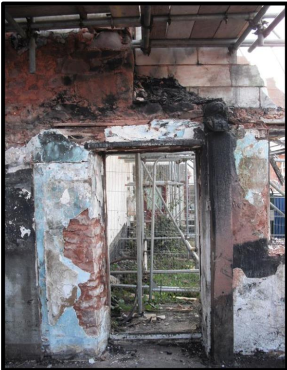
Fig. 20 The former front door of the No. 1, looking north west, showing the post and beam immediately adjacent to it.
