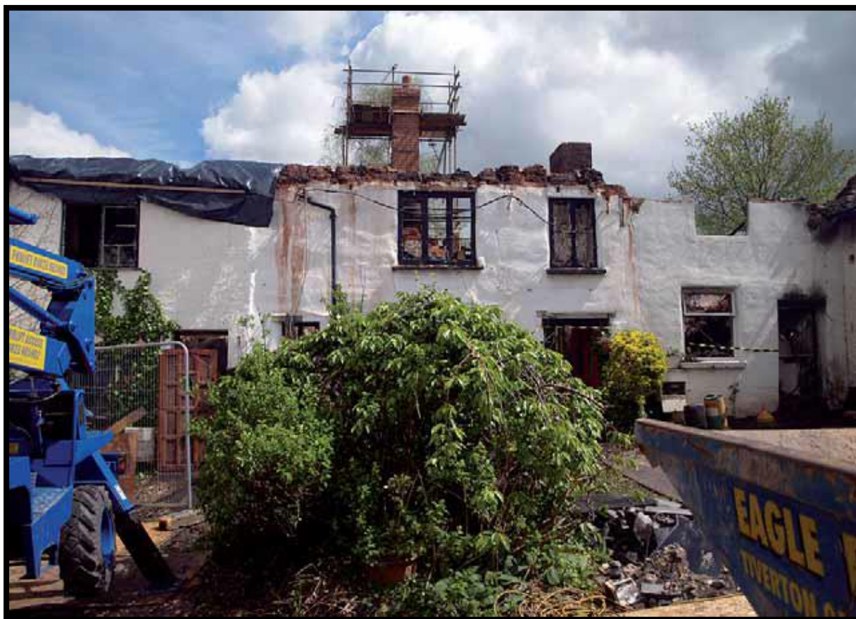
Fig. 17 Elevation of Nos 1-3 Buller square following the fire, but before demolition works, taken from the Keystone report (Keystone 2012 Report No. K823-1).
