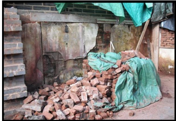
Fig. 28 The remains of the party wall with No.3 showing brick masonry, and the apparent vertical break (left) possibly allowing for a doorway.
