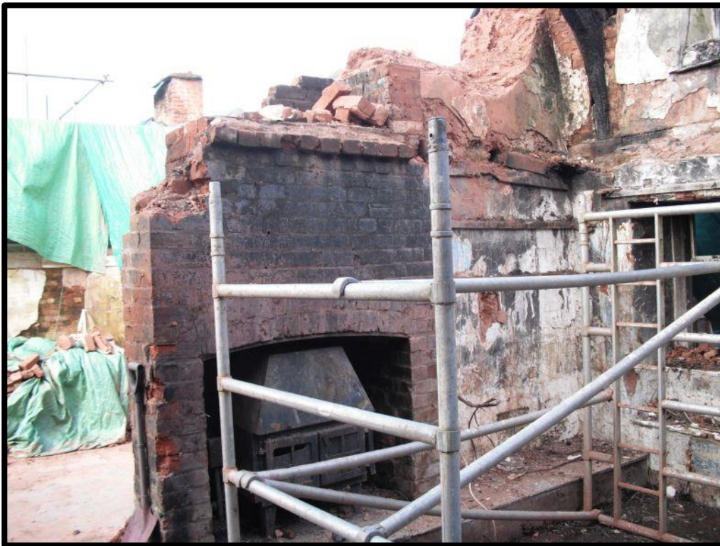
Fig. 24 View of the fireplace in the party wall between the two houses, showing the 19th-century brick fireplace cutting into the earlier cob walling and the remains of a second fireplace embrasure at first-floor level above.
