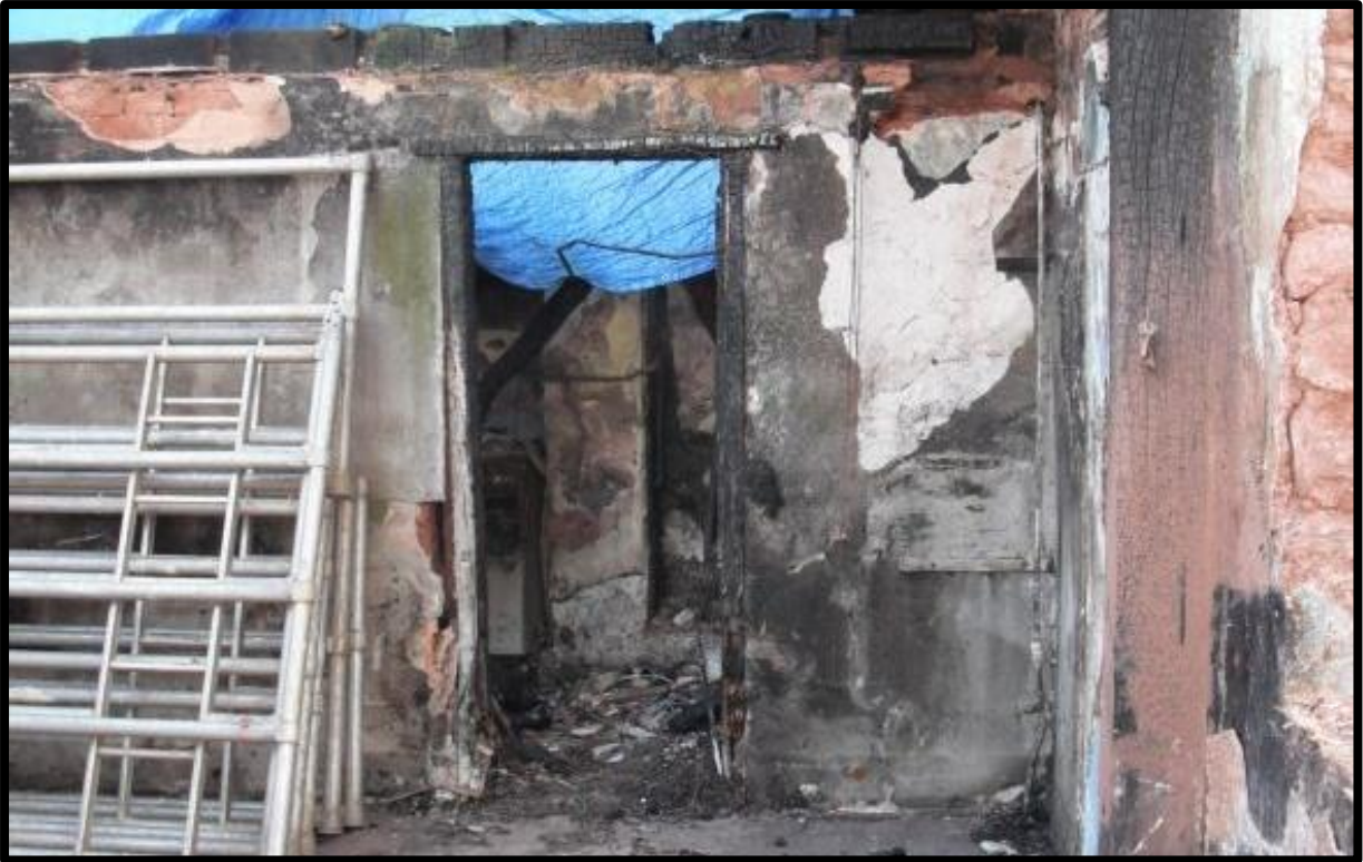
Fig. 31 Detail of the late partition defining the south-eastern room of No. 1 Buller Square.
