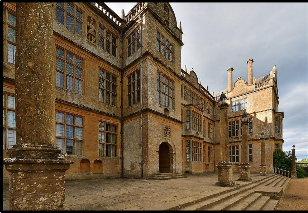
Fig. 16 Montacute, Somerset, an Elizabethan E- plan house with elevations employing both round- topped shell-headed niches and hemispherical roundels as architectural features
