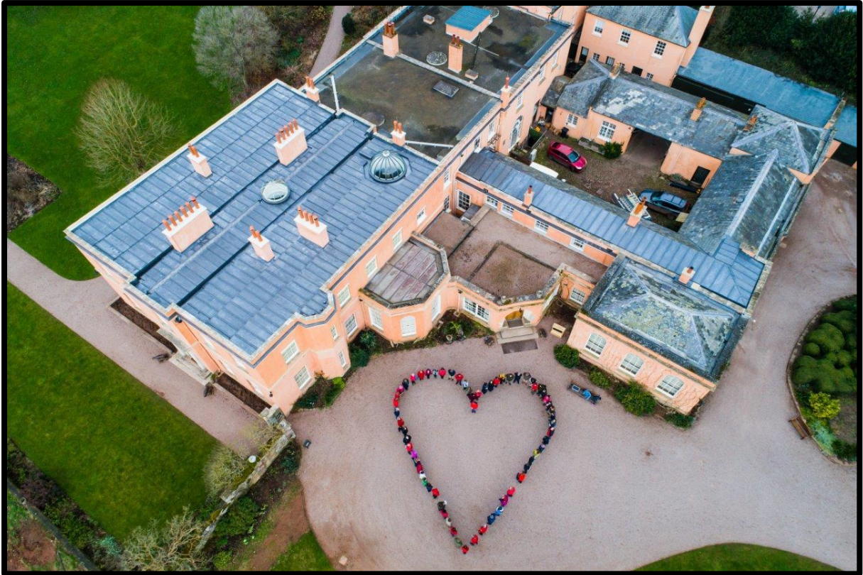
Fig. 19 Aerial view of the new roof structures at Killerton House in 2019 (possibly by Malcolm Jarvis for PCA Consulting engineers and the National Trust), showing the new lead flats, rebuilt chimneys and domes, and expressing the fond hope of Killerton staff and volunteers that this solution will endure for a little longer than its predecessors.
