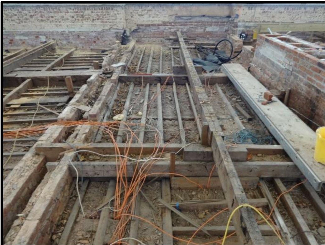
Fig. 26 The ceilings over the central spine corridor, showing the south end, with the chimney of the present library to the right. The ridge timber shown over the corridor, centre right, appears to relate to the 19th-century roof.
