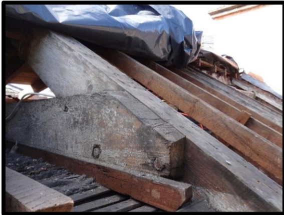
Fig. 39 The end of one of the collars showing the method of securing with large metal spikes.
