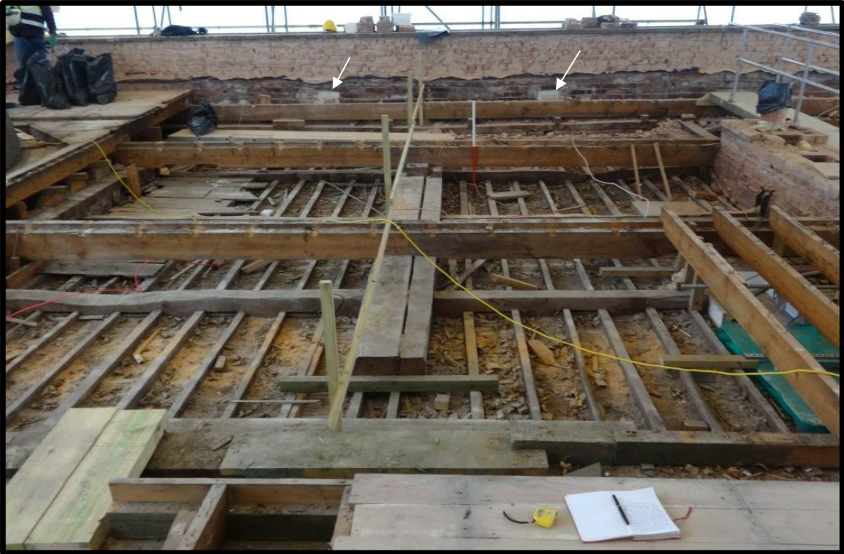
Fig. 21 The northern part of the eastern roof showing blocked sockets in the parapet wall answering to the open sockets visible in the west wall (see below). These sockets are unrelated to the flat or double-pitched roof structures and must surely have housed tie beams for an earlier phase of roofing.
