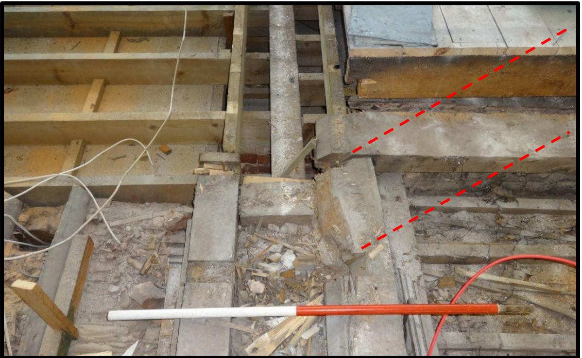
Fig. 22 Angled housings in the beams over the eastern spine wall of the first-floor corridor showing the position of the rafters of a shallow pitched roof over the east part of the house - probably a different phase from the large blocked sockets above.
