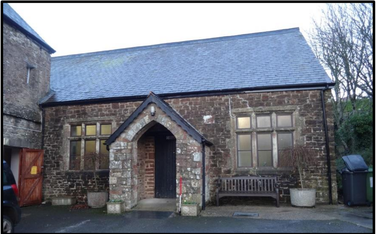
Fig. 30 Detail of the south façade of the early 20th century parish hall.
