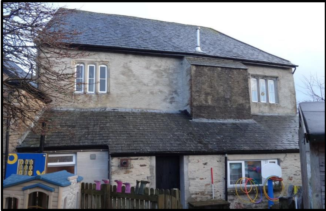
Fig. 19 West elevation of the west range showing the two three-light windows at first-floor level and the large chimney breast serving the fireplaces at ground- and first-floor level. The lean-to probably dates from the 19th century.
