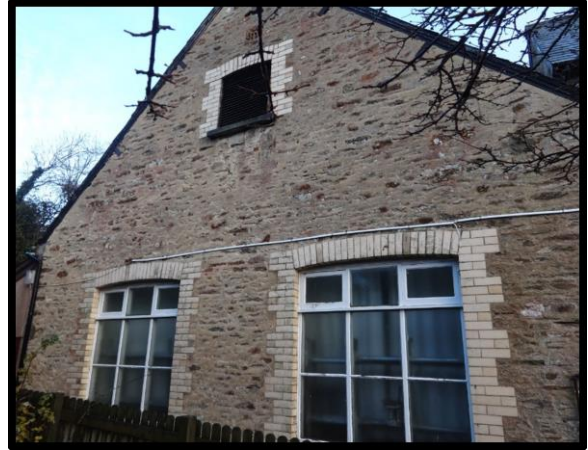
Fig. 32 View of the western gable of the hall, showing white brick dressings, and (top centre) a reused carved stone.
