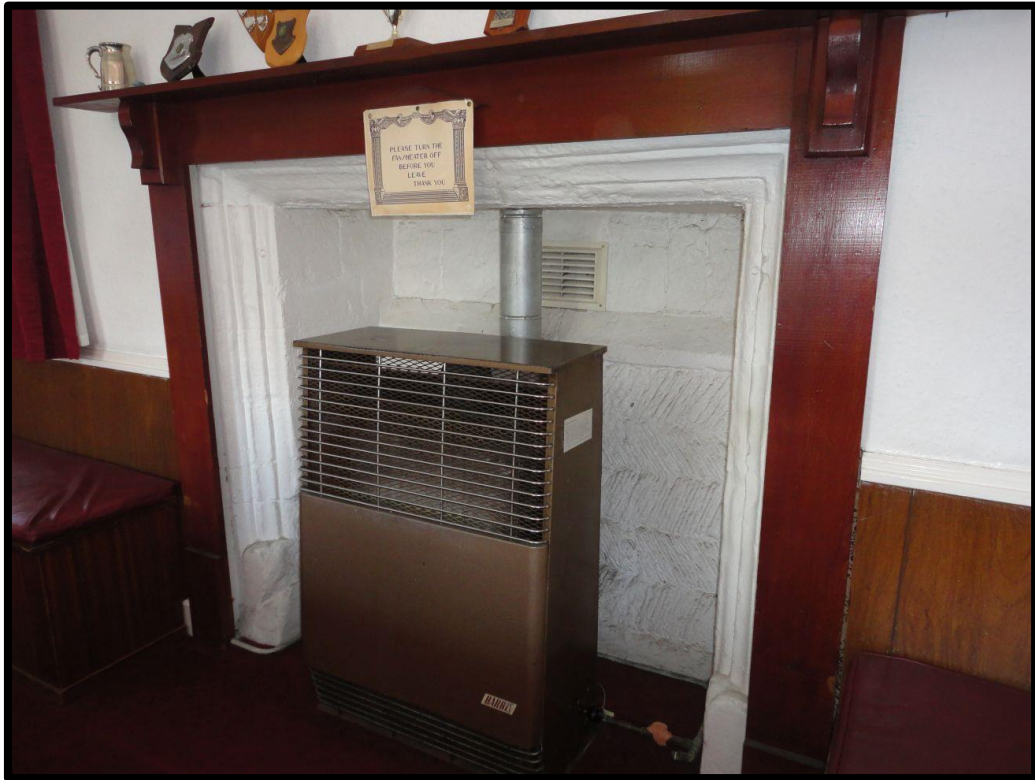
Fig. 25 View of the fireplace in the west wall of the Billiard Room, featuring a moulded and stopped stone frame partially concealed by a 20th-century timber mantelpiece.
