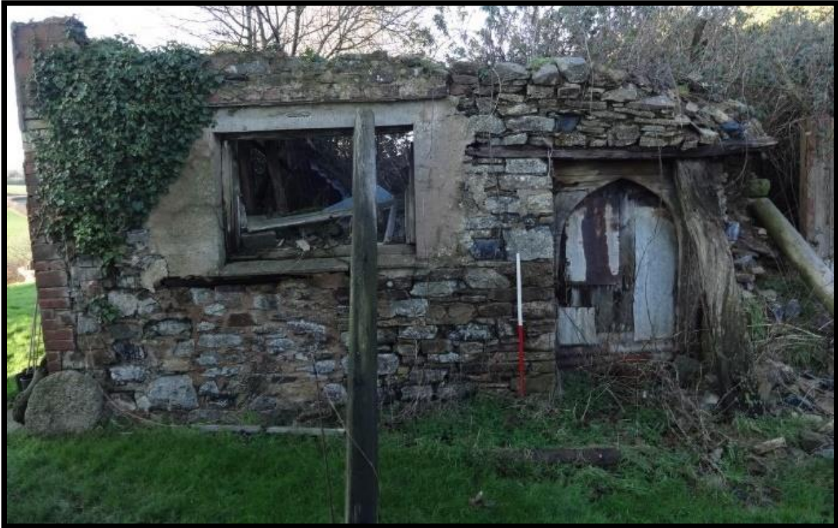
Fig. 33 The remains of the ruined building to the north of the house, showing a 14th- or 15th-century arched timber doorway. Compare with Figs. 2, 34 and 35.
