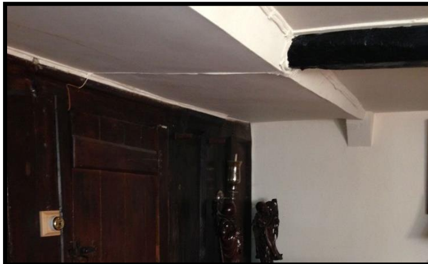
Fig 23 Detail of the hall screen, showing the pronounced internal jetty towards the hall formed by the joists of the chamber floor projecting over the earlier screen and the junction with the later beam supporting the hall chamber floor.
