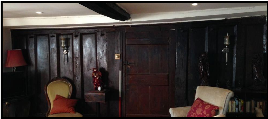
Fig 22 Elevation towards the hall of the hall screen, showing the position of the central doorway and the absence of provision for the staircase, right, suggesting that the screen predates the addition of the chamber over the entry.
