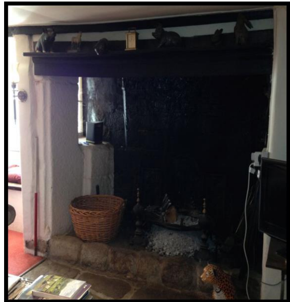
Fig. 29 Detail of the fireplace in the hall, showing the granite jambs pierced by a later window. The lintel, also of granite, rises well above the ceiling, which is supported by a trimmer against the lintel.
