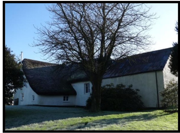
Fig. 14 The rear of the house showing the blank wall of the shippon (right) the stair window marking the position of the cross passage (centre) and the rear wing and outshut (left).
