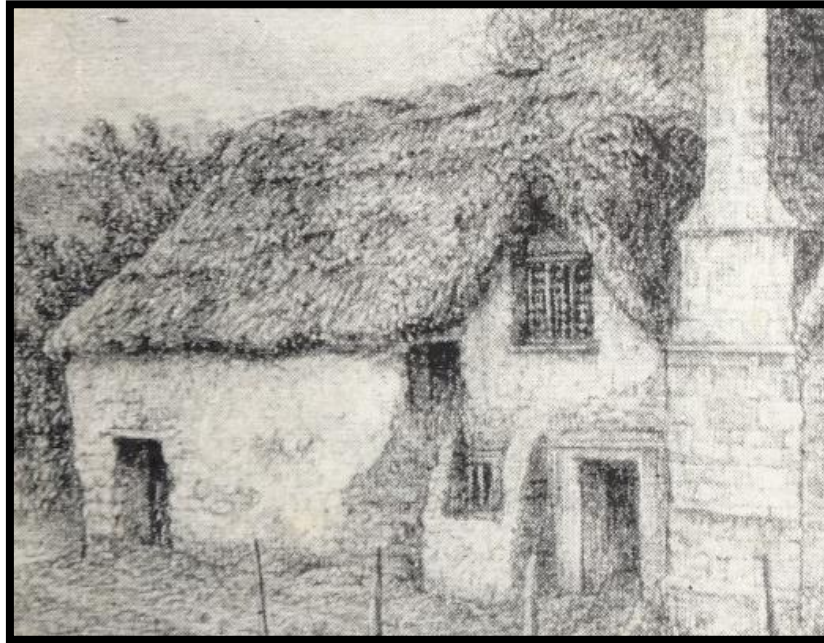
Fig. 20 Detail of Lega-Weekes' drawing of the shippon in 1902, showing the early openings in the south-eastern wall and other features now removed.
