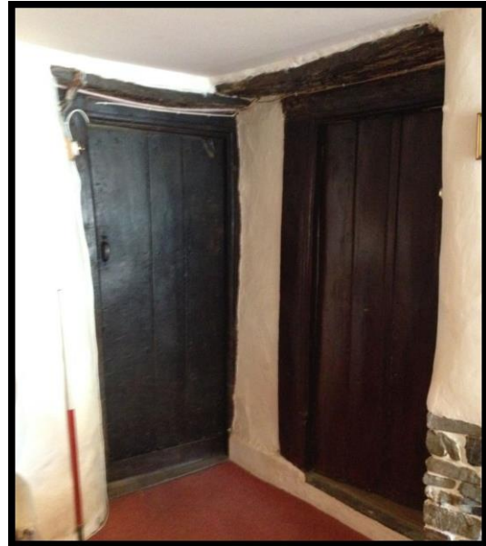
Fig. 31 Doors from the hall to the rear wing and inner room, decorated with ovolo mouldings and scroll and bar stops.
