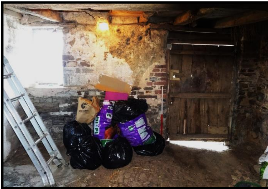
Fig. 19 The interior of the shippon, looking south-east, showing the surviving parts of the cobbled floor and the cob and later brick rebuilding of the front wall supporting the joists of the loft floor.
