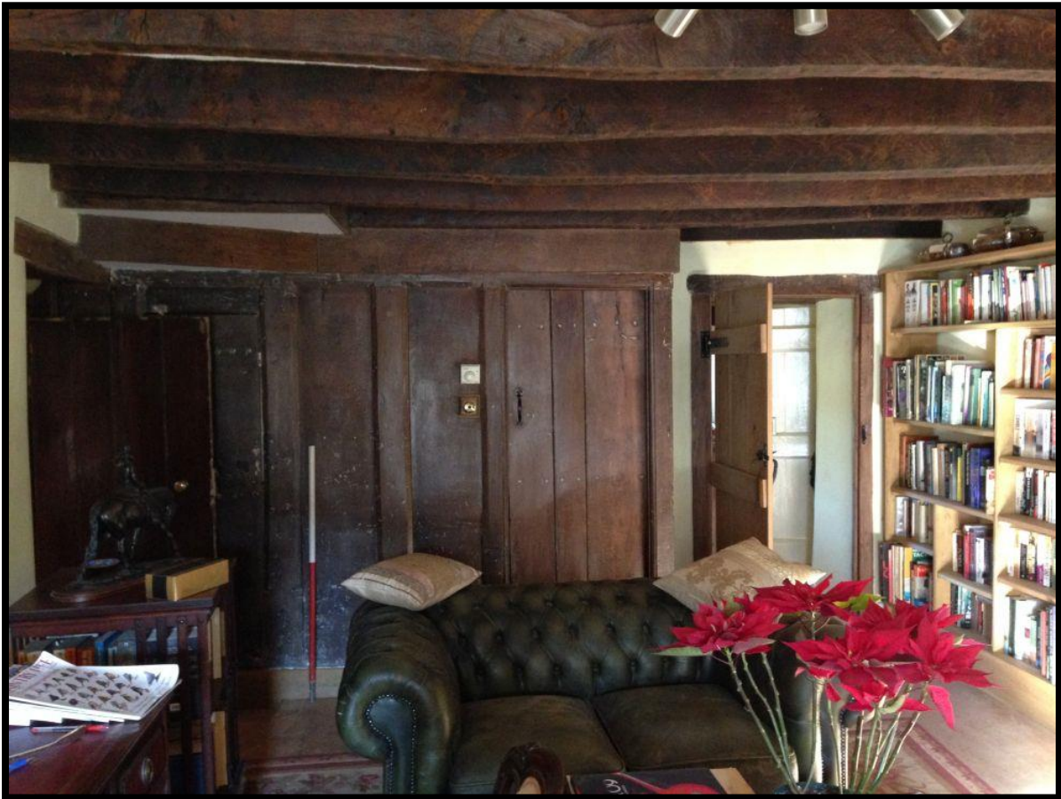
Fig. 32 The inner room from the south-east, showing the 17th-century plank and muntin screens hiding the staircase cut within its north-western wall and the joists of the ceiling reset in 1983.
