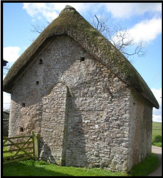
Fig. 34 View of the medieval detached chapel at Bury Barton, Lapford, showing the high eaves and small window openings, including an elaborate traceried east window behind the buttress.
