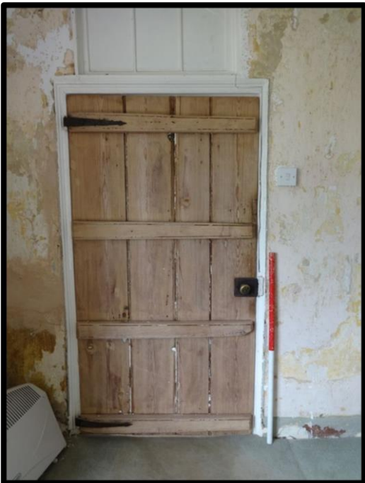
Fig. 10 The plank door to the south-west of the 'kitchen', possibly dating from the 18th century.
