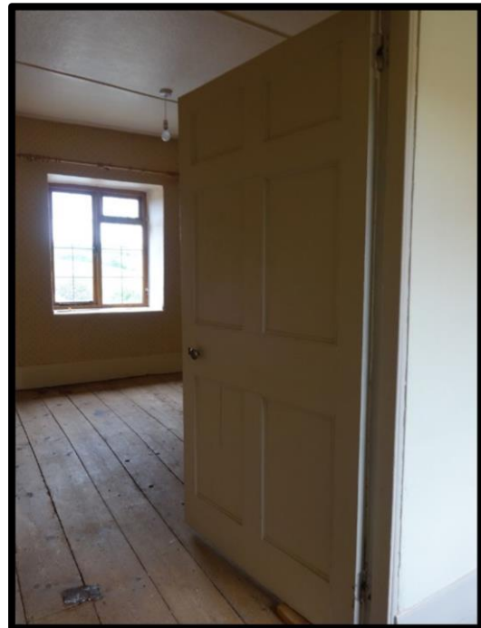
Fig. 15 A fine late 18th- or early 19th-century door leading into the south-western room at first-floor level.
