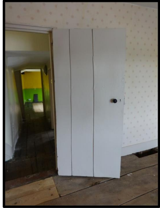
Fig. 17 A fine late 17th- or early 18th-century plank door leading into the north-eastern room at first-floor level, showing wide floorboards of elm.
