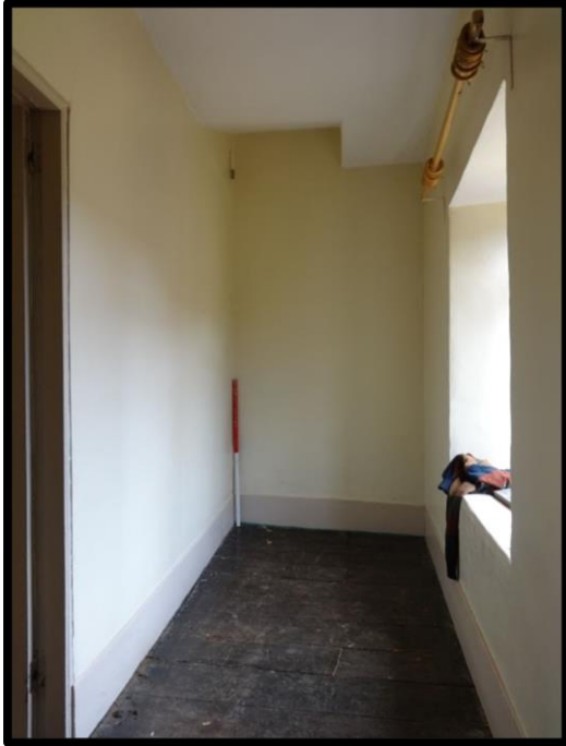
Fig. 16 The site of the corridor to the main house, showing the recess for the stairs in the ceiling: the site of the proposed new bathroom.
