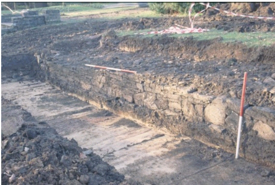
Plate 23 The ha-ha showing initial depth of excavation looking south west
