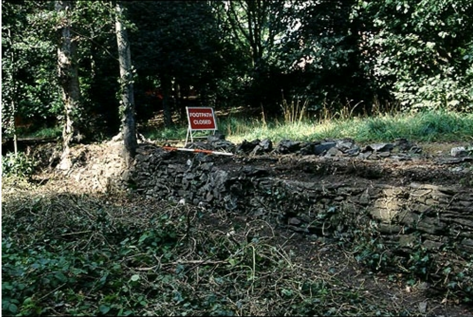
Plate 10 HHP 4.23 Wall No. 3 (east of steps)
