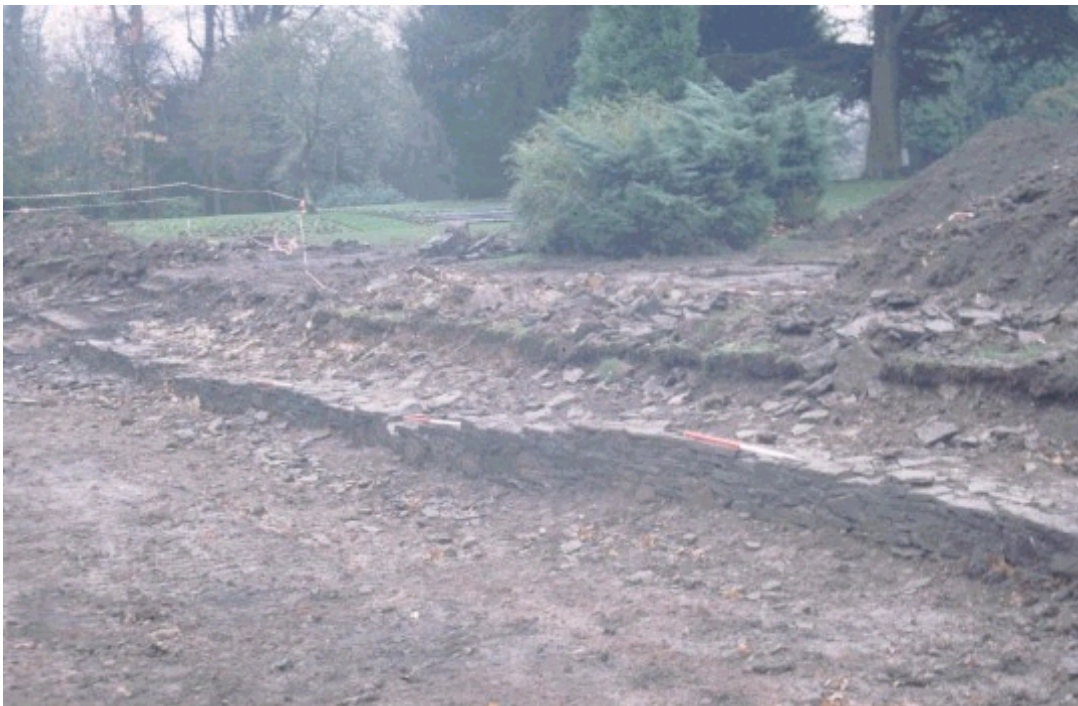
Plate 22 North end of the ha-ha looking south west
