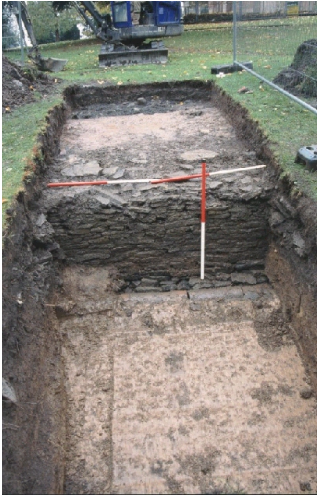
Plate 19 Trench 2 of the evaluation of the ha-ha, looking west
