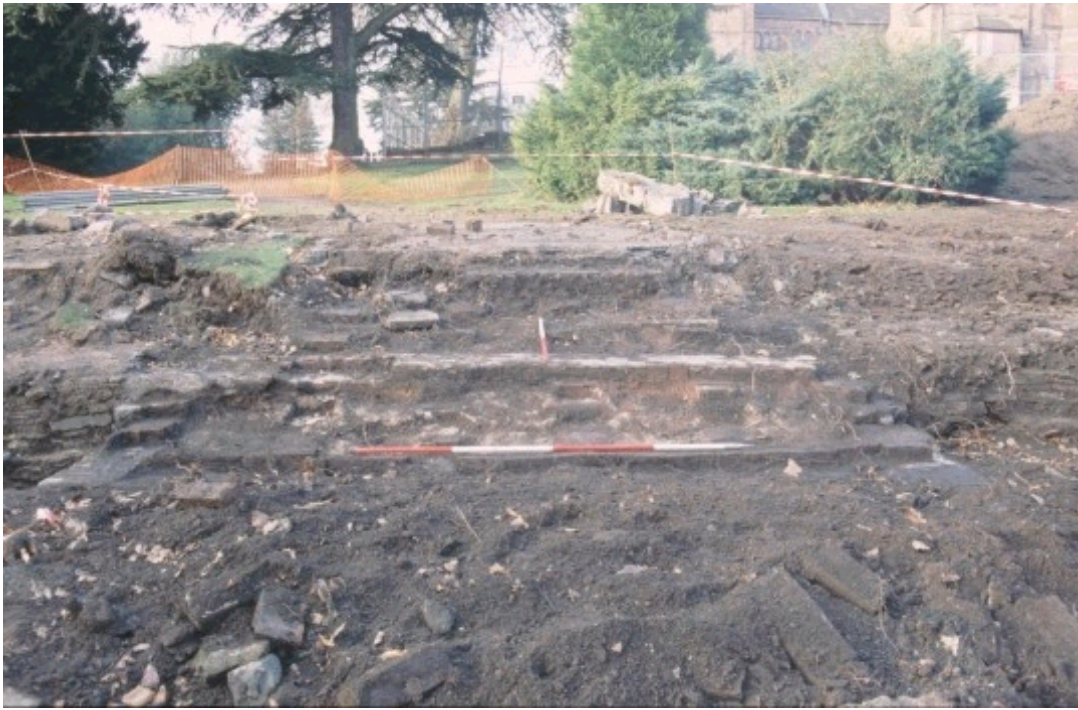
Plate 26 The foundation utilised by the existing steps, looking west
