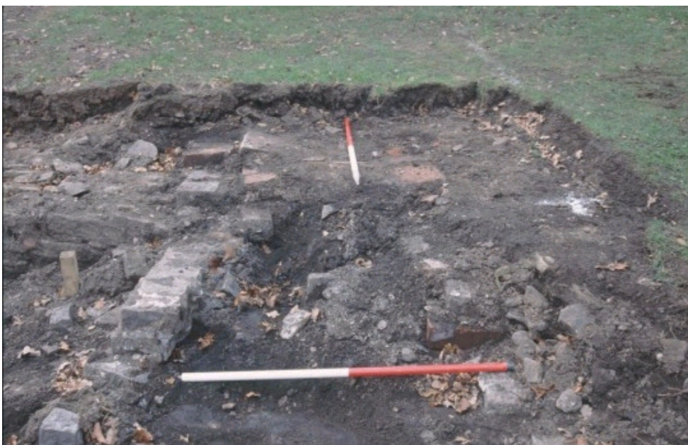
Plate 25 The missing north steps, looking west
