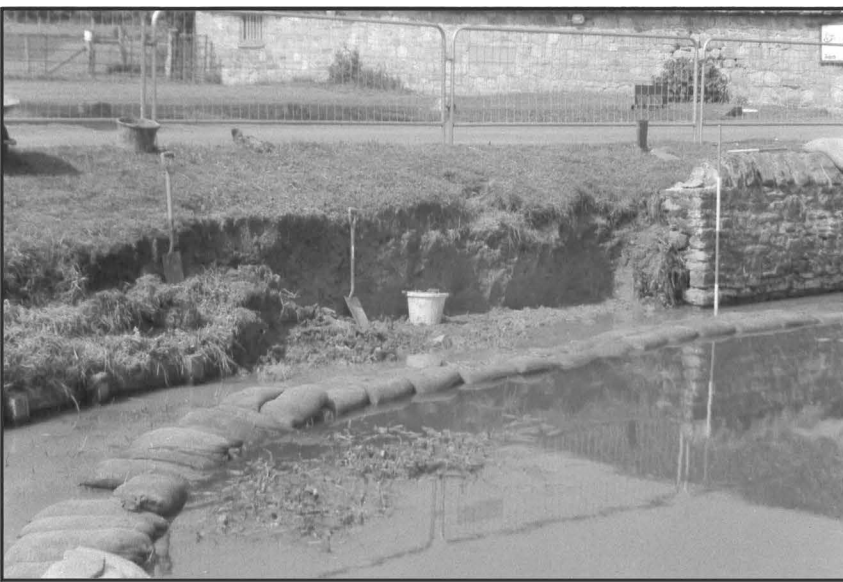
Plate 3: Digging foundation trench for new revetment wall
