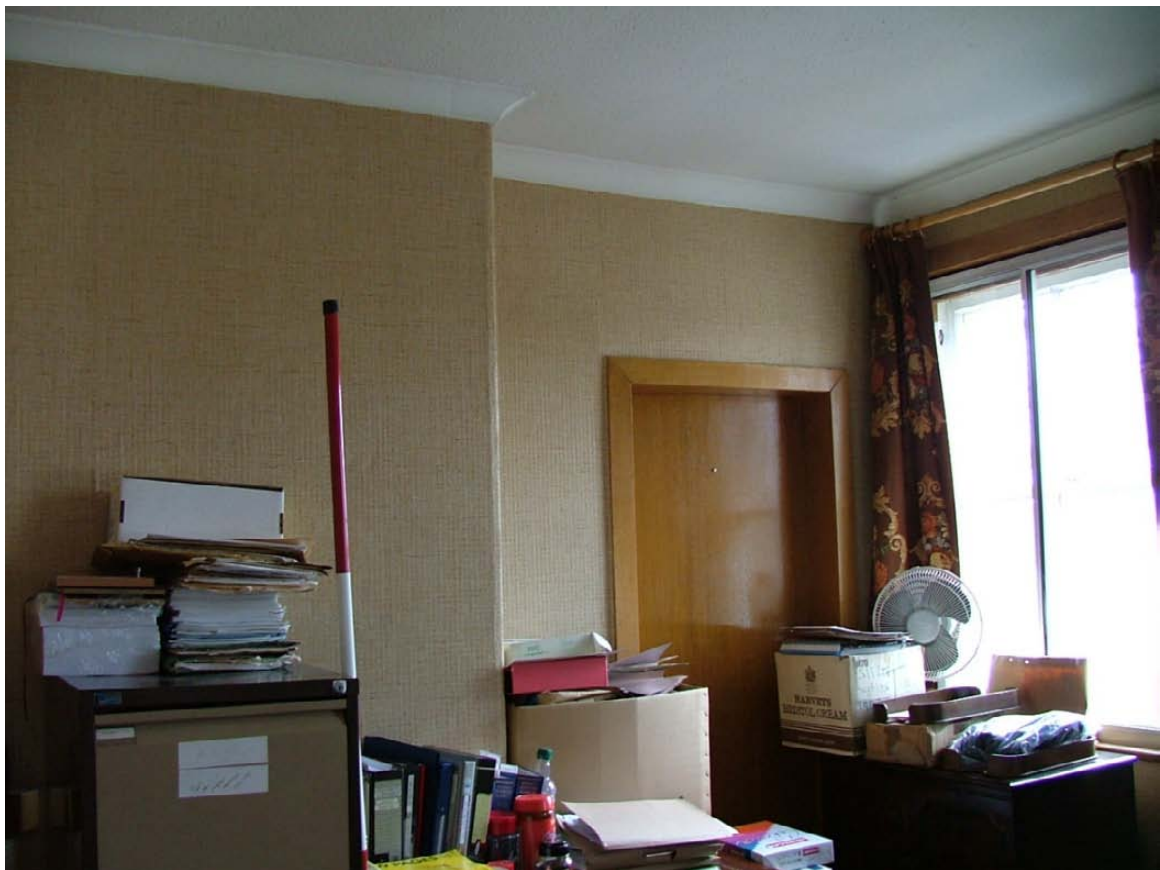
Plate 12: Representative shot of an office room, first floor
