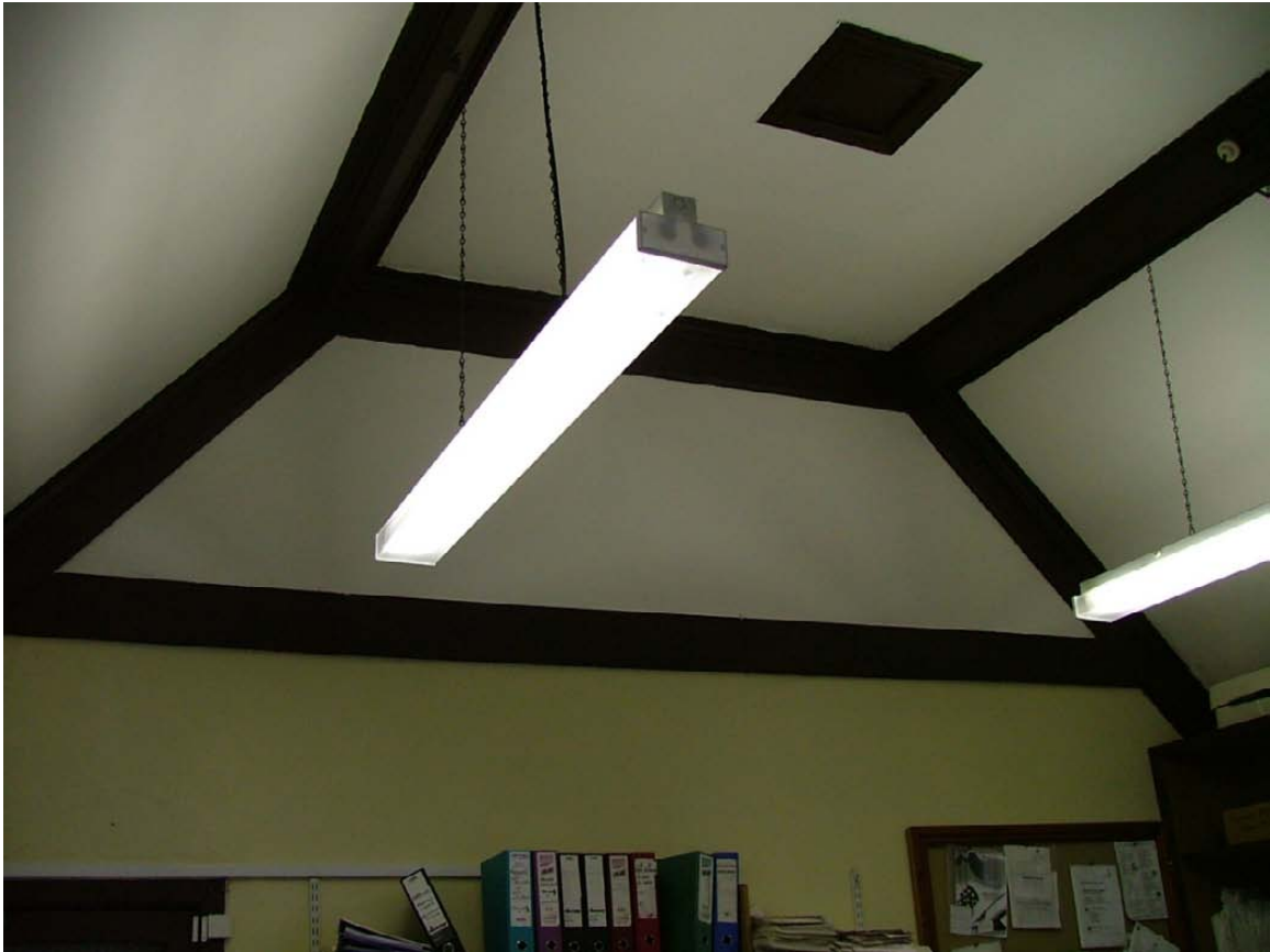
Plate 15: 19th century roof trusses, east cross wing, viewed from Securities office
