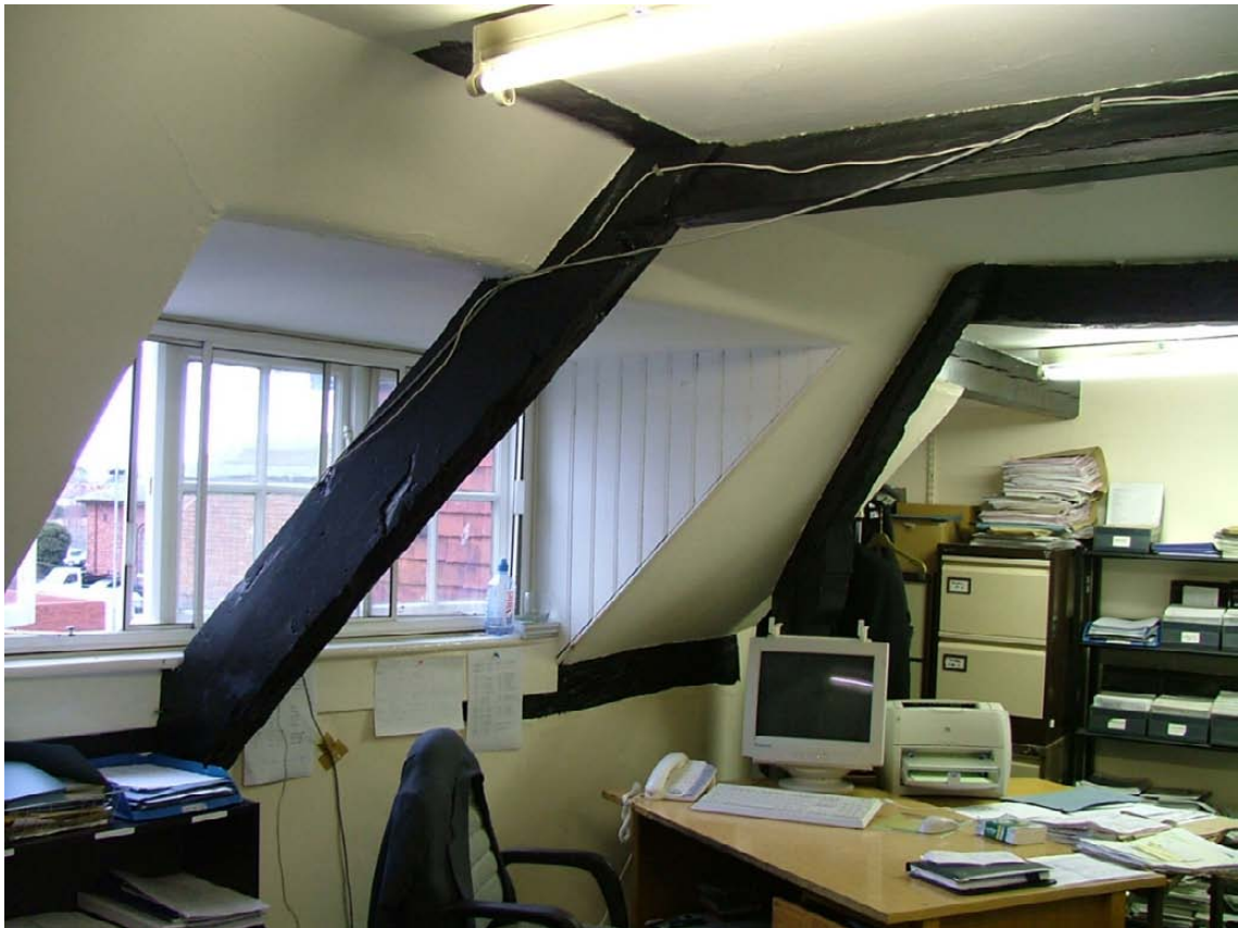
Plate 16: Exposed roof timbers in north attic office
