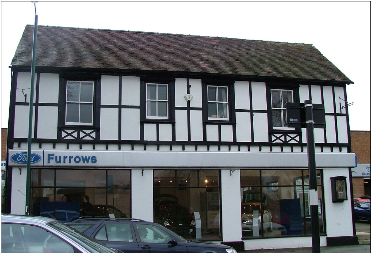
Plate 5: West elevation of Furrows Garage
