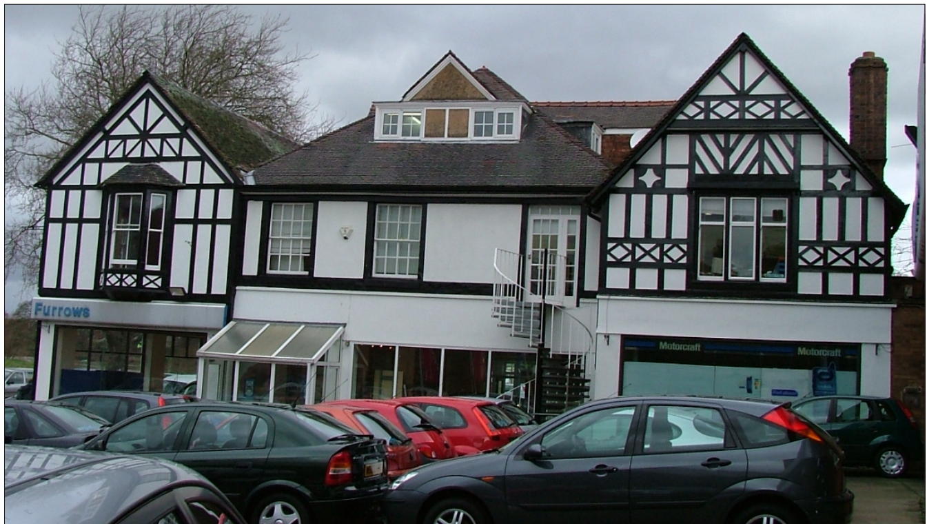
Plate 6: South elevation of Furrows Garage
