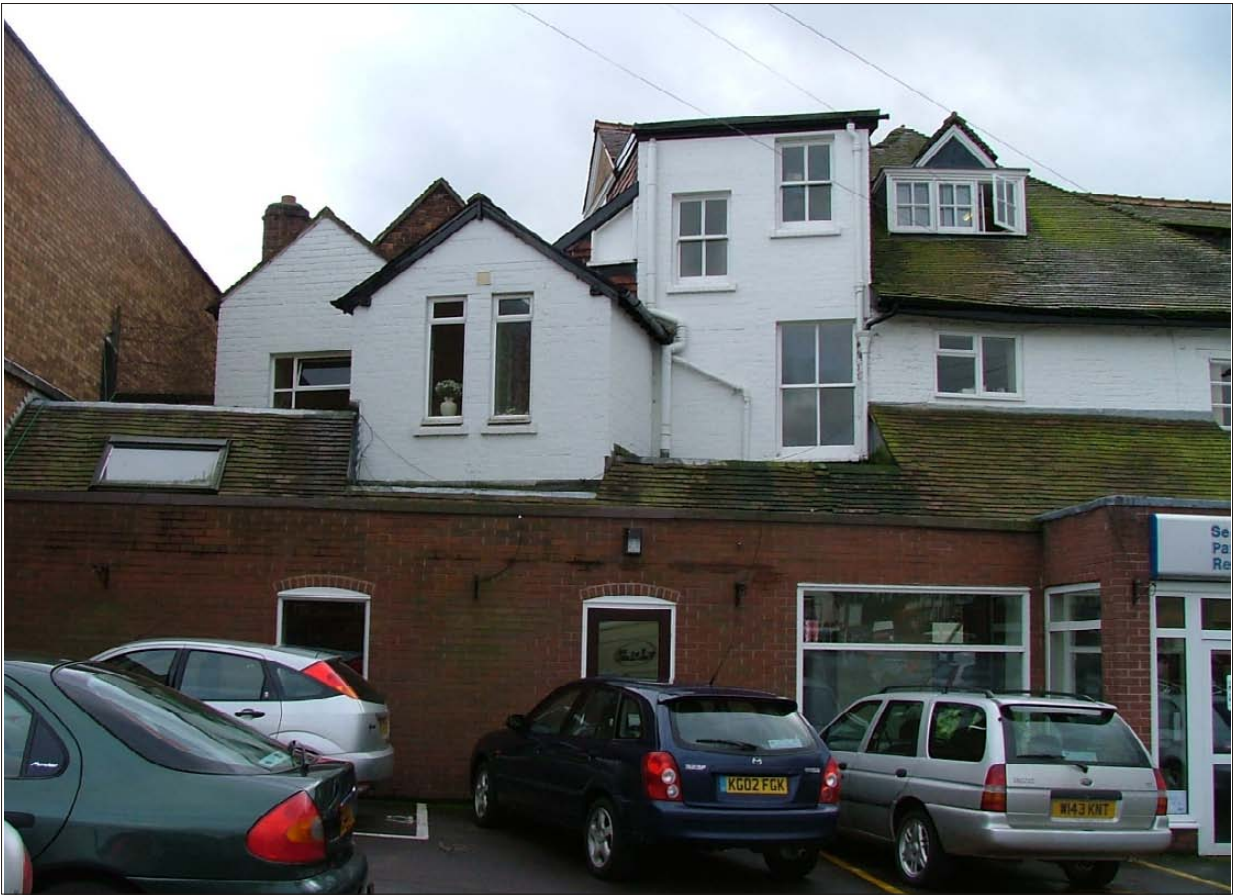
Plate 7: North elevation of Furrows Garage, east end
