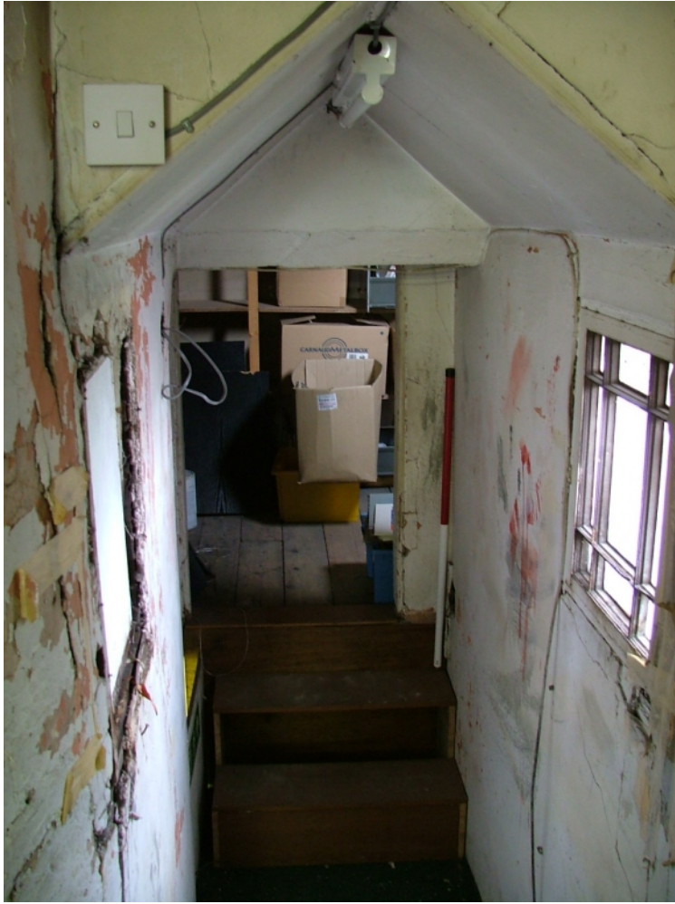
Plate 19: Passageway linking attic offices to attic of west cross-wing
