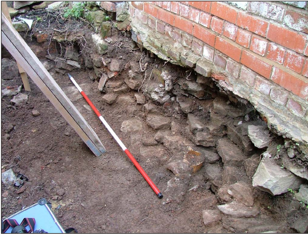
Plate 3: Exposed rubble core of Post-medieval wall
