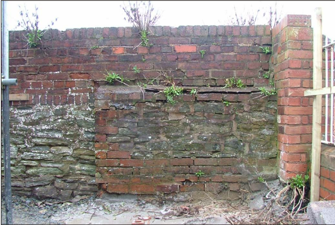
Plate 1: West face of boundary wall at south end
