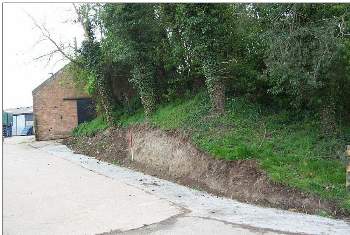
Plate 4 View of the motte facing south (Barn two is visible in the background)
