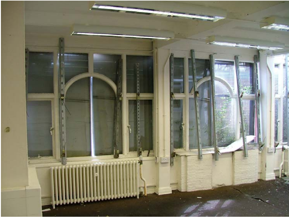
Plate 41: Windows in south wall of Room 7
