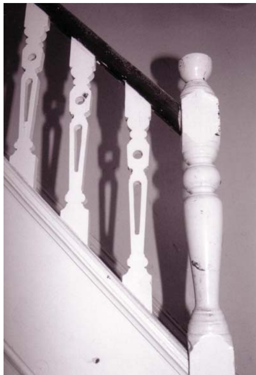
Plate 68: Detail of balustrade in corridor 24
