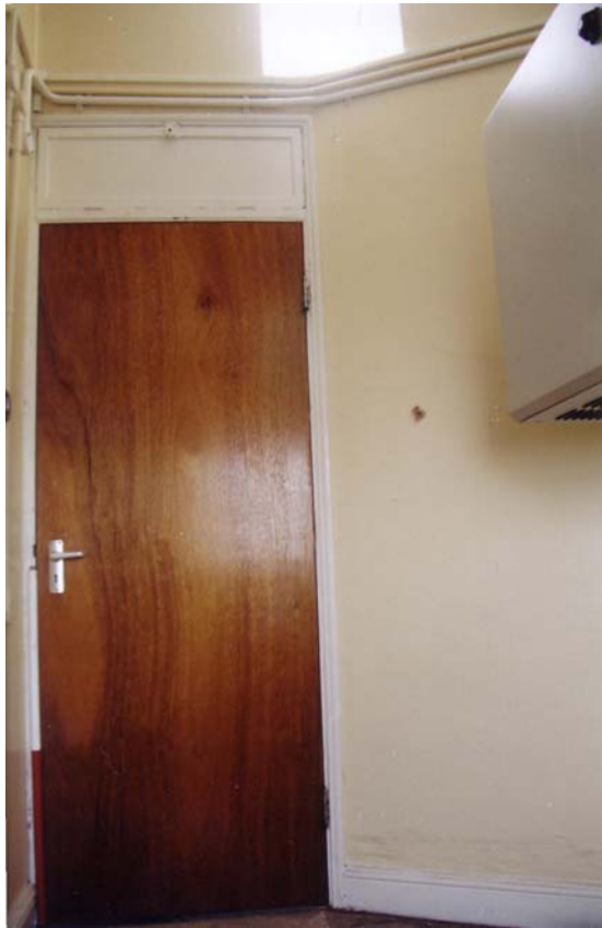
Plate 95: Room 42 from north
