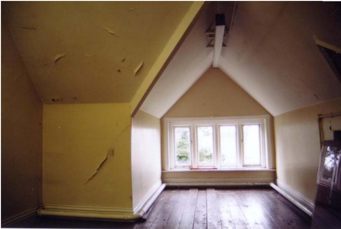
Plate 103: Room 44 looking west
