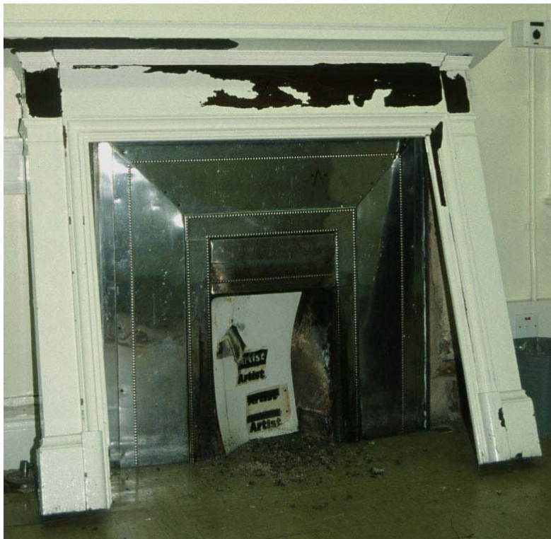
Plate 82: Fireplace in Room 35
