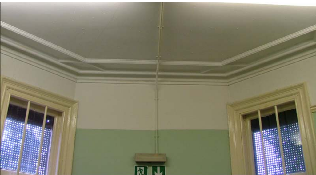
Plate 24: Pattern of cornicing in Room 2
