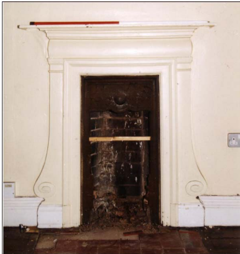
Plate 106: Fireplace in Room 45
