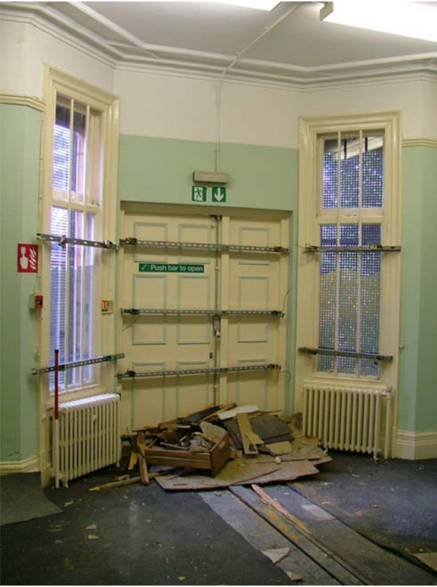
Plate 23: West entrance into Room 2
