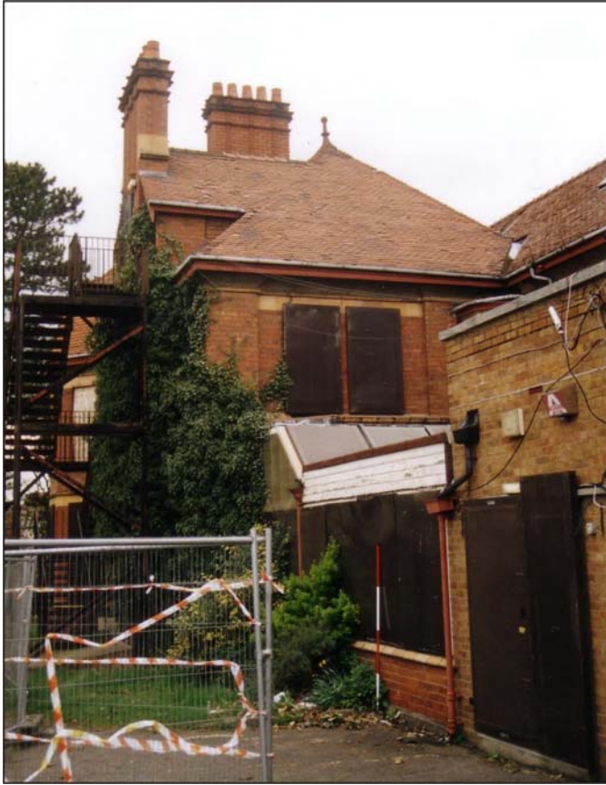
Plate 4: Southern east-west range of house from the south-east.
