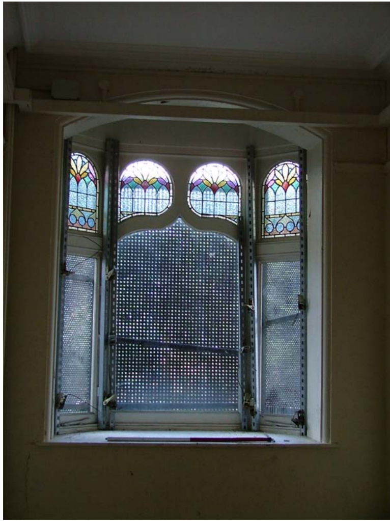
Plate 28: Oriel window in north wall of corridor 4a
