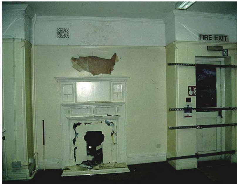
Plate 86: Room 37 from north
