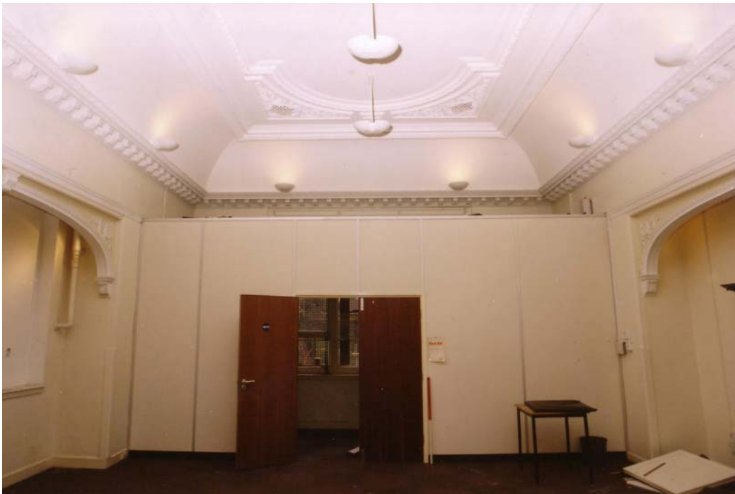
Plate 57: Room 22 from north
