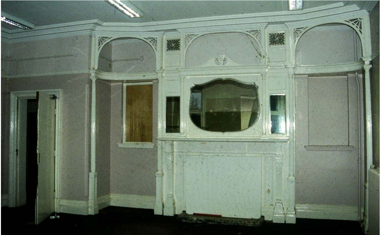
Plate 15: Fireplace and chimney-piece on east wall of Room 1
