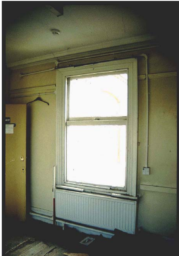
Plate 69: Room 25 from east
