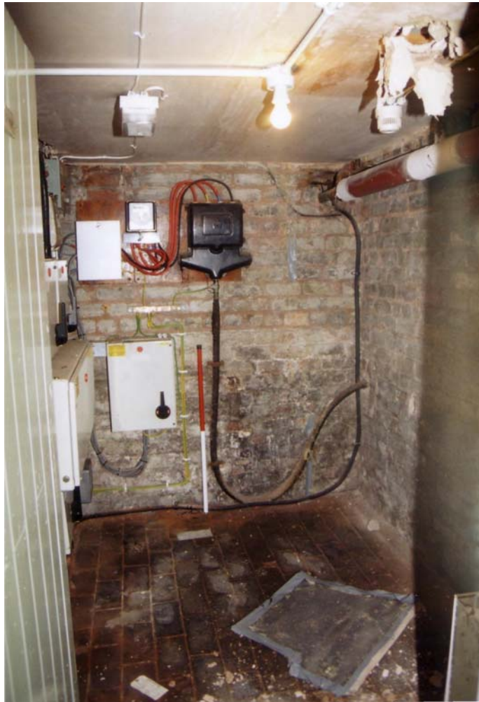
Plate 111: Room 48 looking east
