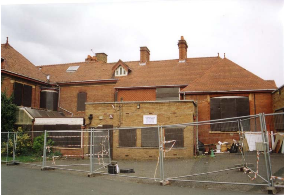
Plate 1: Rear bays of house from the south
