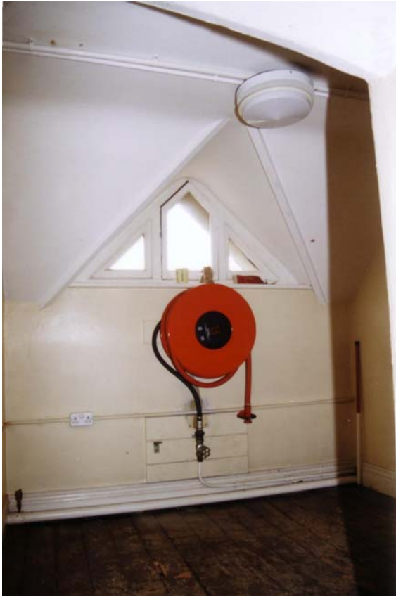
Plate 100: Triangular dormer in corridor 43b
