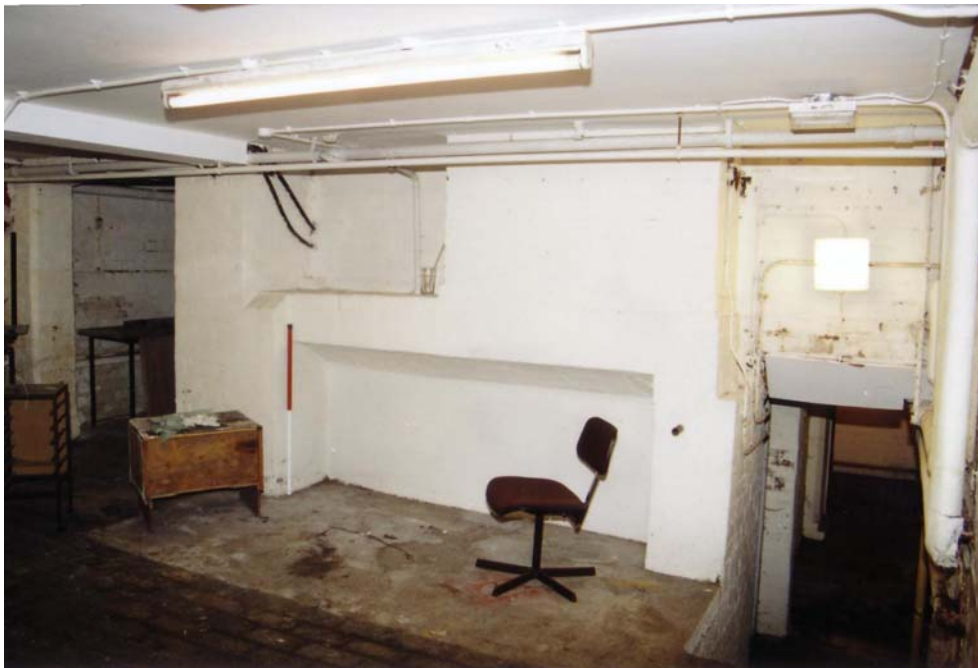
Plate 112: Room 51 looking west
