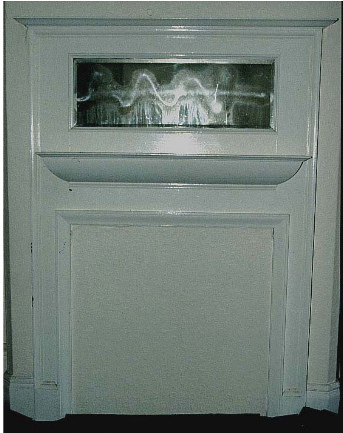
Plate 64: Fireplace in Room 22
