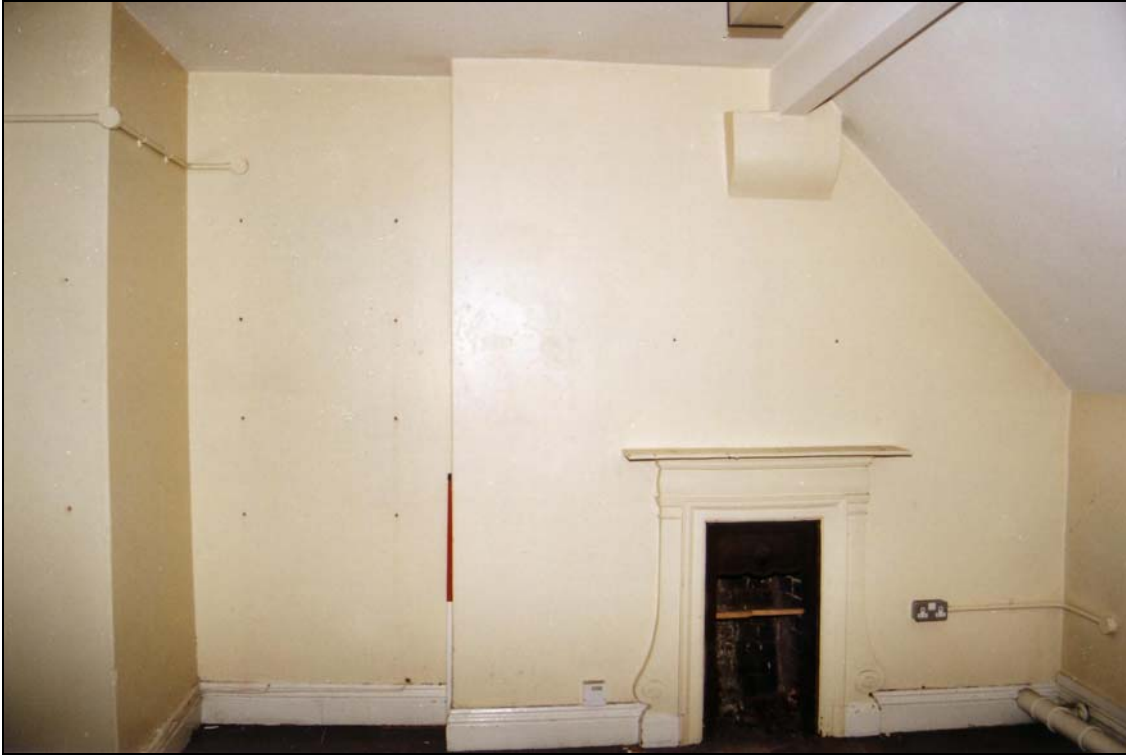
Plate 105: Room 45 looking east
