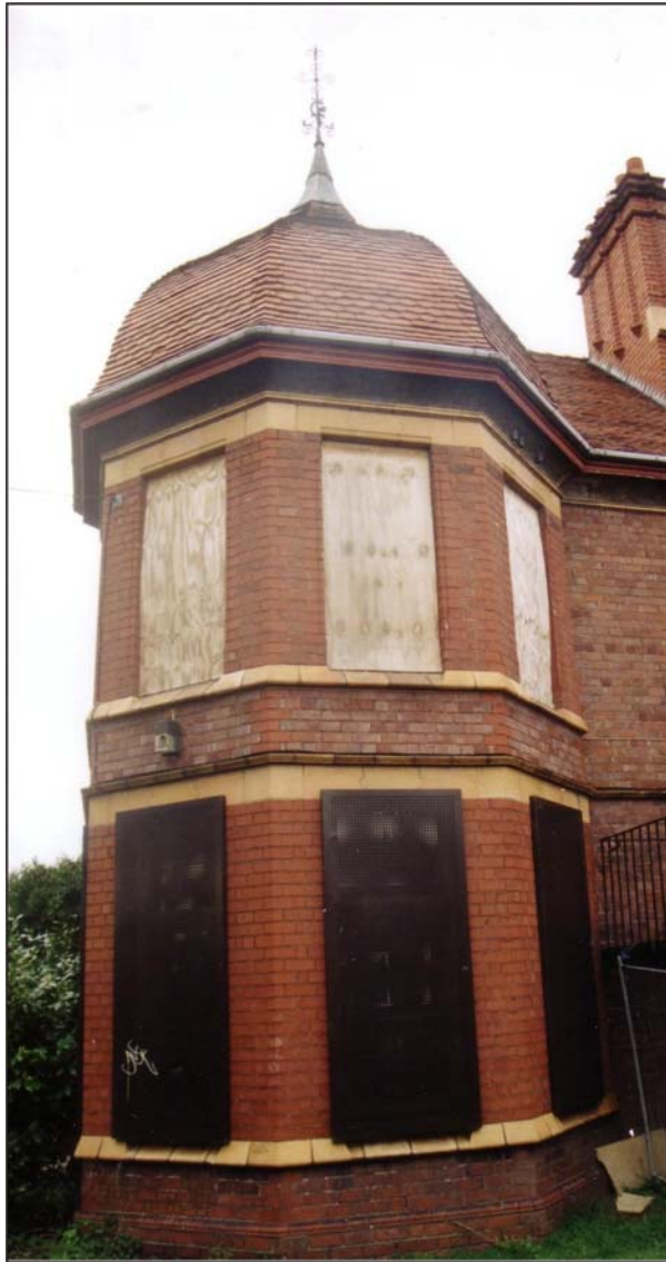
Plate 6: South-west tower from south
