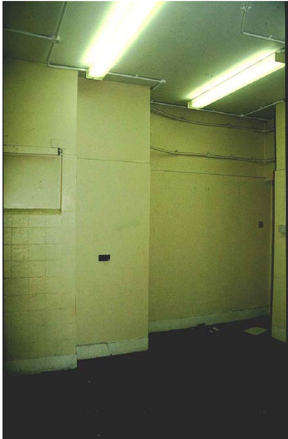
Plate 48: Room 13 showing tiling and dumb-waiter
