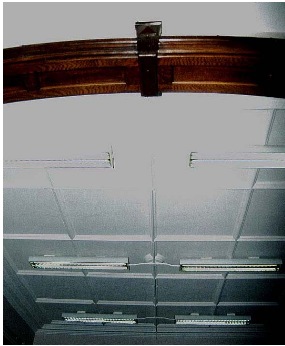
Plate 39: Coffered ceiling of Room 6
