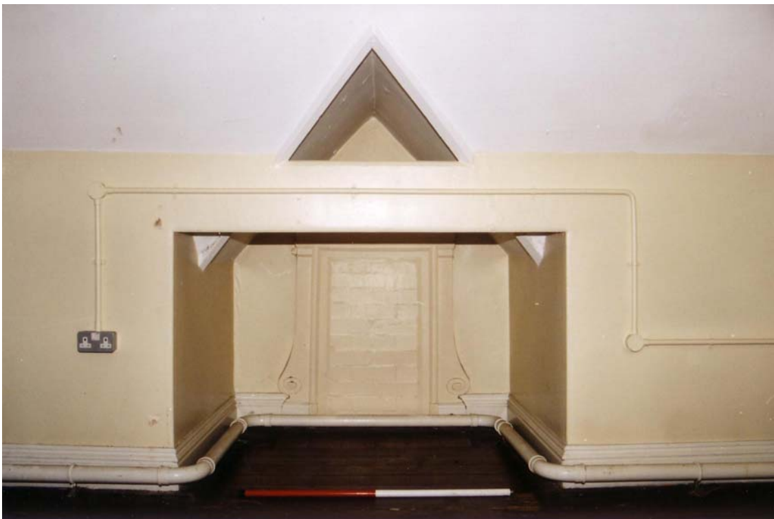
Plate 104: Fireplace in Room 44
