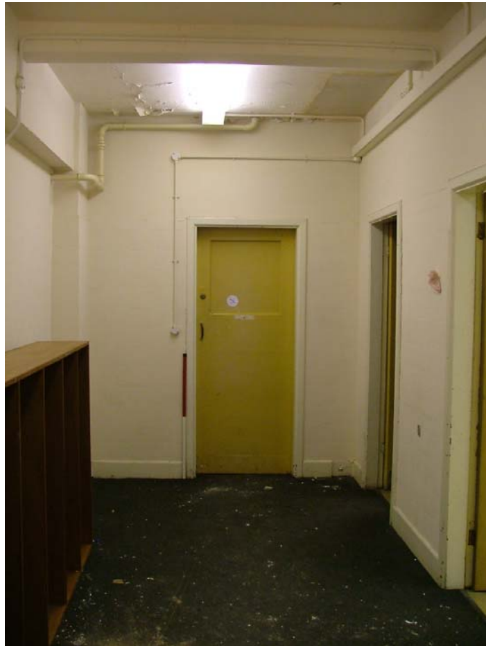
Plate 47: Room 10 from the south
