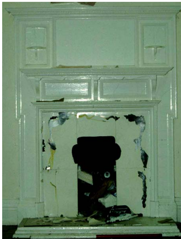
Plate 87: Fireplace in Room 37
