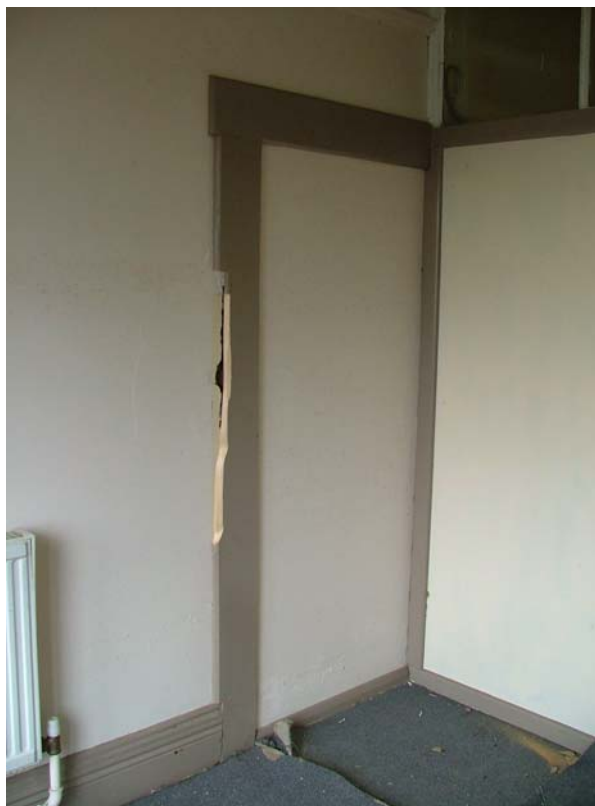
Plate 80: Blocked doorway in south-east corner of Room 34
