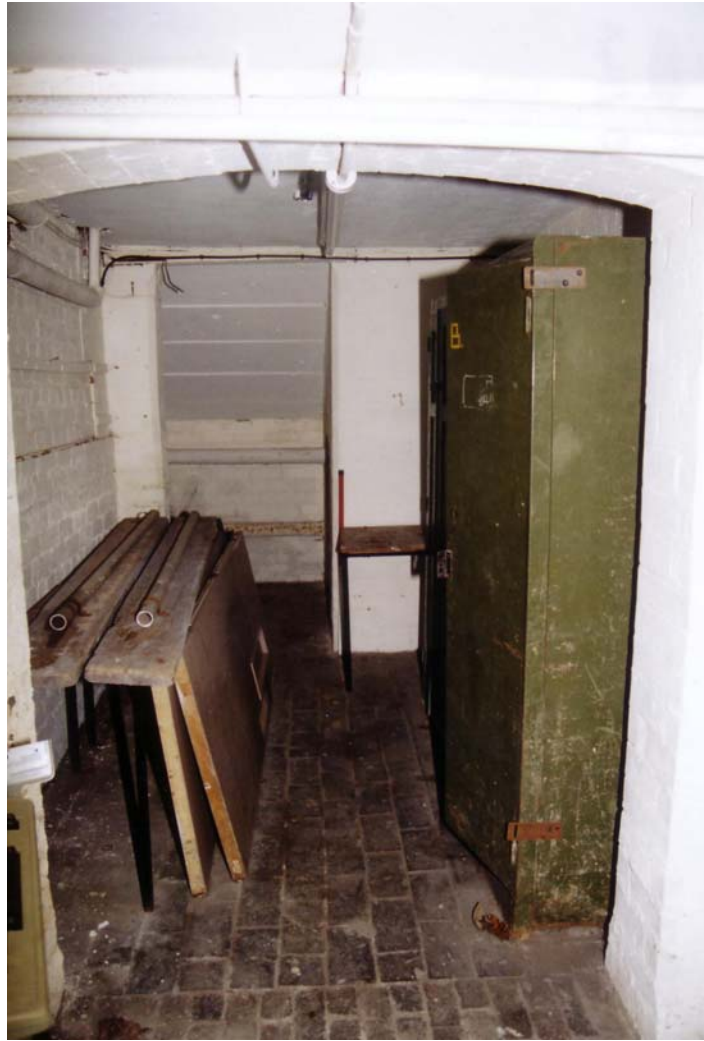
Plate 113: Room 52 looking west
