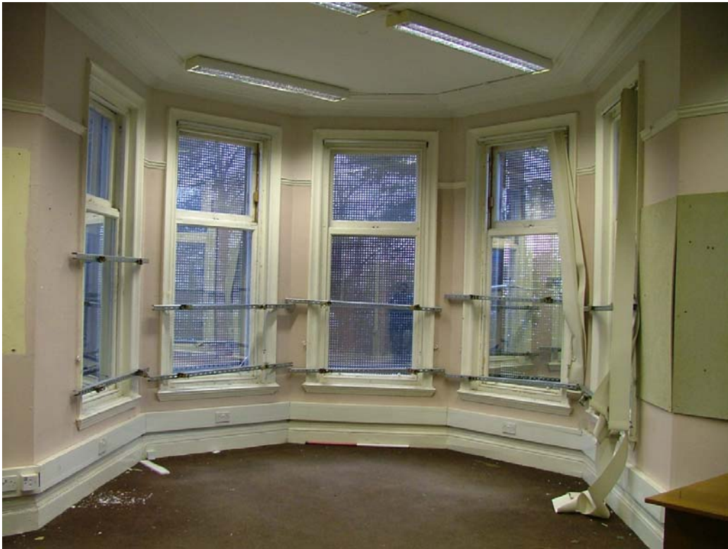
Plate 20: Bay window in south-west corner of Room 1
