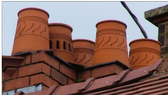
Plate 3: Example of decorated chimney pots
