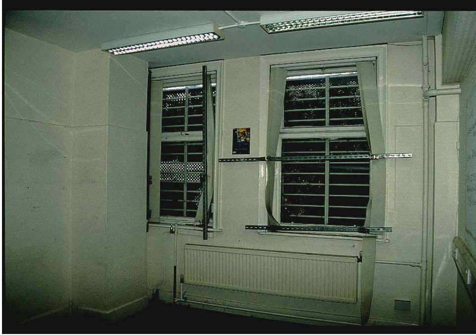
Plate 46: Room 10 from the south-east
