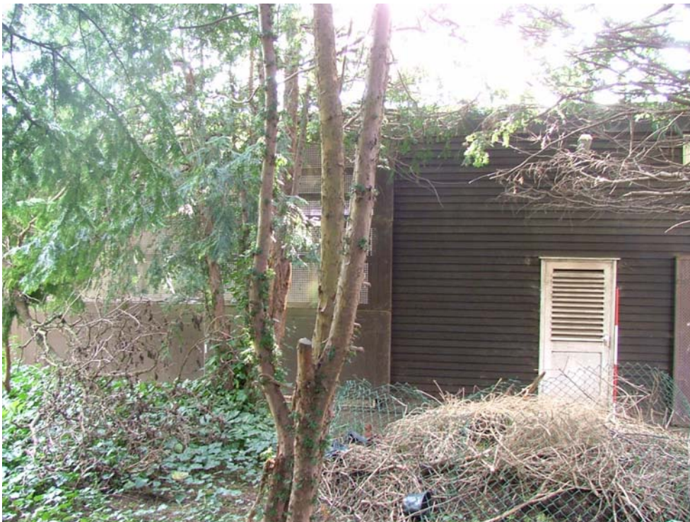
Plate 126: 20 th century extension from east
