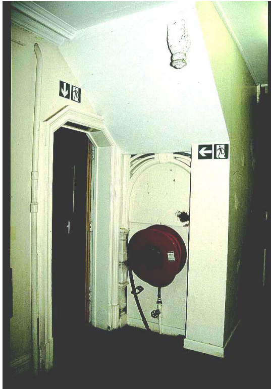
Plate 33 Blocked entrance to stairs and doorway to Room 6
