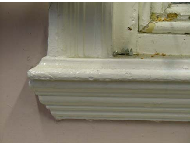
Plate 21: Detail of window mouldings
