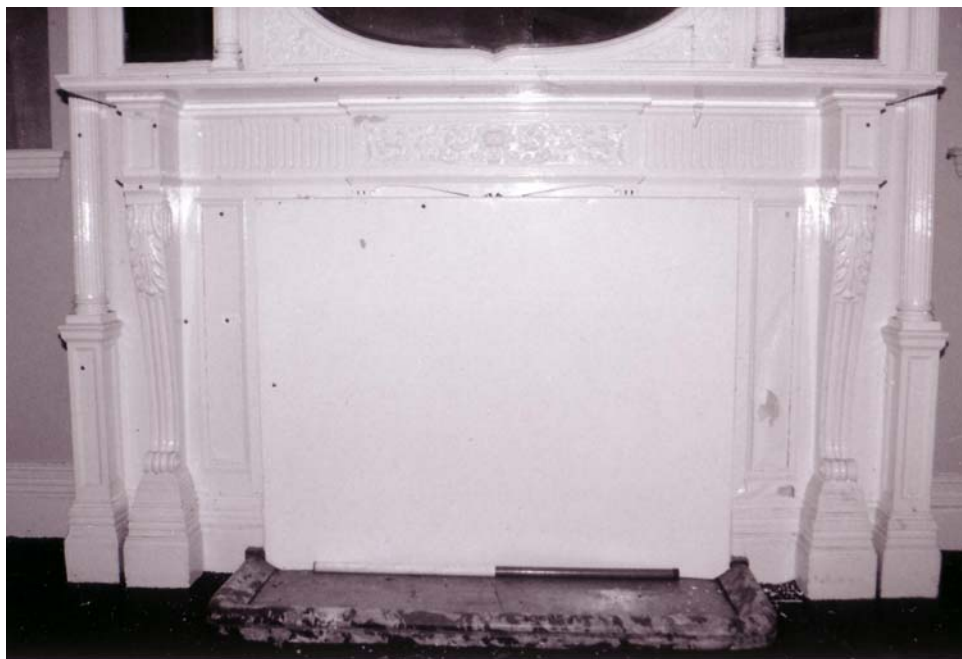
Plate 19: Fireplace in Room 1
