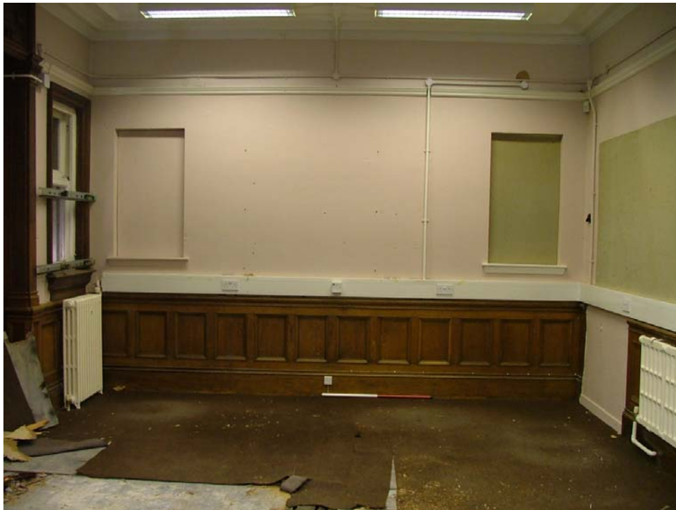
Plate 38: West end of Room 6
