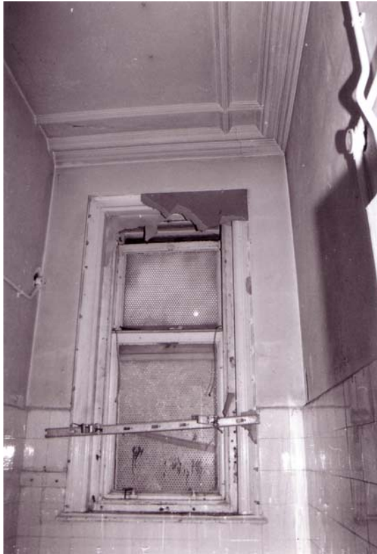
Plate 26: Room 3 looking north
