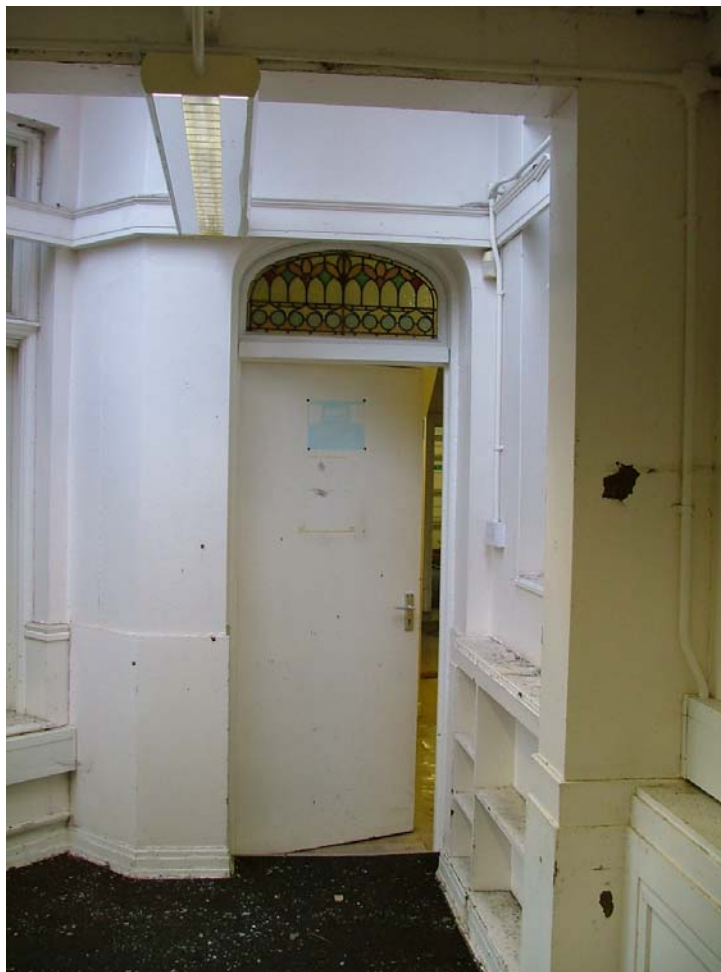
Plate 42: Second entrance to house, with decorative fanlight
