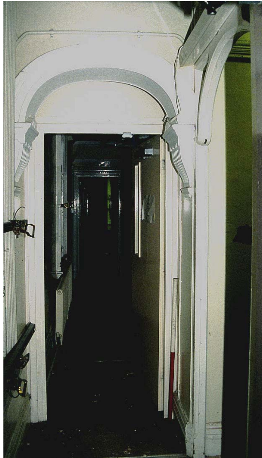
Plate 65: Corridor 23 from east, showing plaster arch
