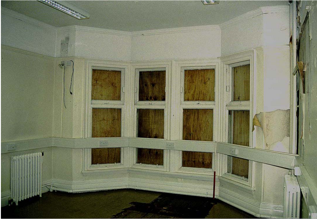
Plate 81: Bay window in west wall of Room 35
