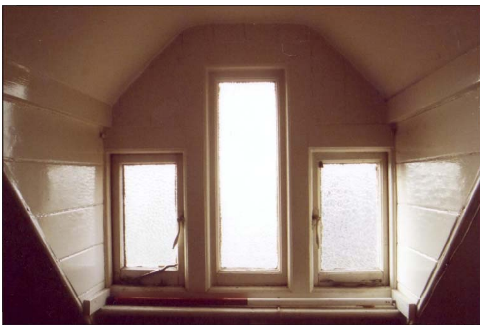
Plate 97: Window on second floor land 43a
