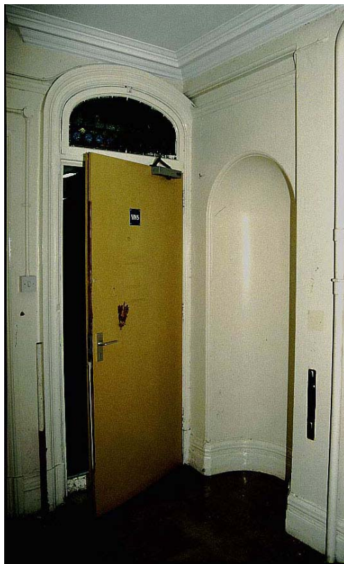
Plate 34: Second entrance and niche in corridor to east of Room 6
