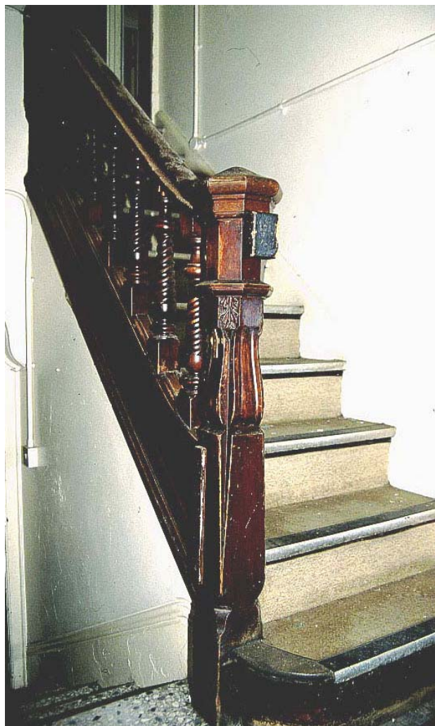
Plate 55: Staircase from half landing 19
