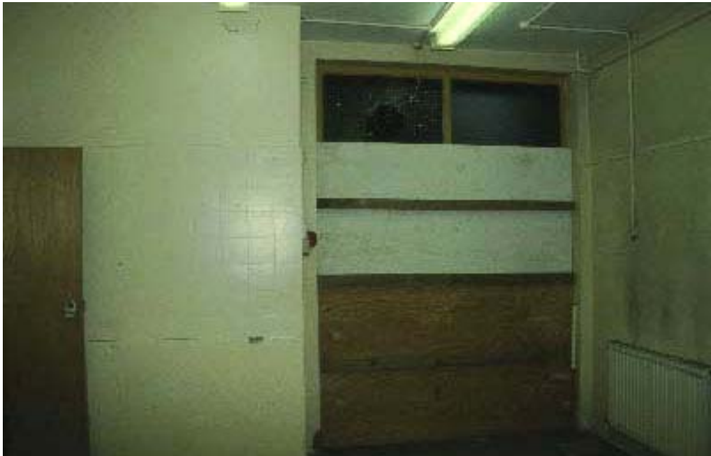
Plate 49: Room 13 looking east
