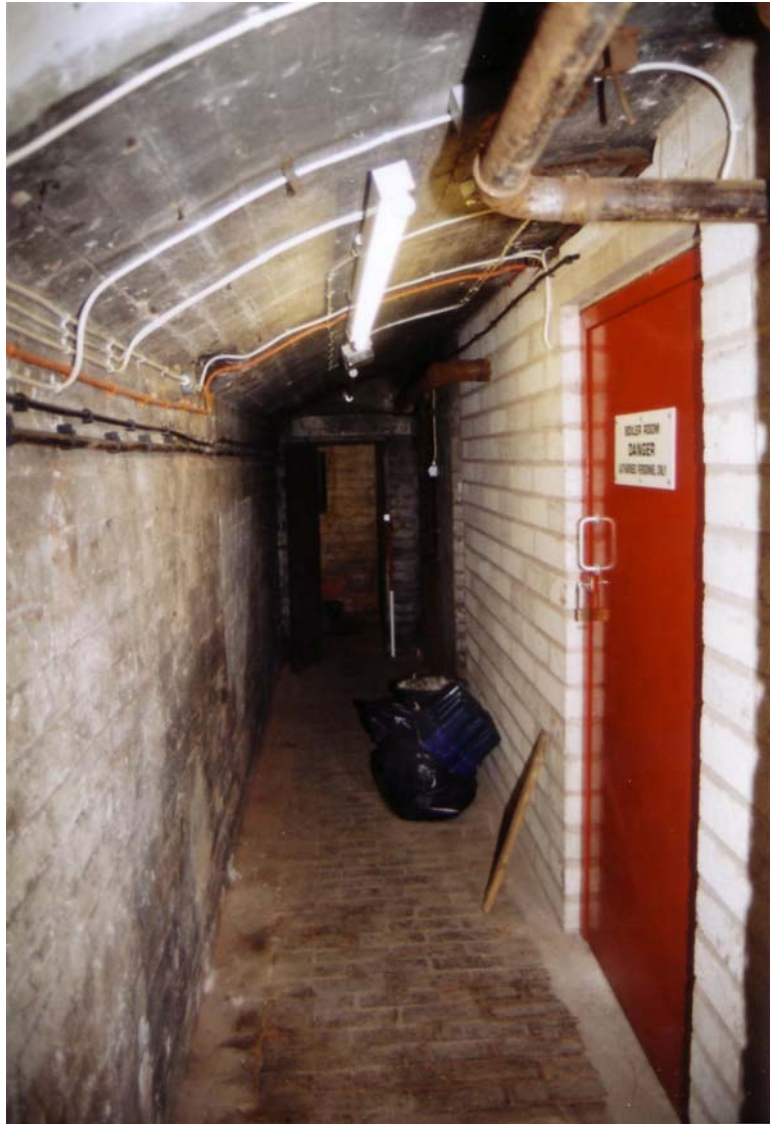
Plate 115: West end of corridor 53 looking west.
