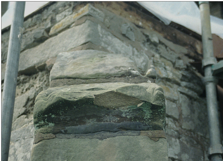
Plate 4: Capping stones of the south-est buttress showing grooves
