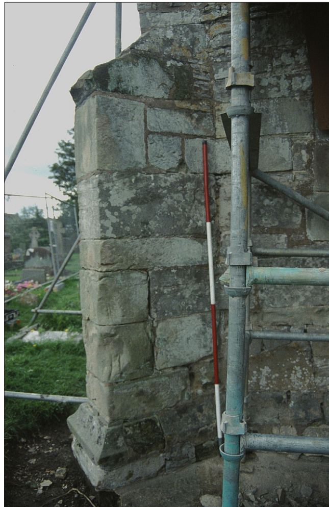
Plate 2: The south-east buttress of the south aisle from the east
