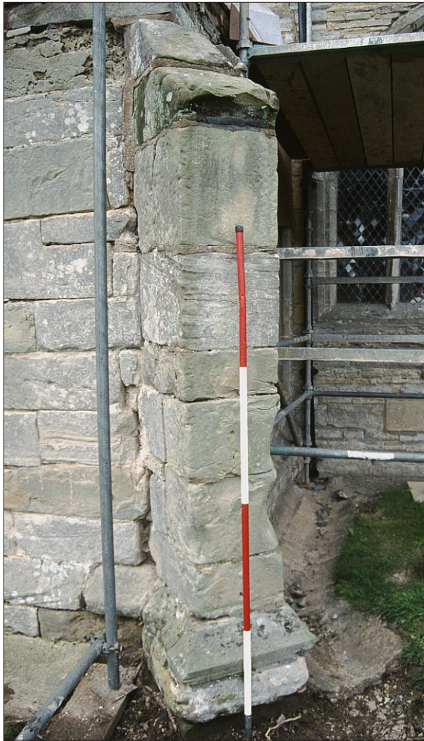
Plate 3: The south-east buttress of the south aisle from the south-east
