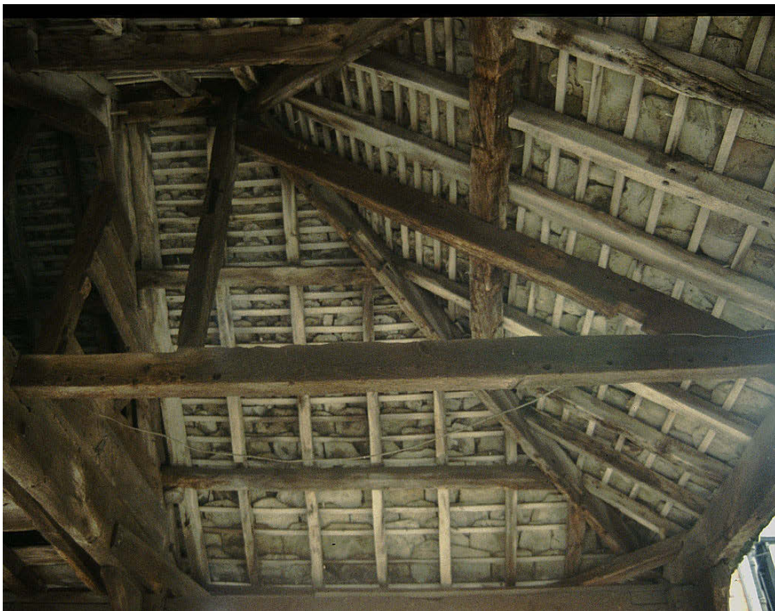
Plate 8: Half truss supporting hipped roof
