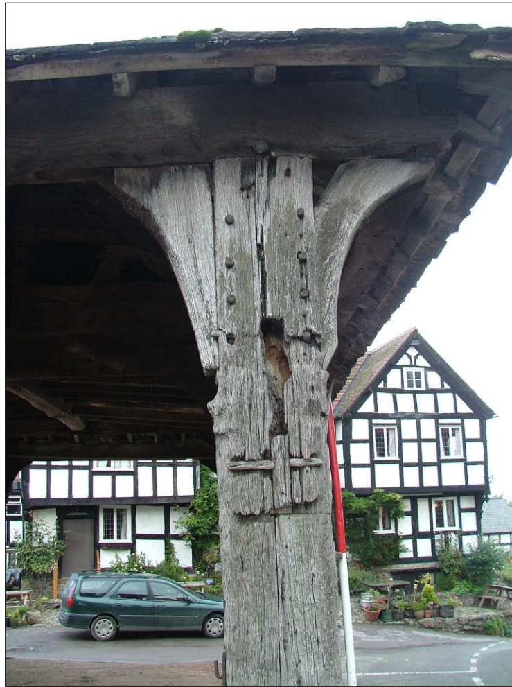
Plate 9: South-east post of market hall showing Phase I and Phase IV replacement brackets together with mortice and tenon on external face
