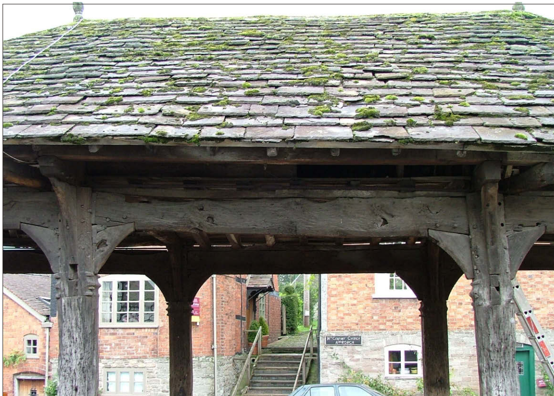
Plate 10: Remains of mortice and tenon joints in west faces of posts in the west elevation at the level of the decorative caps
