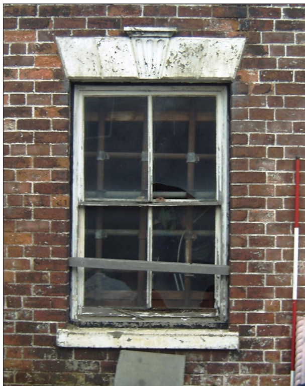
Plate 4: Ground floor sash window with rusticated stone lintel
