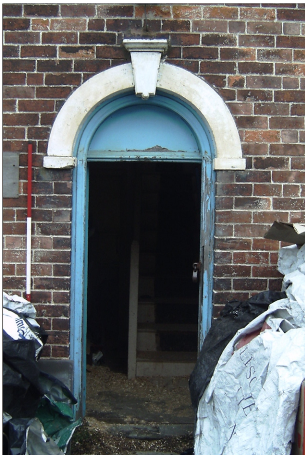
Plate 3: Doorway in south elevation of house
