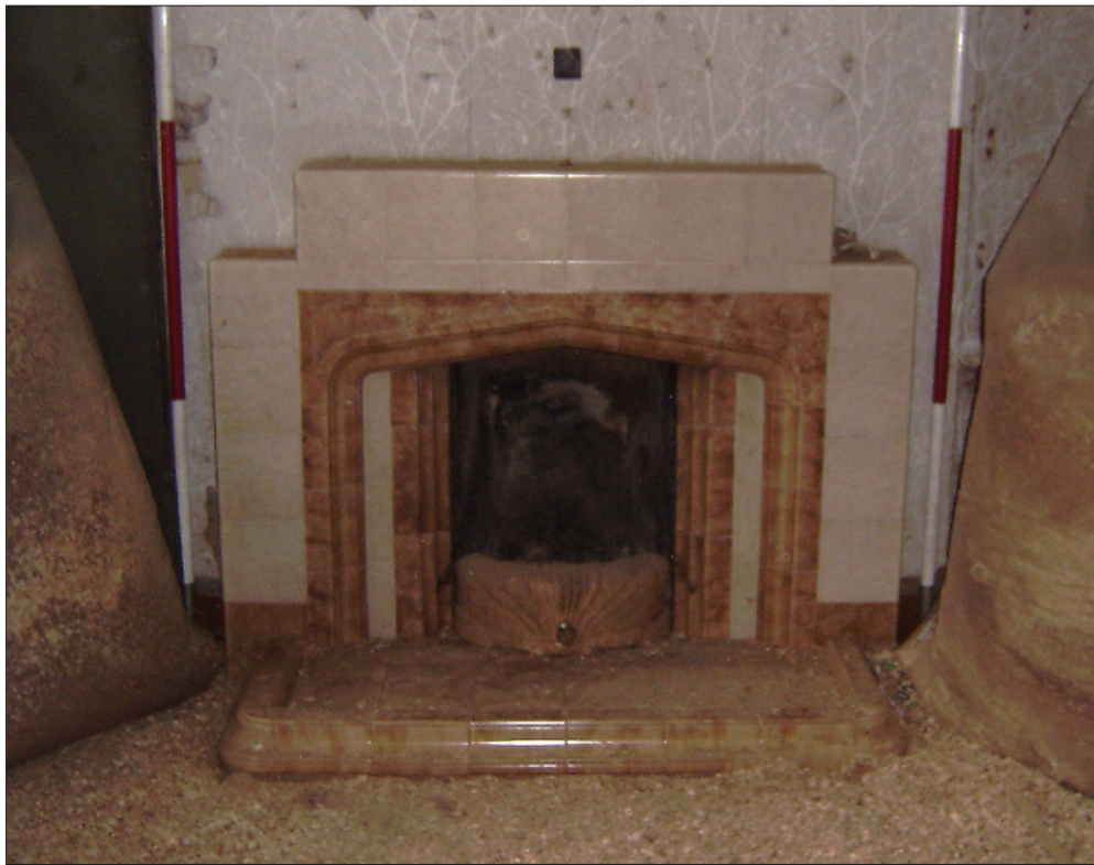
Plate 5: Fireplace in Room 3
