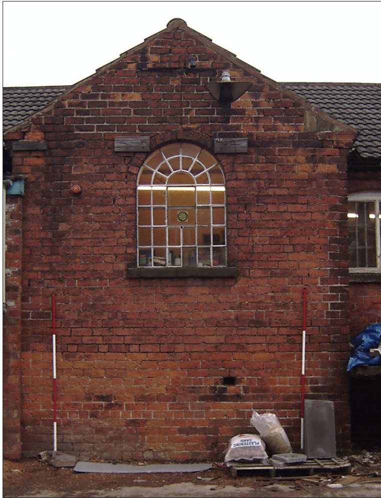
Plate 11: Extension on north-west side of building with Phase II rebuild
