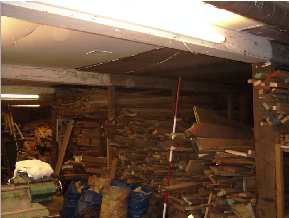
Plate 15: Basement room 13 looking north
