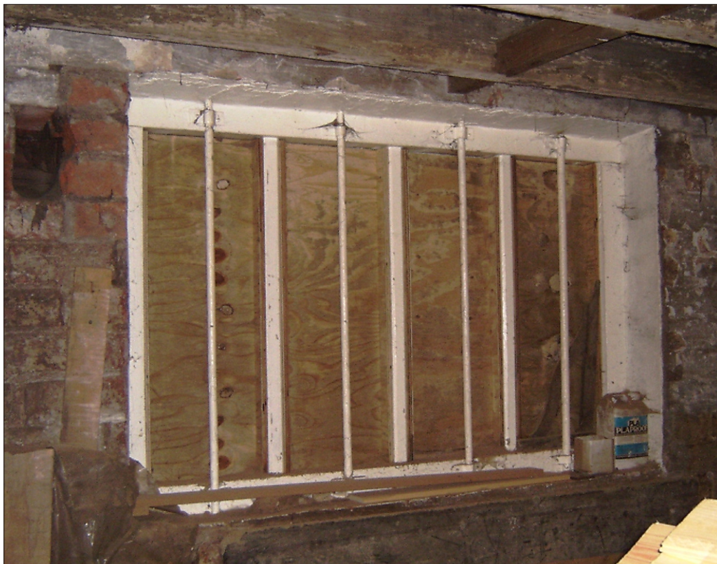
Plate 14: Phase III window lighting basement Rooms 12 & 13
