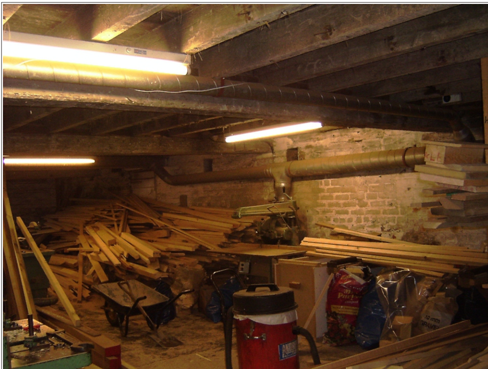
Plate 16: Basement room 14 looking north showing doorway in north-west wall
