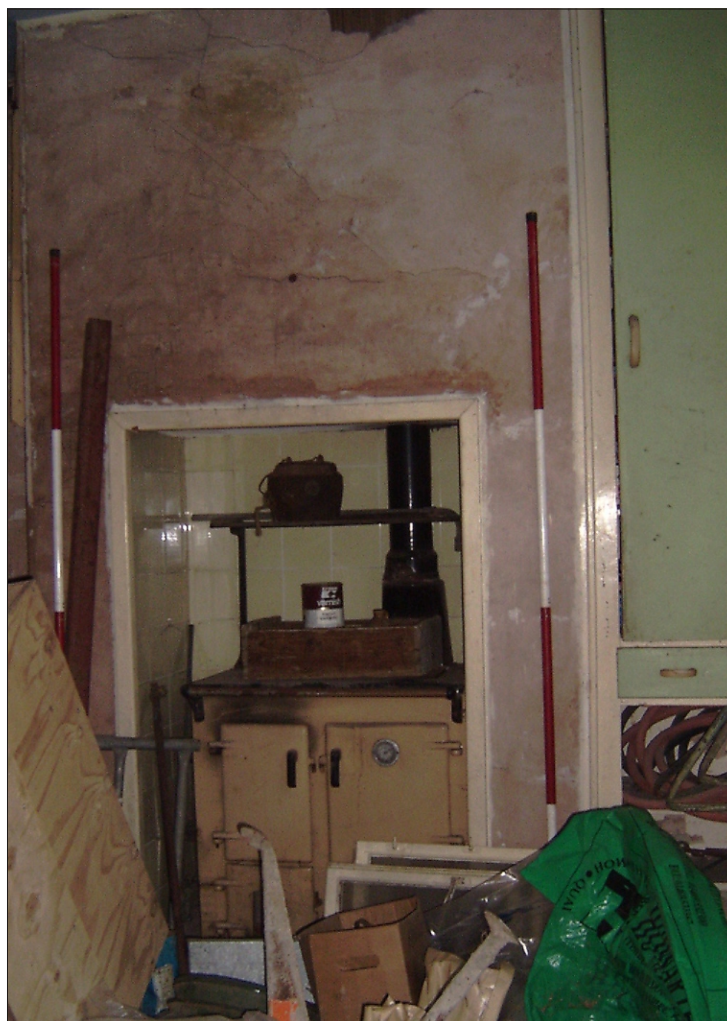
Plate 6: Fireplace and range in Room 4
