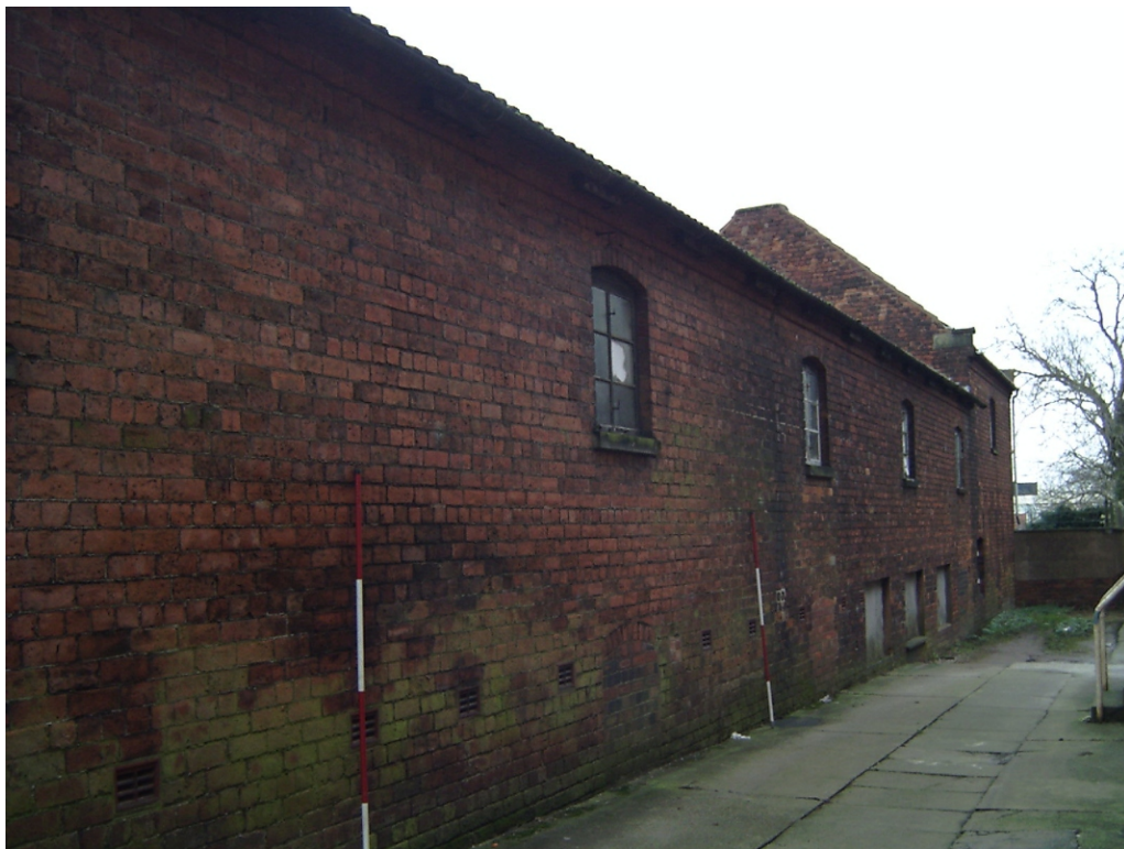
Plate 10: South-east elevation of workshop
