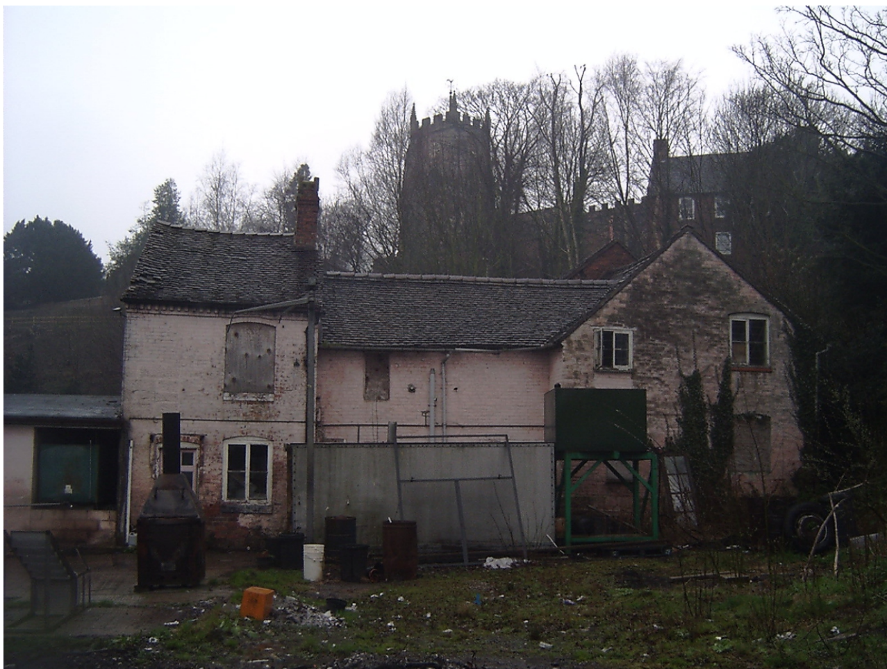
Plate 7 19th century cottage and additions at the north of the site, looking west
