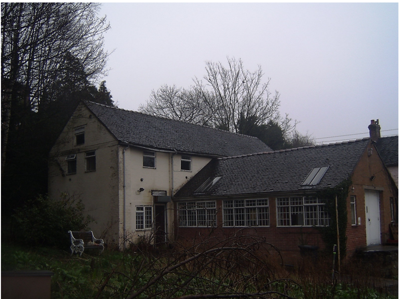
Plate 6 Whitewashed late 18th century brick building and modern extension
