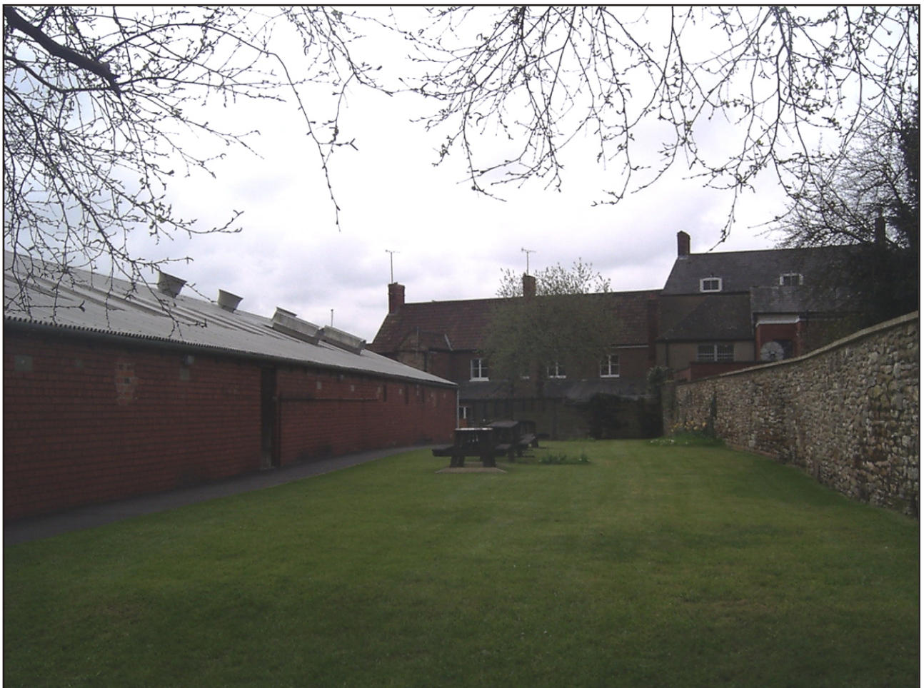
Plate 4: View of factory building looking south towards Long Street
