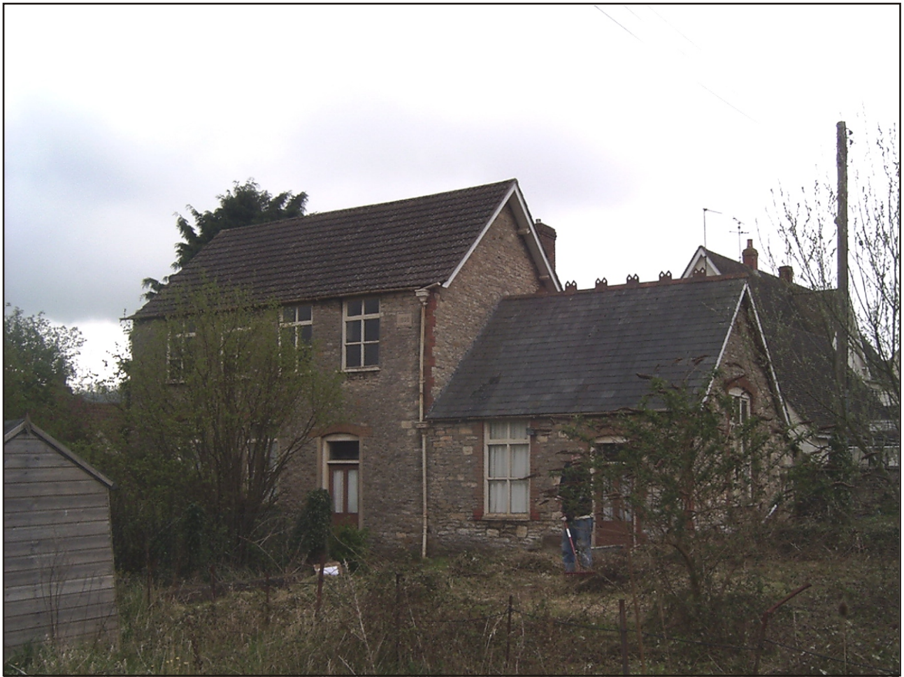
Plate 5: View of building in the far east of site looking west
