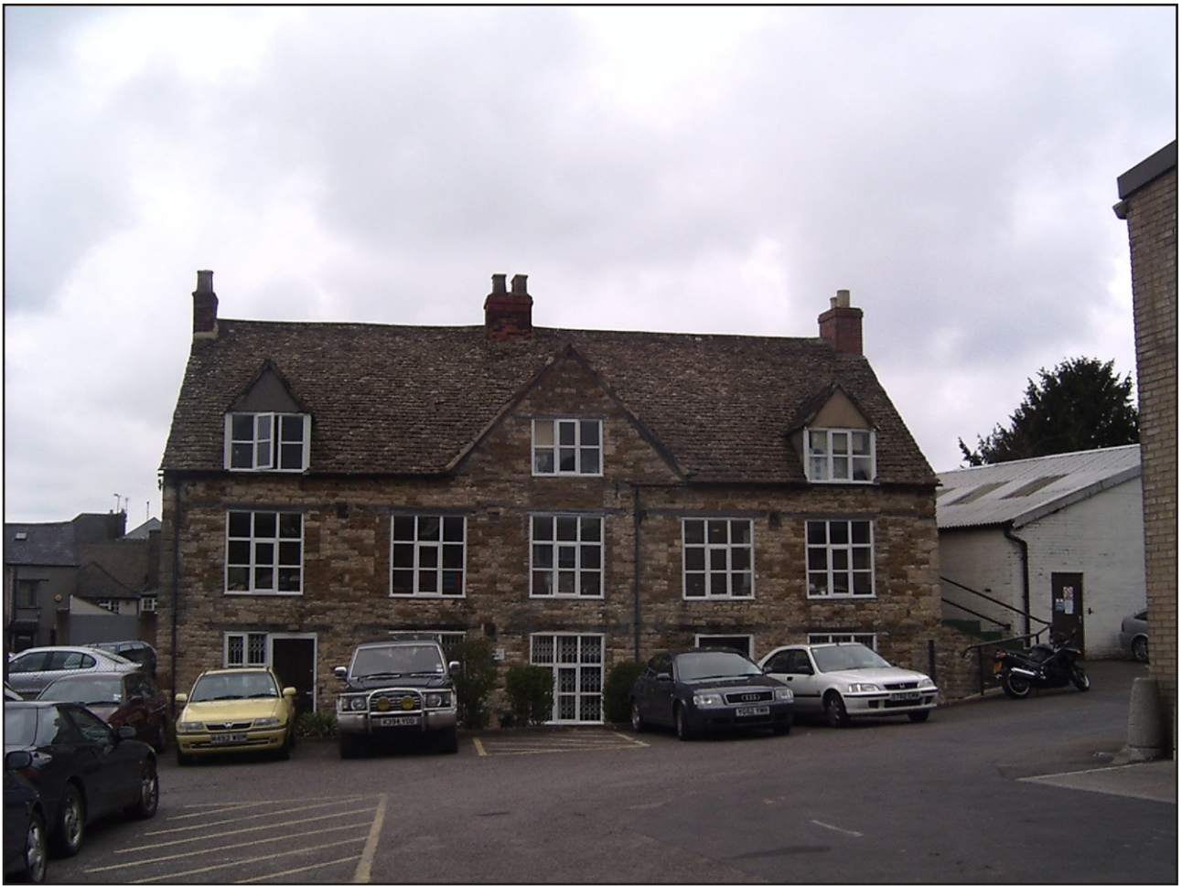
Plate 7: Listed building 19576 looking south
