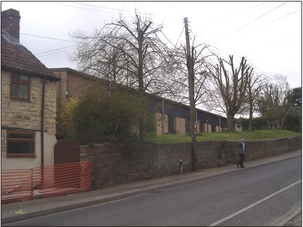
Plate 1: View of main factory building fronting on to Old Town looking south-west
