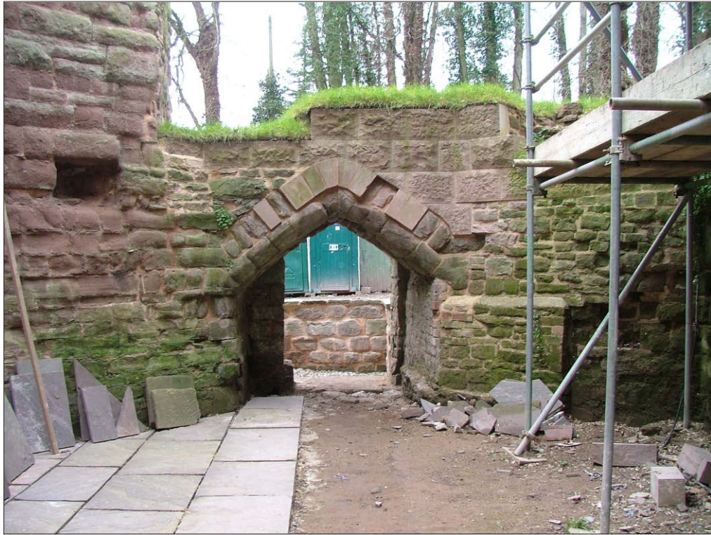
Plate 3: Door D9 at west end of tower, basement level
