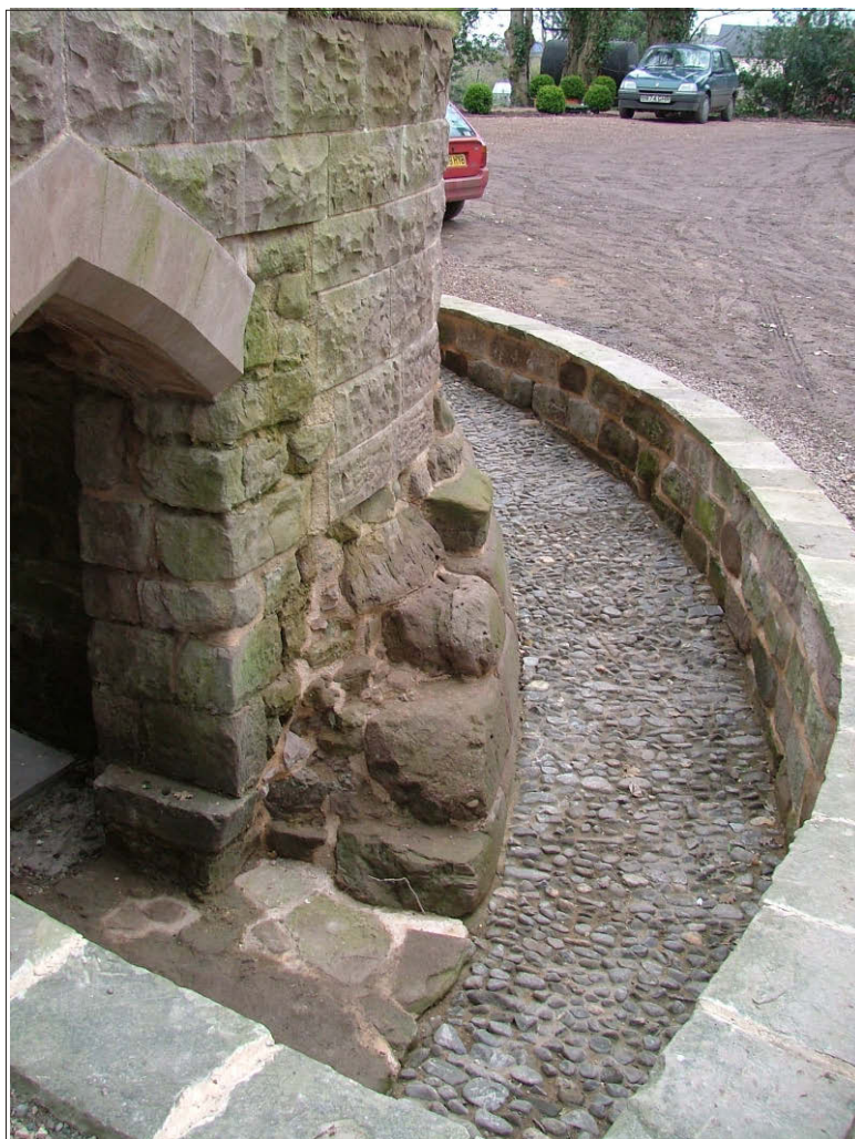
Plate 2: External battered base of tower
