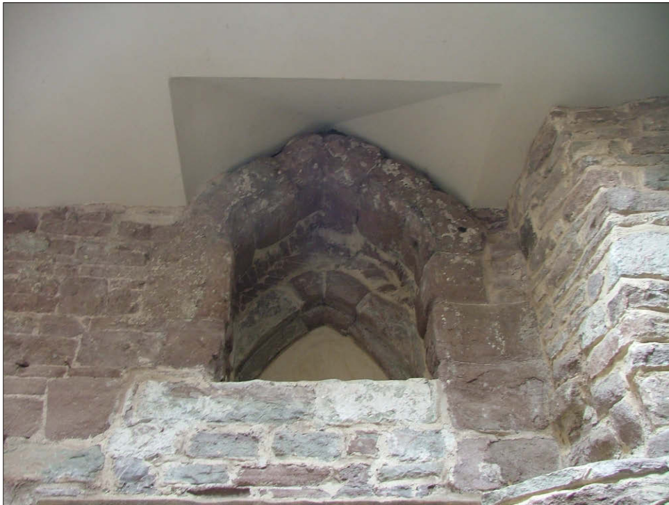
Plate 12: Door D33 between main first floor room and possible chapel room
