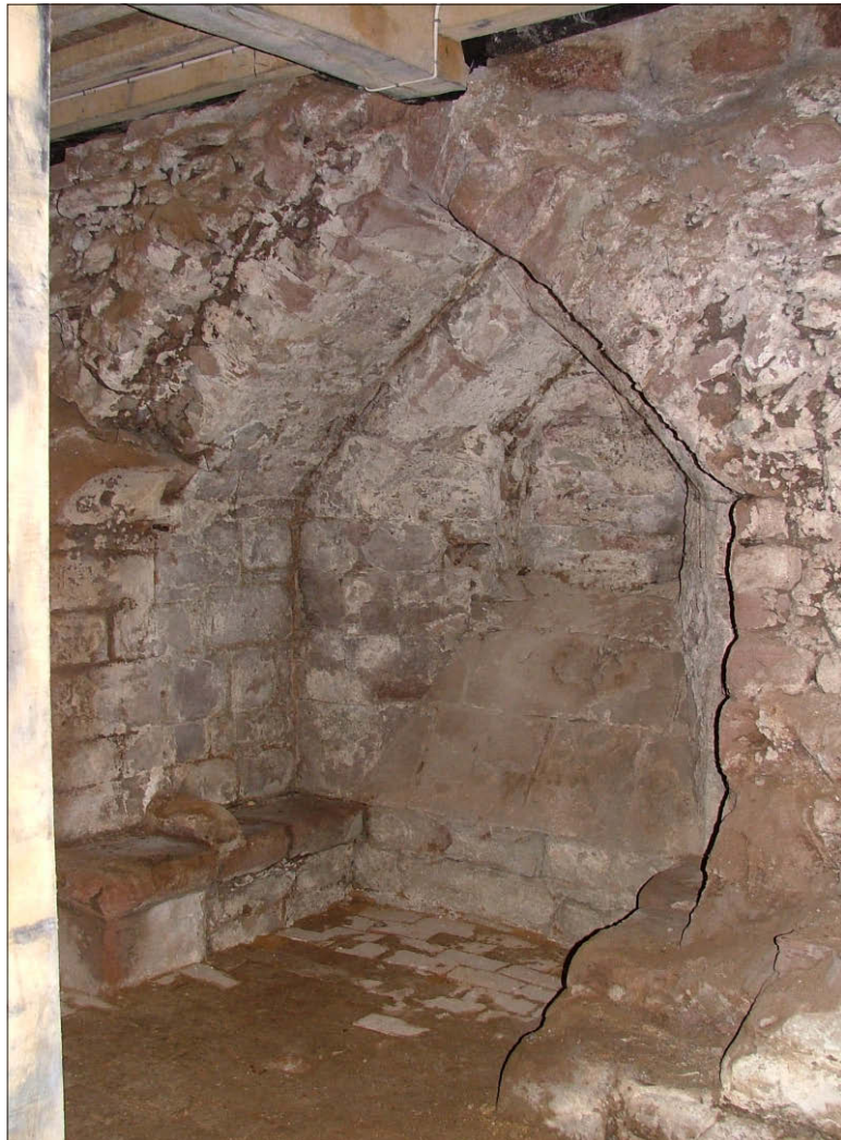
Plate 4: Window W17 in south wall of basement
