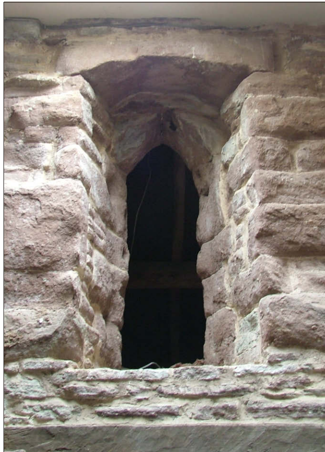
Plate 14: Window W31, one of three lighting possible chapel
