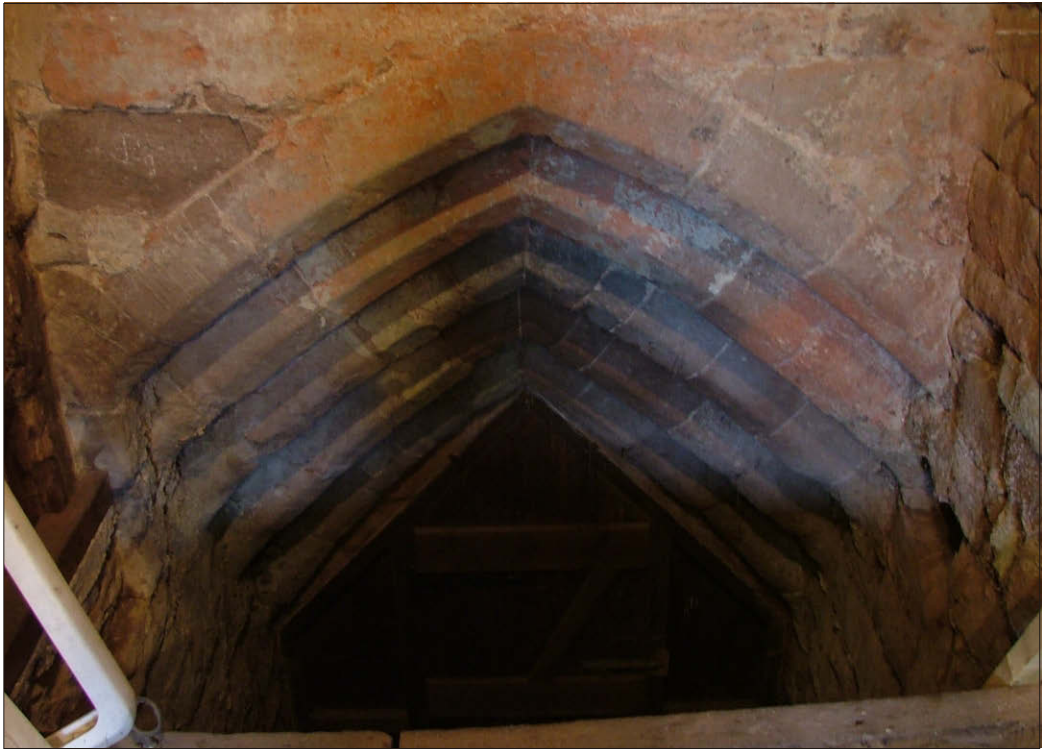
Plate 5: Door D10 from basement level
