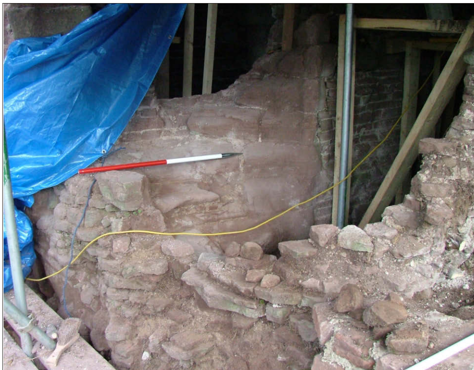
Plate 10: Spiral staircase to roof level
