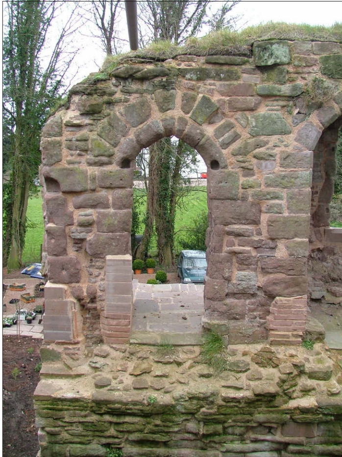
Plate 9: Door D8 leading into first floor passage to south
