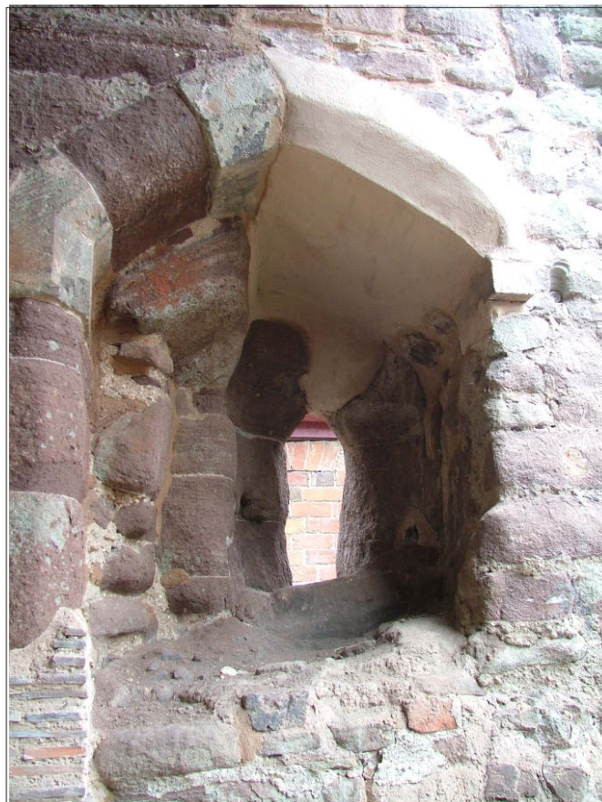
Plate 8: Arrow loop A1 in east wall of south passageway
