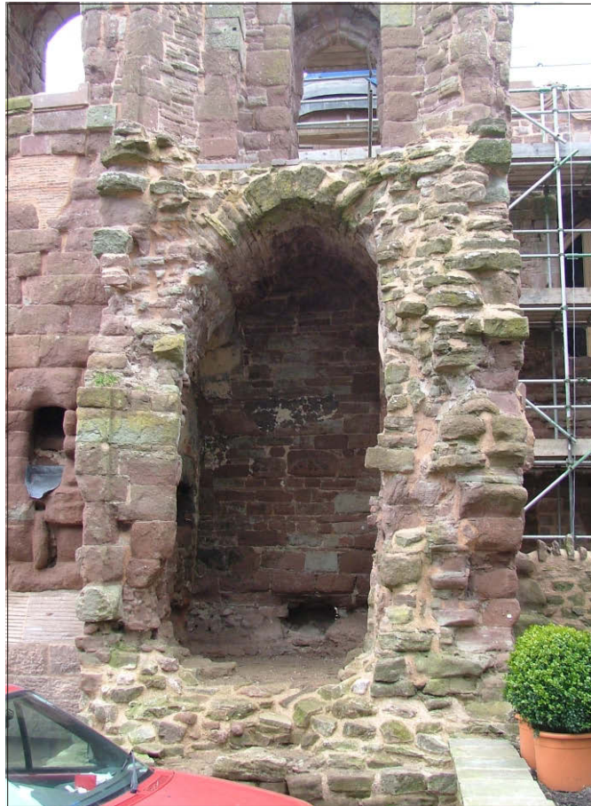
Plate 7: Passageway leading off south side of south-west tower
