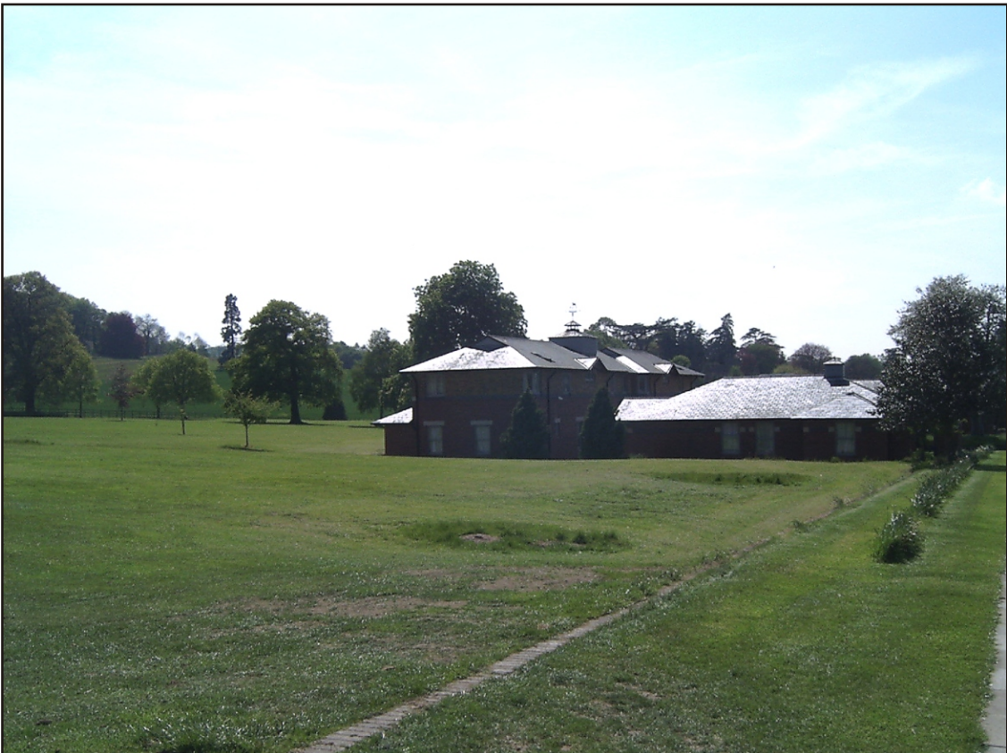
Plate 4 View of the site from the north-east
