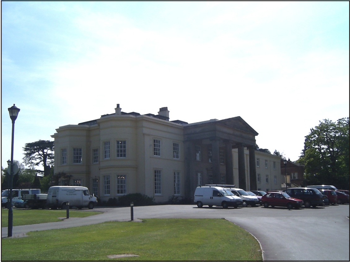
Plate 1 Acton Burnell Hall from the north-east
