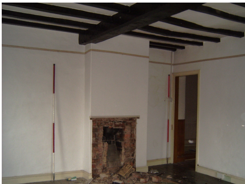
Plate 5 Interior of Well House. South-western first floor room looking north
