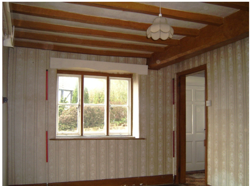
Plate 4 Interior of Well House. South-eastern ground floor room looking south
