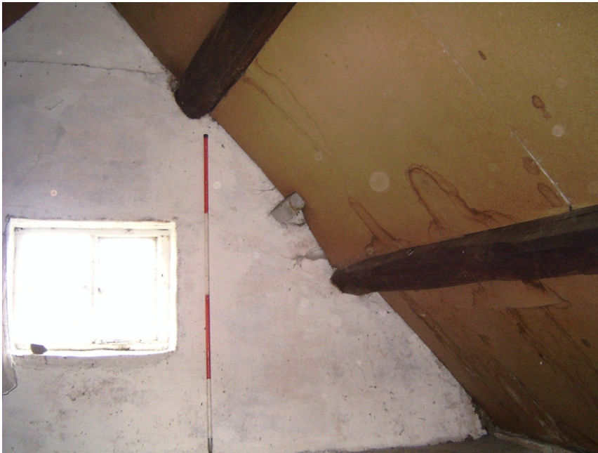
Plate 6 Interior of Well House. Internal roof space looking south-west
