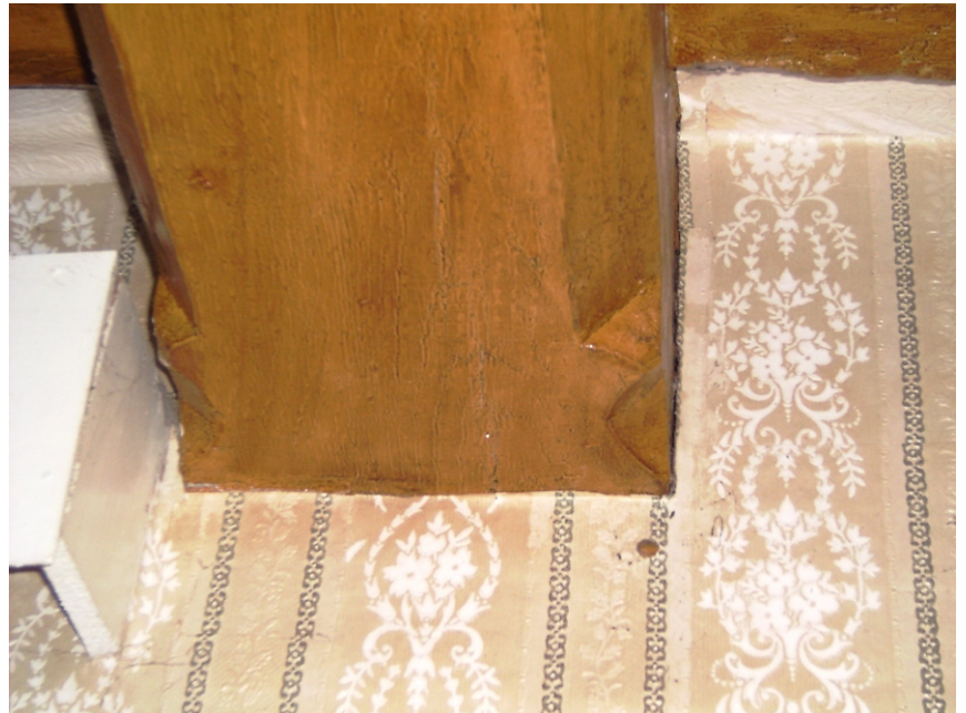
Plate 7 Interior of Well House. Ground floor, detail of chamfered beam stops
