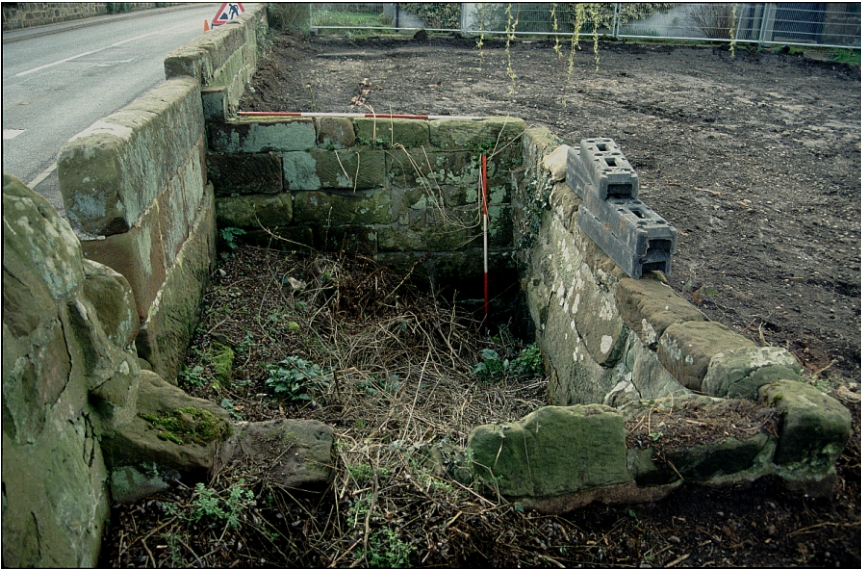
Plate 3 Well enclosure to east of Well House, looking west
