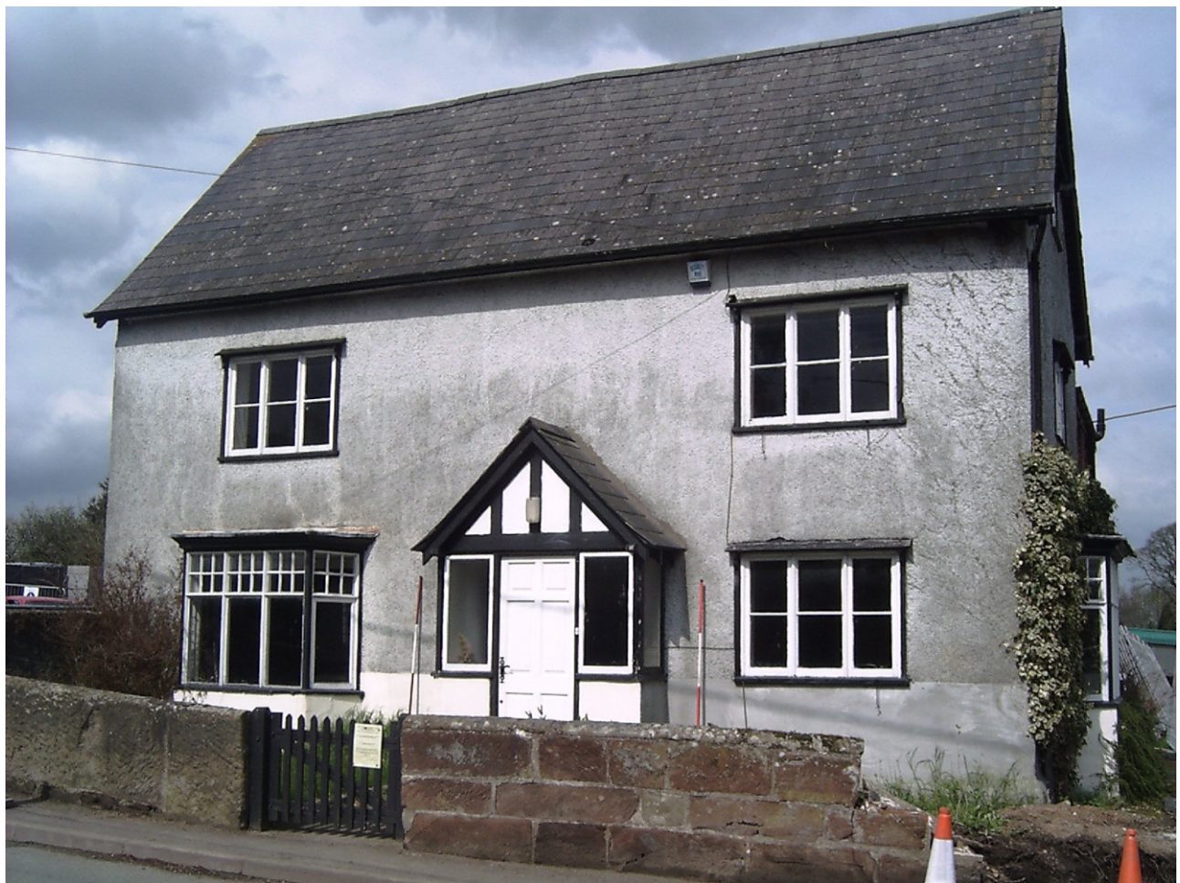
Plate 1 Well House, south elevation
