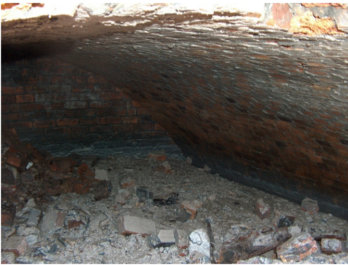
Plate 9 - tunnel structure over old canal dock
