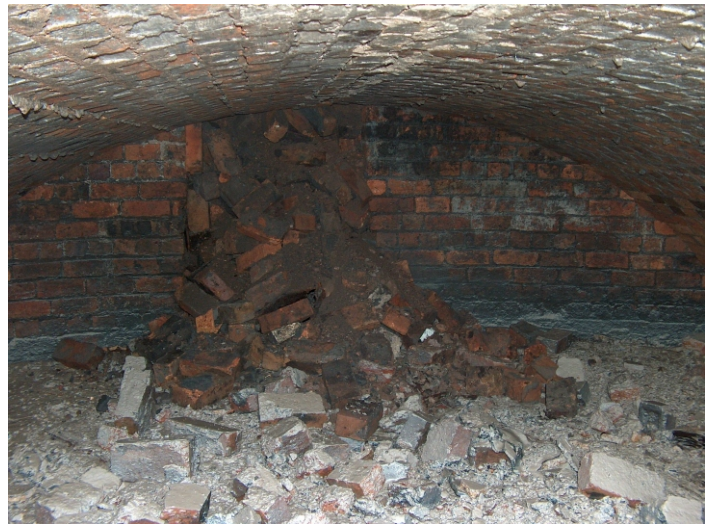
Plate 10 - tunnel over dock showing blocking wall
