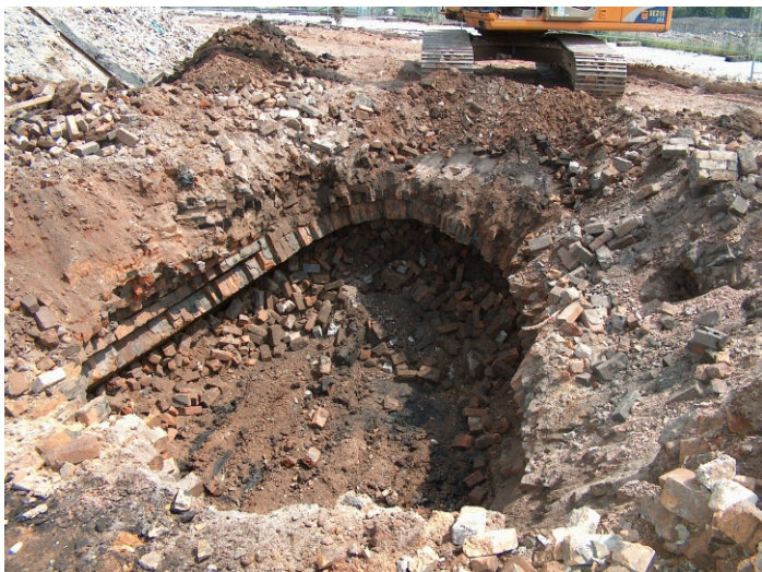
Plate 11 - tunnel over dock showing roof (canal in background)
