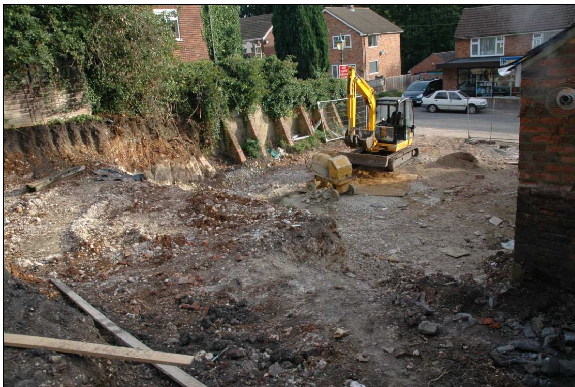
Plate 1: The northern retaining wall (looking northeast)
