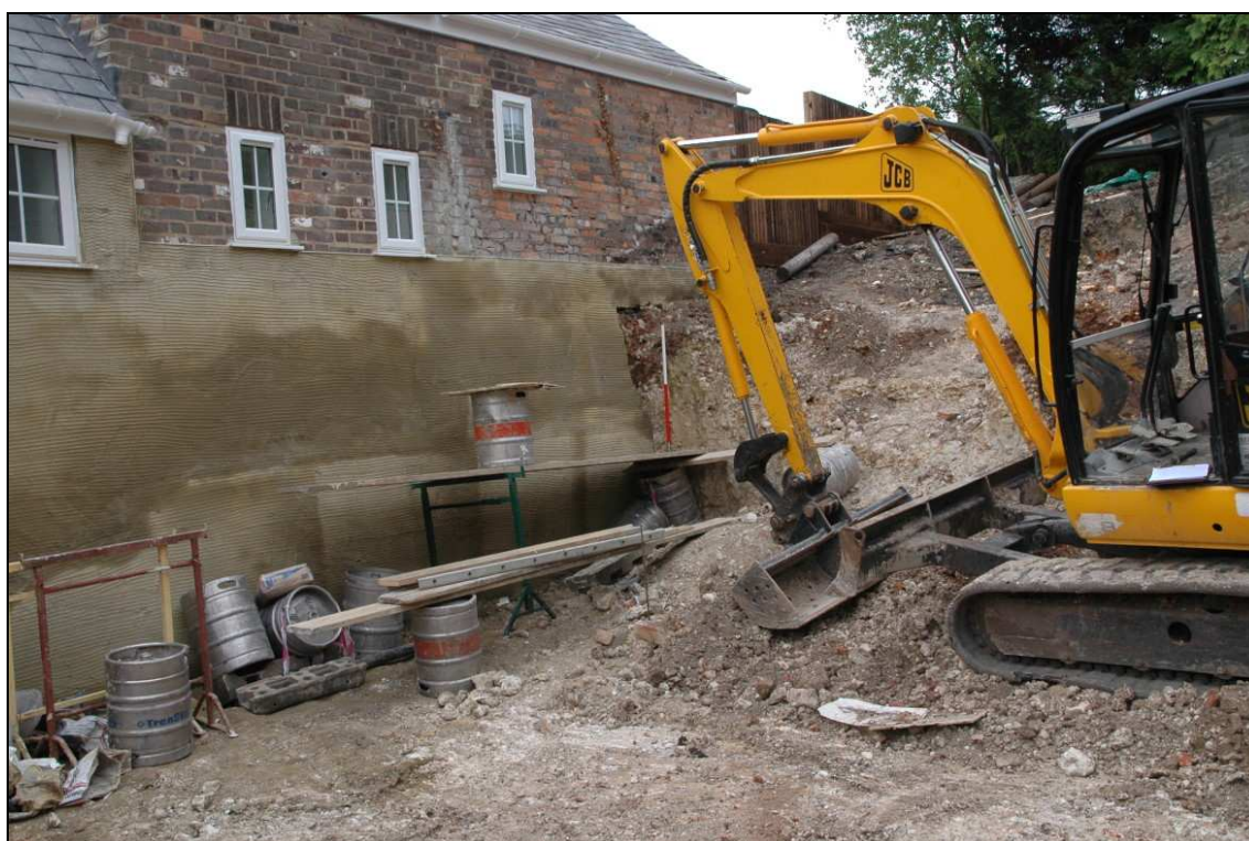
Plate 3: The building platform for the Red Lion, cut into the natural chalk (looking southwest)
