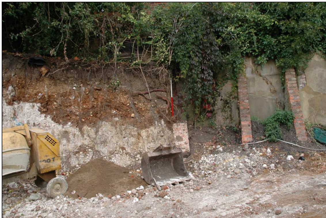
Plate 3: The natural profile of the bank behind the removed western retaining wall, and the tree root disturbance (looking north)
