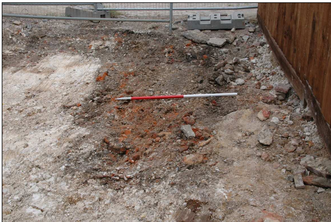
Plate 5: Fragmentary remains of Wall [001] (looking east)
