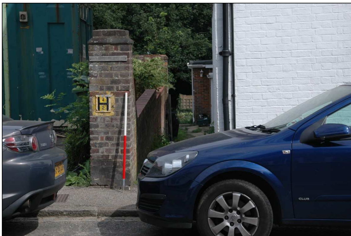
Plate 11: Natural land profile and retaining wall to the south of the car park (looking east)
