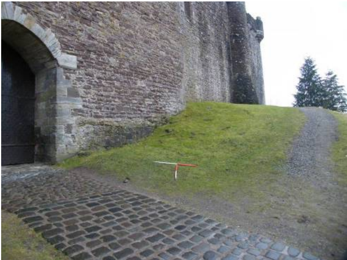
Plate 1: Pre excavation of the area of trench 1 and 2.
