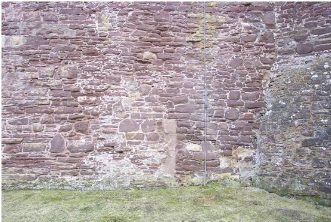
Plate 15: The early postern (right – to the left of the lightning rod) with the rough facing stones (centre)
