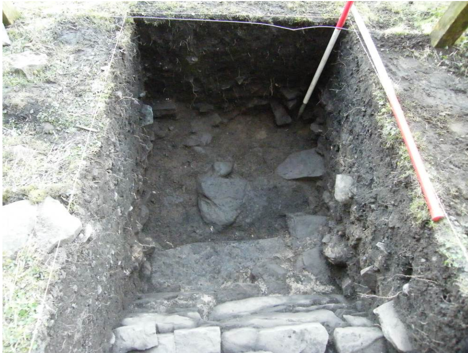
Plate 14: Mid-ex view showing foundations cut [506] running NNW/SSE (north is to the left of the picture)
