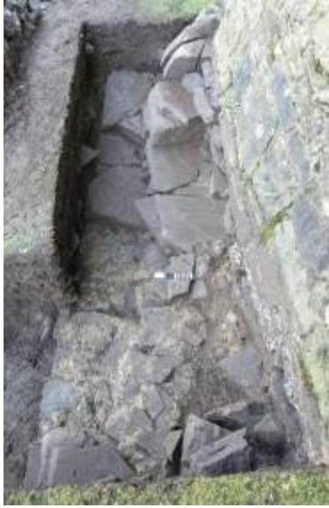
Plate 3: Footings (104) projecting from the existing north wall
