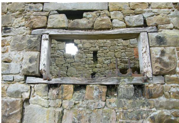
Figure 7 In situ axle housing, exterior of west wall
