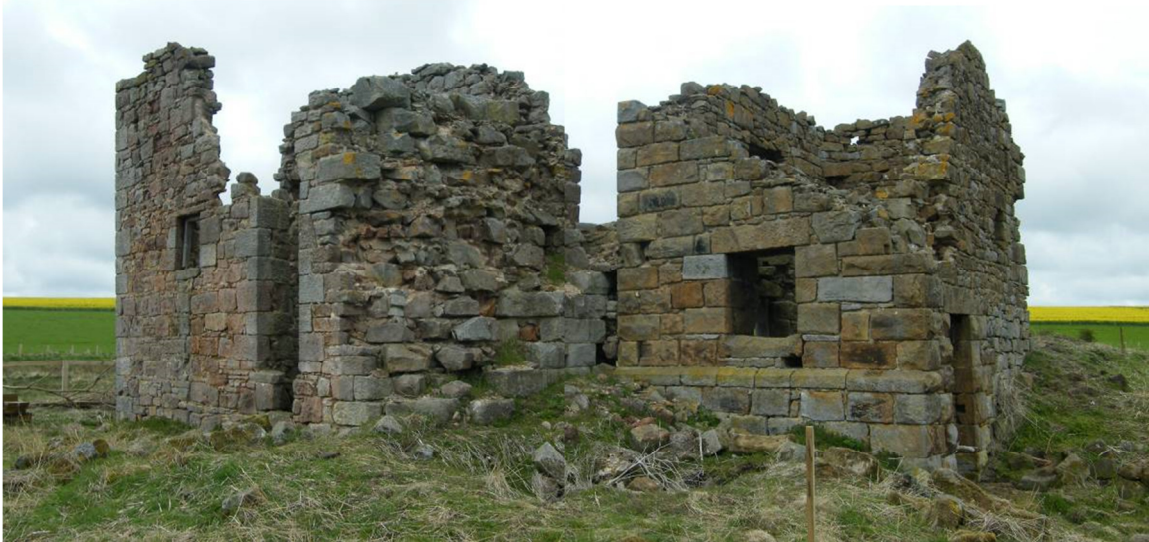
Figure 2 The two engine houses with the rubble-clogged pit head between, looking NW
