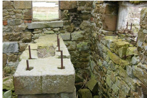
Figure 7 In situ axle housing, exterior of west wall
