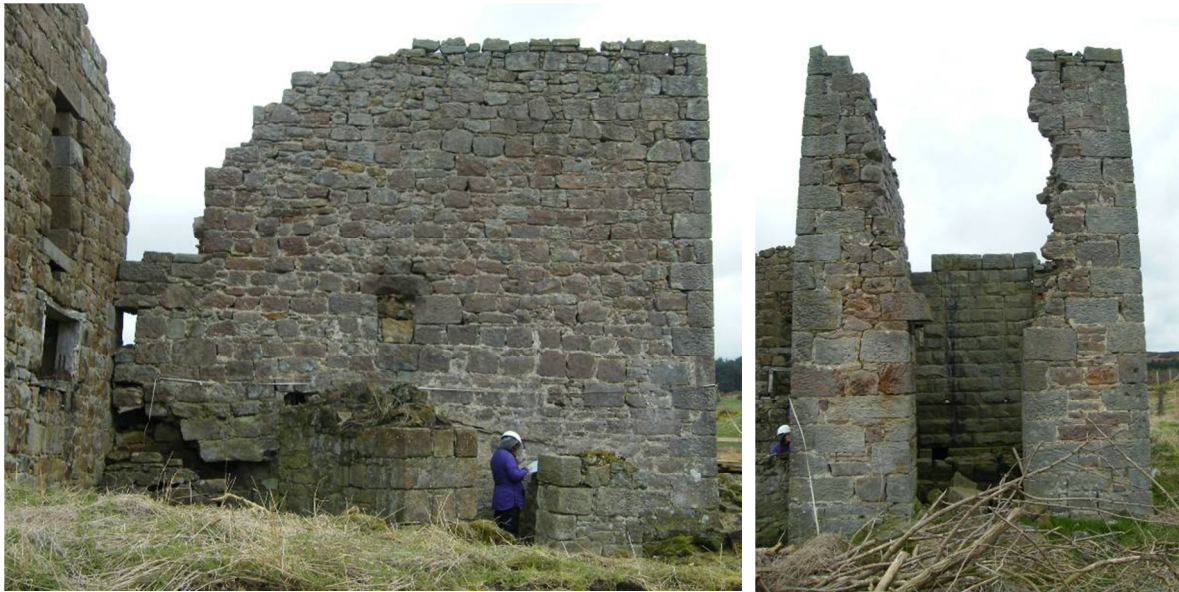
Figure 16 Engine House 2 north elevation
